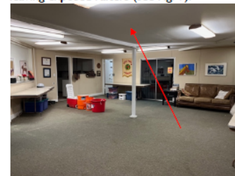
Figure 9: Remove ceiling drywall
