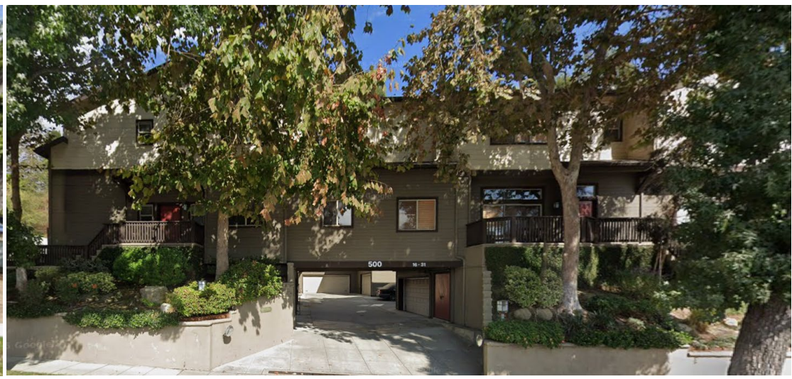
500 N. Rosemead Blvd. (multi-family, adjacent to south)
