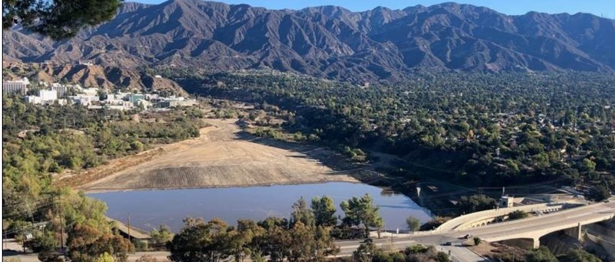
Figure 4-3: Devils Gate Dam
