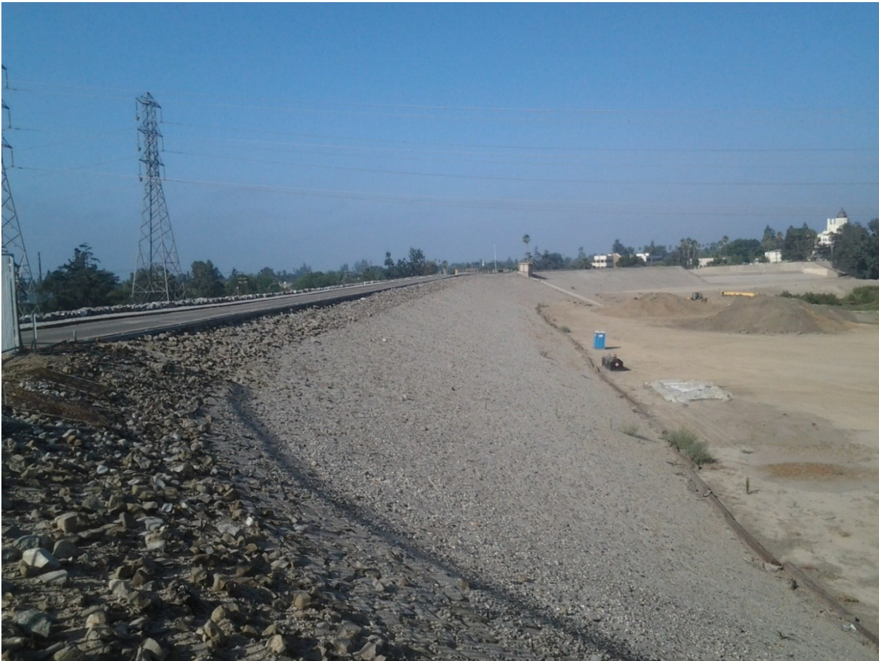
Figure 4.5: Eaton Wash Dam
