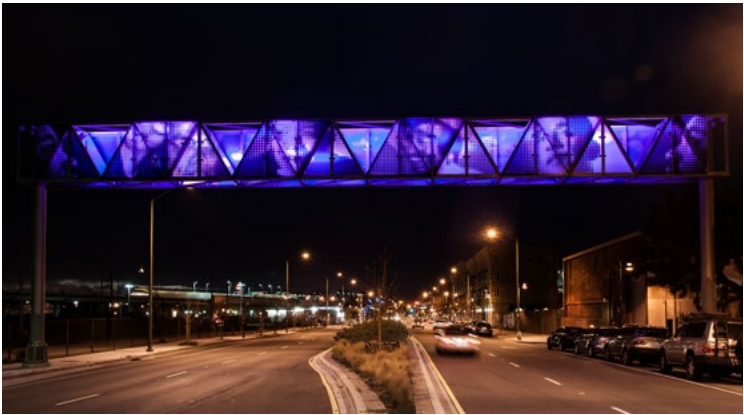
7TH STREET GATEWAY, OAKLAND, CA
