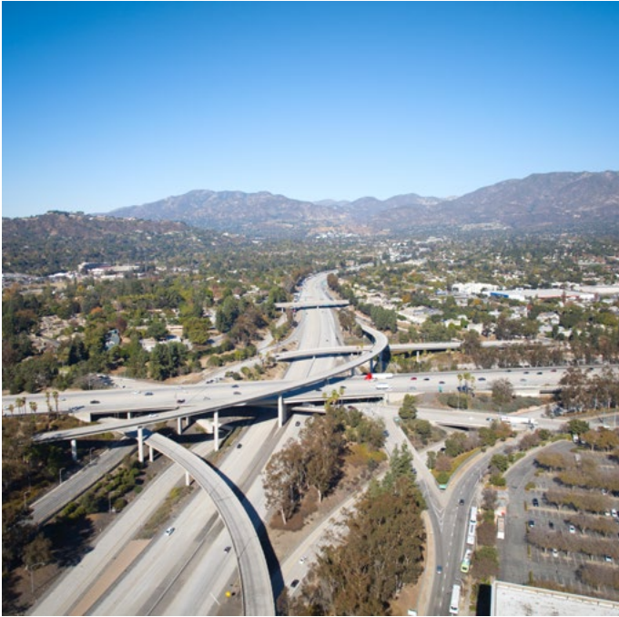
AS SEEN LOOKING TO THE NORTH SHOWING THE 710 APPROACH TO THE 210 INCLUDING THE CORSON STREET FRONTAGE ROAD AND 134 CONNECTION
