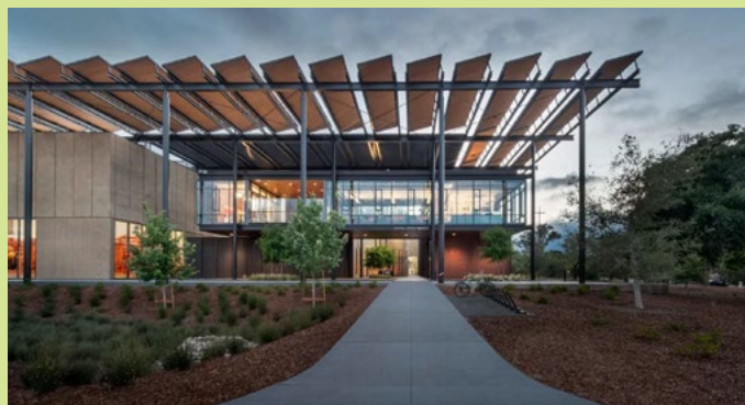
STANFORD UNIVERSITY CENTRAL UTILITY PLANT (2015) SOURCE: HTTPS://SESI.STANFORD.EDU/ENERGY-SYSTEMS/CENTRAL-ENERGY-FACILITY
