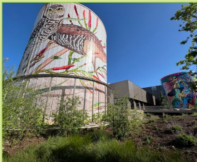
GOOGLE'S MOFFETT PARK CAMPUS. TOP: CONCEPT MASSING; BOTTOM: PHOTO OF THE BUILT CONDITIONS. SOURCE: WEST8.
