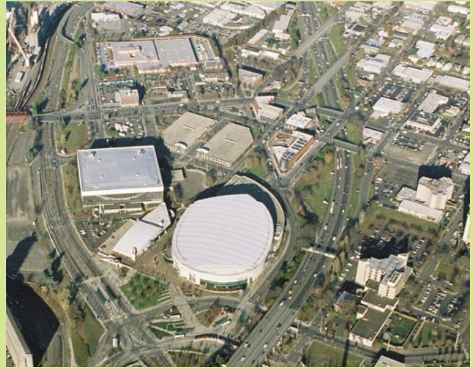
SOURCE: CITY OF PORTLAND.- LOWER ALBINA TODAY
