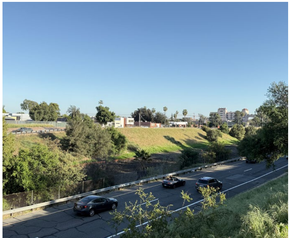
BOTTOM: EXISTING CONDITIONS OF THE "DITCH" AS SEEN FROM HAVENDALE DRIVE LOOKING SOUTH.
