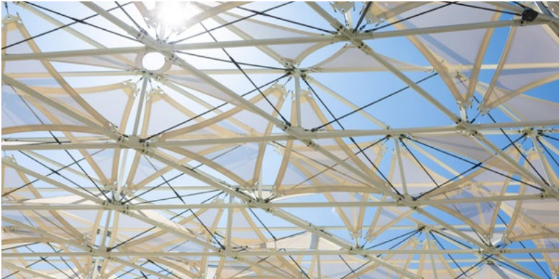
SHADE STRUCTURE AT INTUIT DOME, CLIPPERS ARENA, INGLEWOOD, CA
