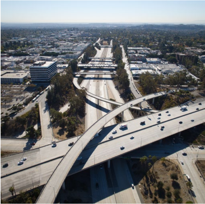
AS SEEN LOOKING TO THE SOUTH SHOWING THE MAPLE STREET FLYOVER, AND A SEQUENCE OF CONNECTING BRIDGES OVER THE 710 PROJECT AREA
