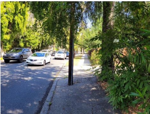
Photo 3 Caltrans signage extends into path of travel along asphalt sidewalk, shown here on Pasadena Avenue.
