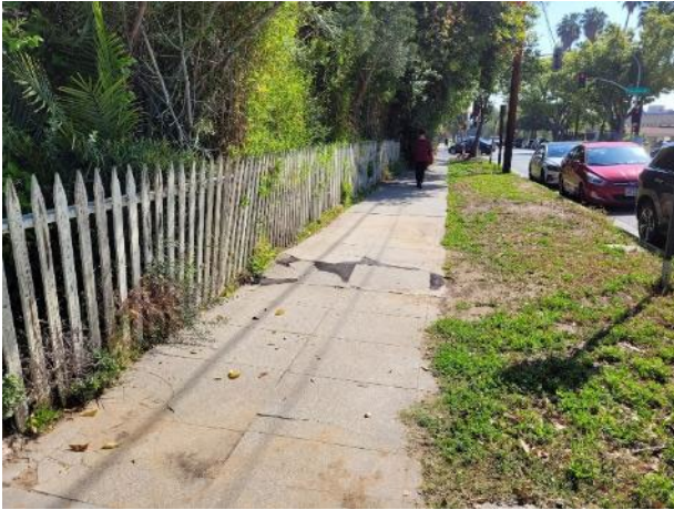
Photo 2 Asphalt sidewalk, shown here on St. John Avenue, provides uneven walking surface. Utilities obstruct path of travel.
