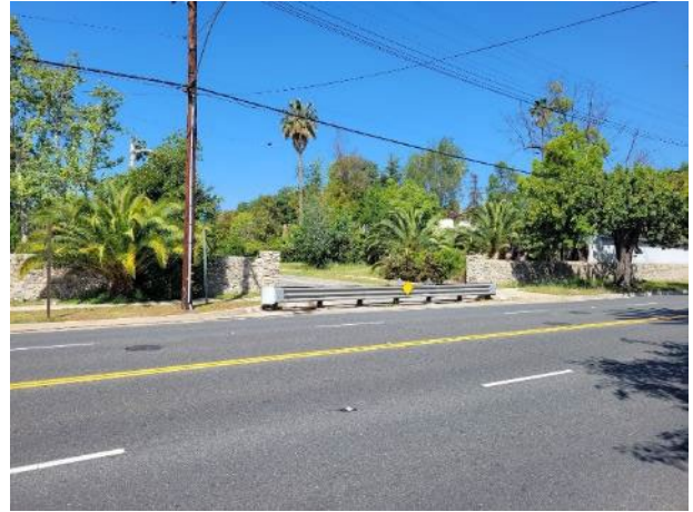
Photo 5 High vehicle speeds on St. John Avenue, south of the SR 710 off ramp, challenge movement between parking and parks.
