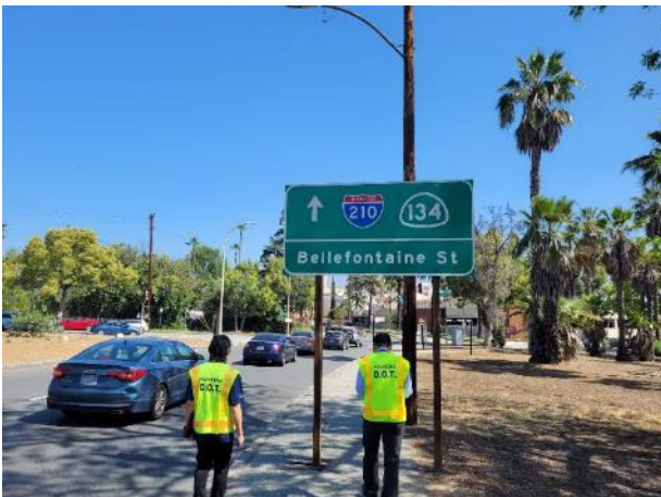
Photo 3 Caltrans signage extends into path of travel along asphalt sidewalk, shown here on Pasadena Avenue.
