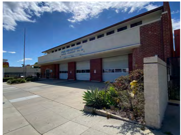
Fire Station 33, located in the subarea.
