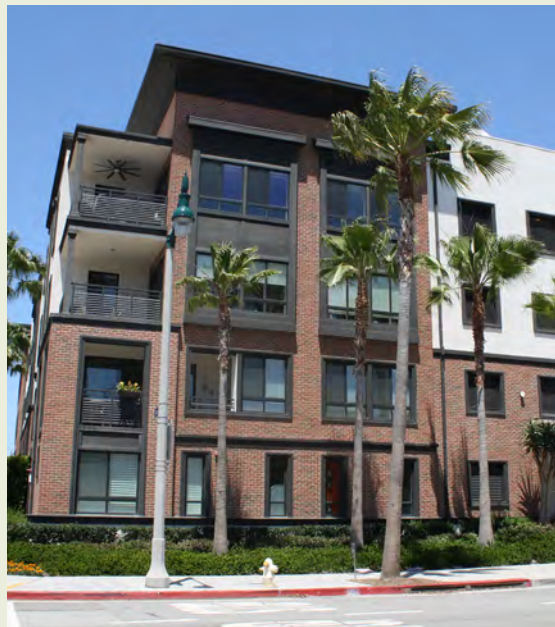
An approximately 51', 4-story building.
