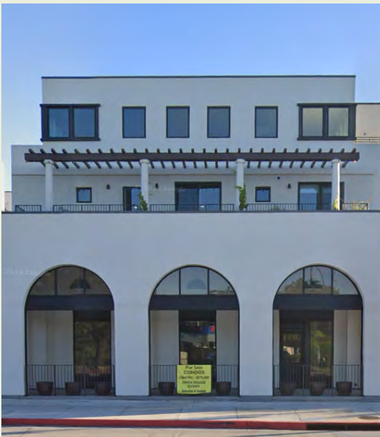
An approximately 39', 3-story building.
