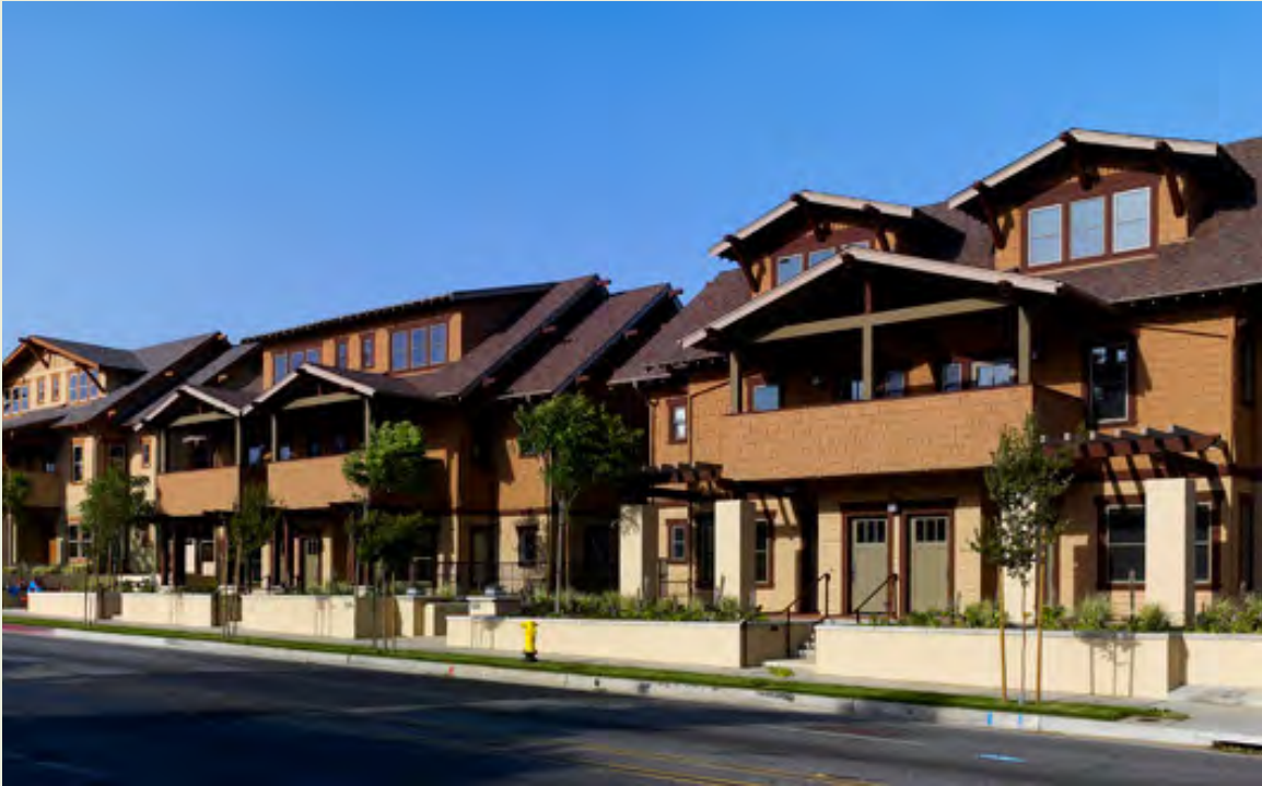
An approximately 35', 3-story building.
