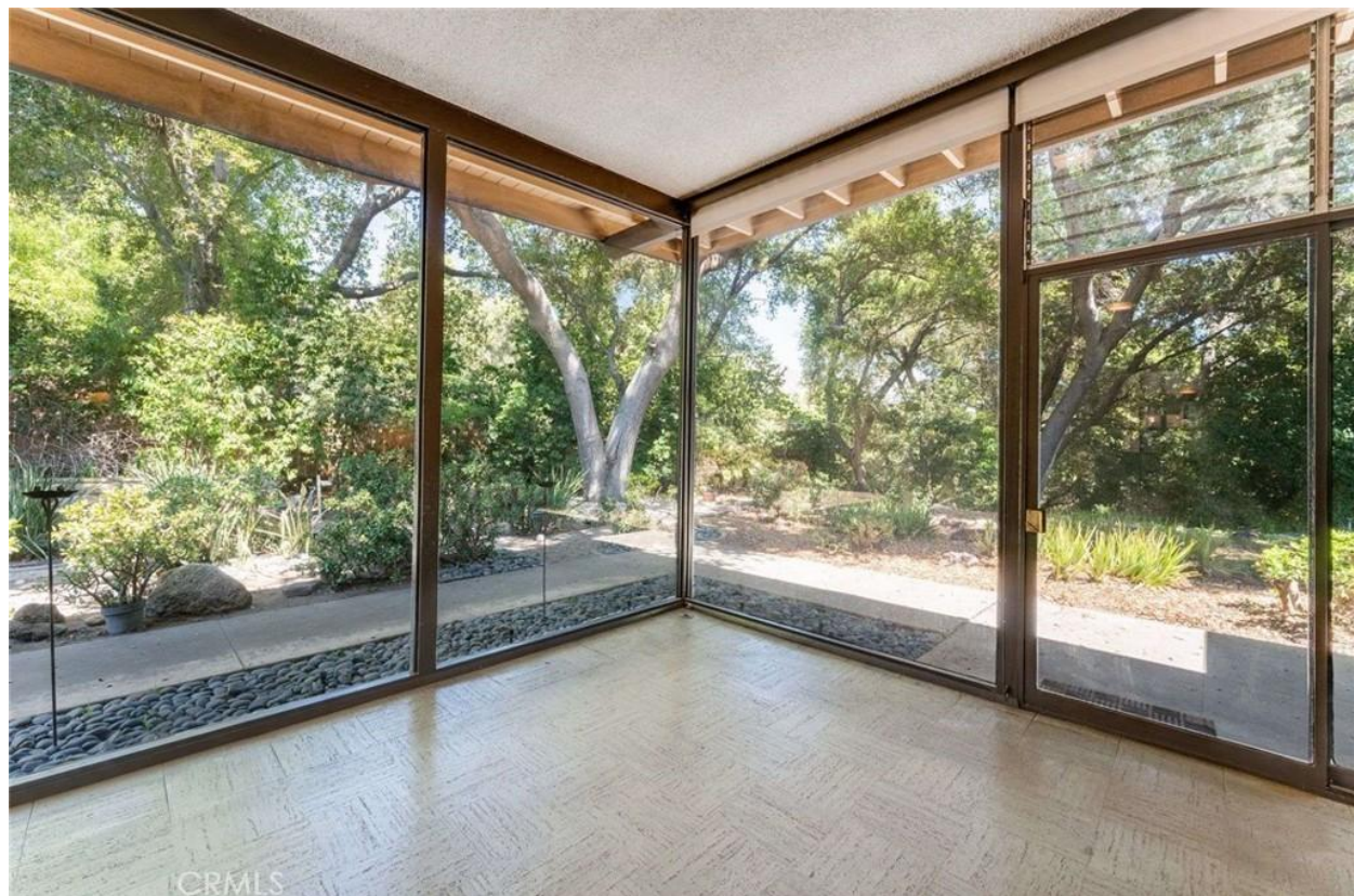
Interior View Facing Northeast
