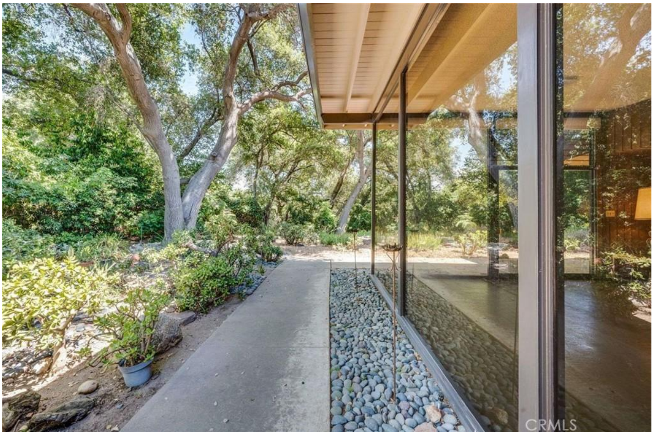
View Facing North along East Elevation
