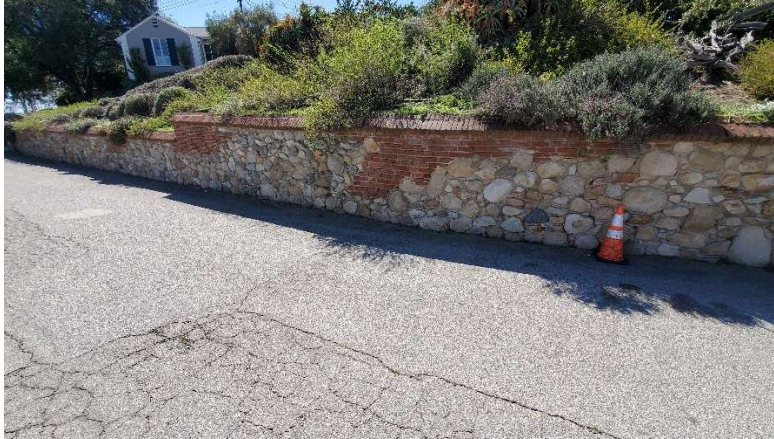
North Wall Section (orange cone is at property line 375 left, 353 right)
