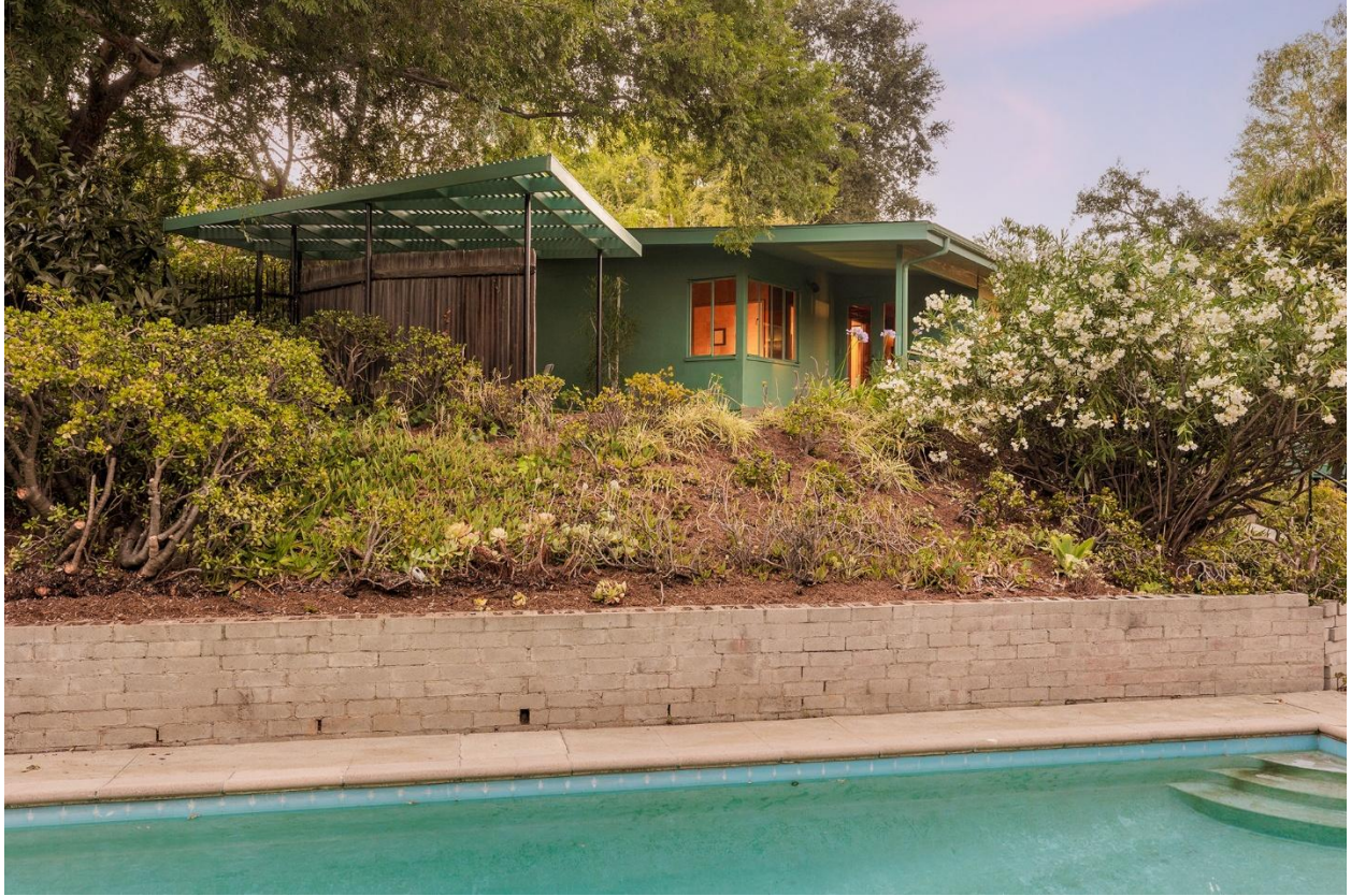
Rear (southwest) elevation looking northwest from pool level
