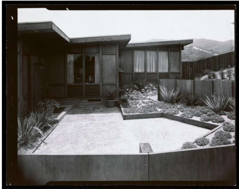
Front (northeast) elevation looking southwest
