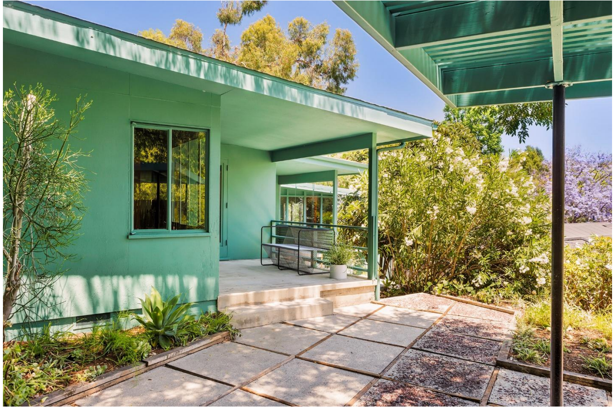
Rear (southwest) elevation looking northeast
