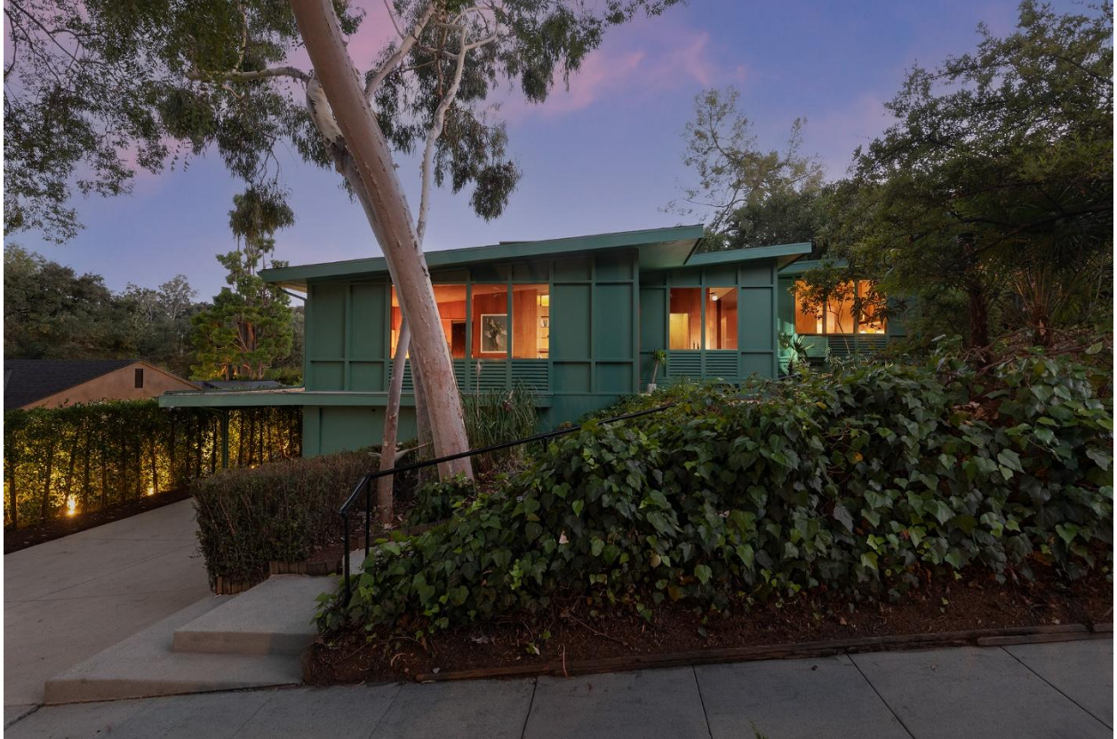
Front (northeast) elevation looking southwest
