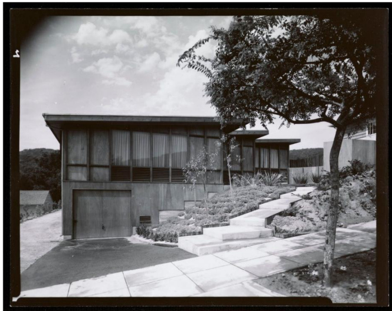
Front (northeast) elevation looking southwest
