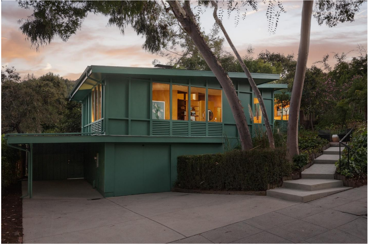
Front (northeast) and southeast elevations looking west
