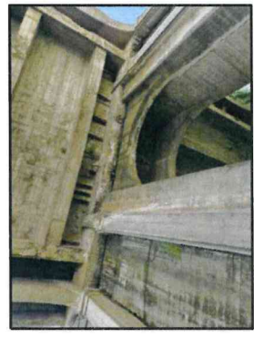
③: Spall Repair on Transverse Girders @ Pier 2
