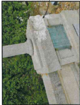
③ : Pedestal Spill Repair
