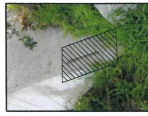
④ : Spall Repair on Pier 15 (North Column).
