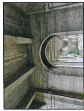
②: Crack Repair along Soffit
