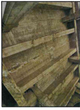
⑤: Span 3 crack repair along soffit
