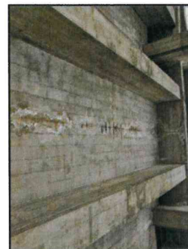
13 : Spall Repair and Crack Repair on Span 11 Soffit and Exterior Girder. (North Girder Shown, South Girder similar)
