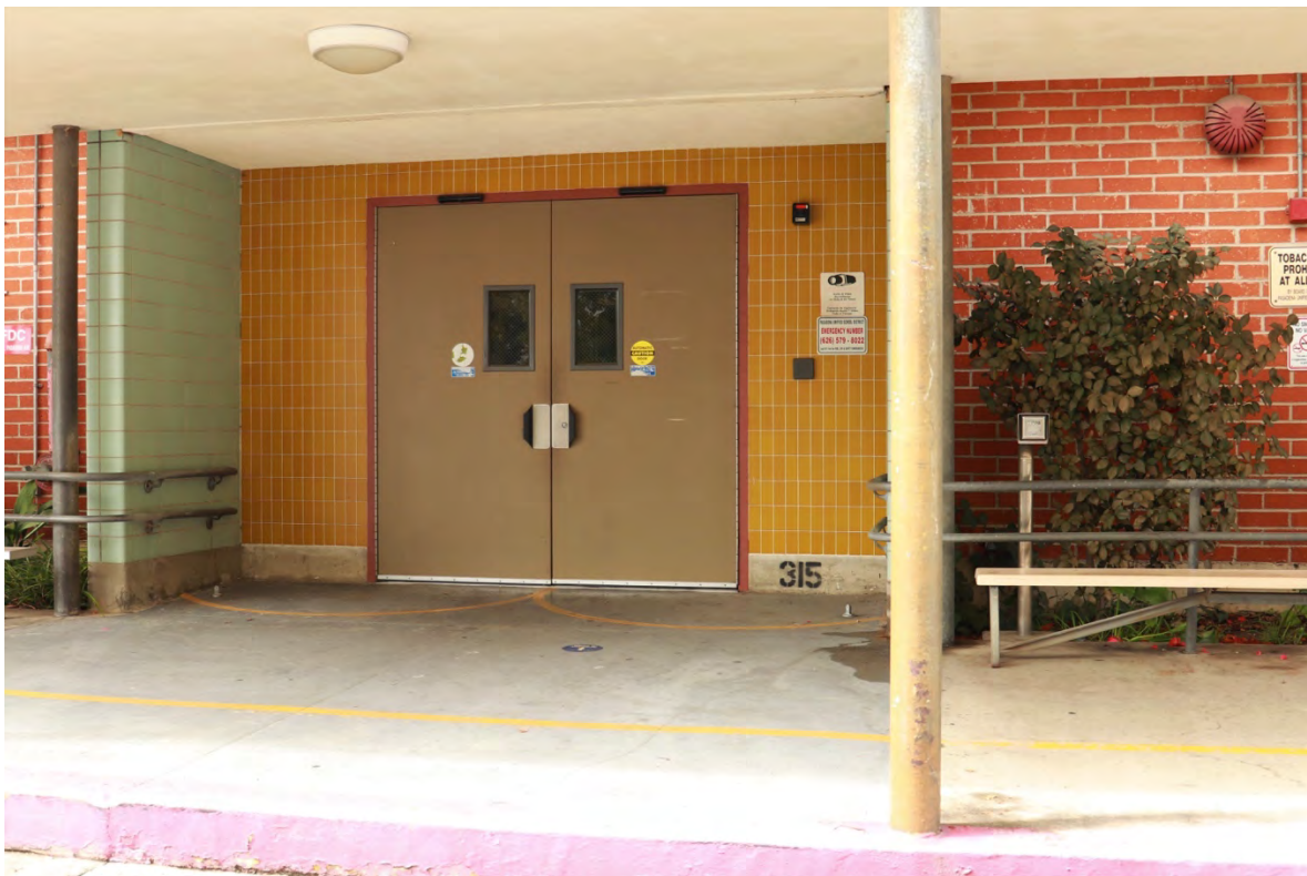
Figure 28. Detail of main entrance, with automated doors, each of which measures 4.5 feet (the minimum width for ADA access defined later was 32 inches)
