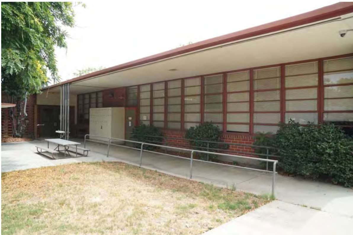
Figure 42. South Wing classrooms, with patterned brick, wide sheltering roof eaves, and continuous band of multi-light windows
