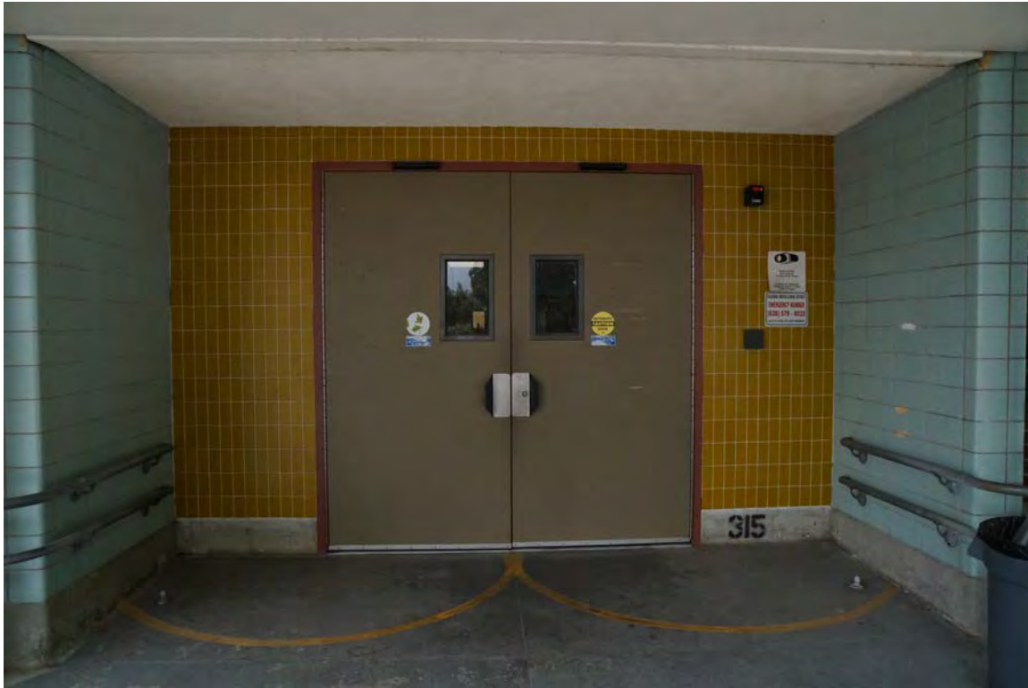
Figure 18. Detail of entrance, with automated door opener, double-height hand-railings, brick sheathing, and tile-clad wing walls
