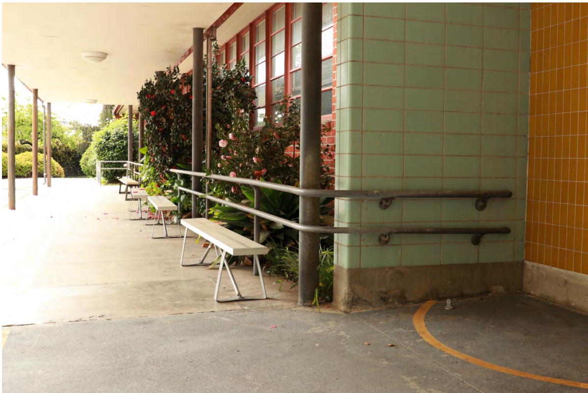
Figure 24. Double-height hand railings optimize accessibility throughout the interior and exterior
