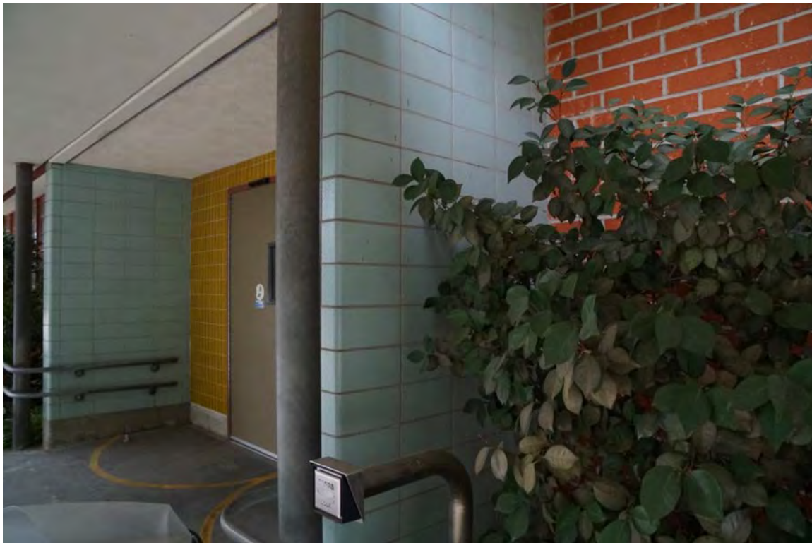
Figure 18. Detail of entrance, with automated door opener, double-height hand-railings, brick sheathing, and tile-clad wing walls
