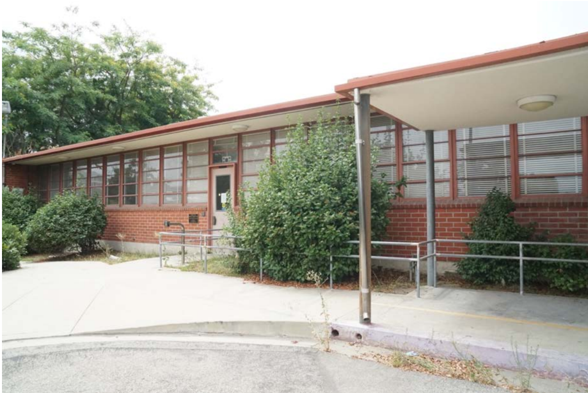
Figure 22. Sheltered entrance patio with landscaping and wide roof eaves with continuous bands of multi-light windows; double-height hand-railings optimize accessibility
