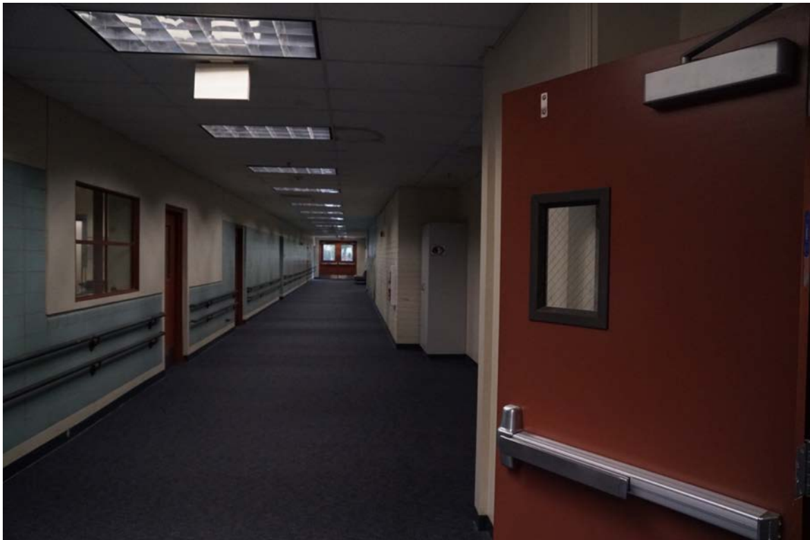
Figure 53. Double-height hand railings, and the absence of stairs or threshold changes, optimize accessibility throughout the interior
