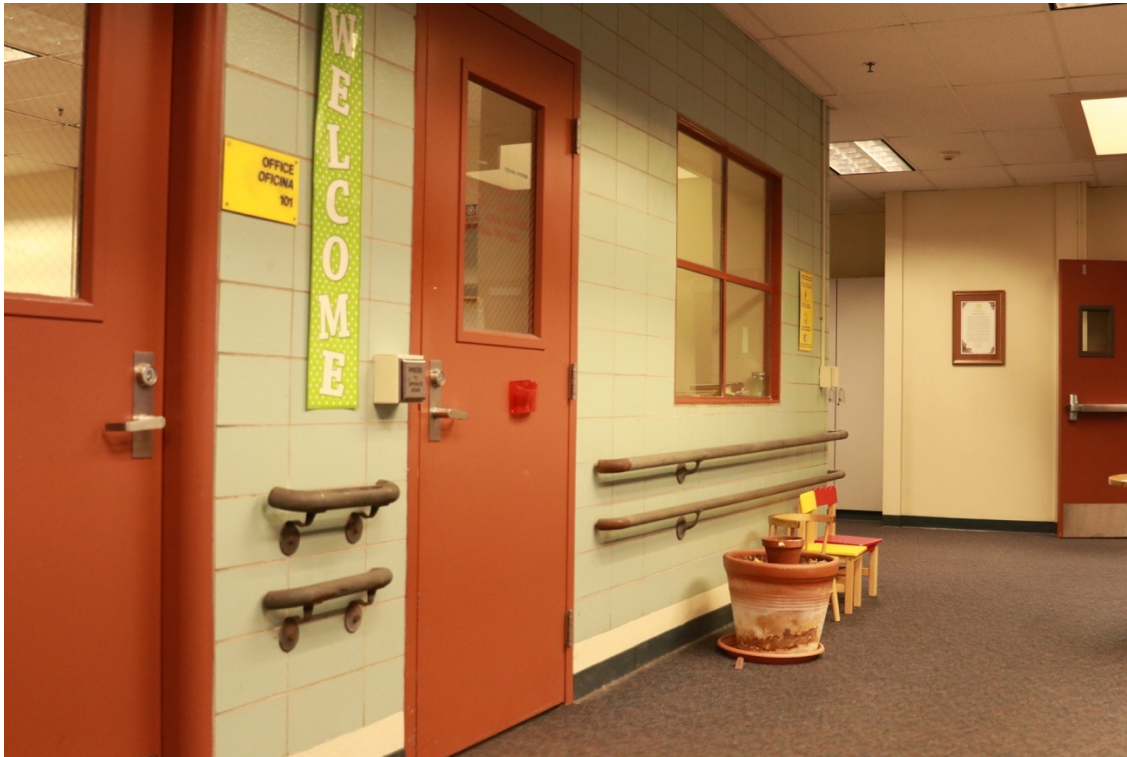
Figure 47. Double-height hand railings optimize accessibility throughout the interior and exterior
