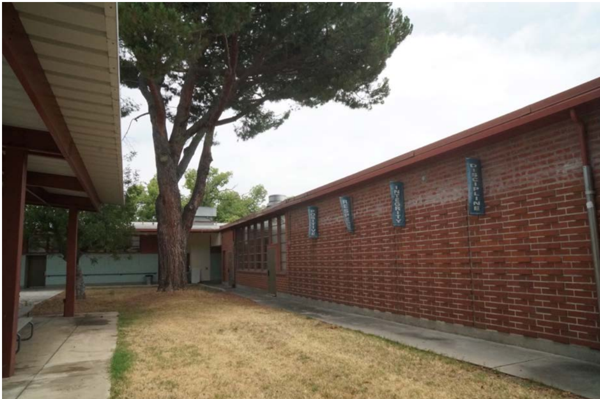
Figure 38. Lunch shelter on left and extension of Central Wing on right; the change in brick patterns marks the area of the extension in circa 1970
