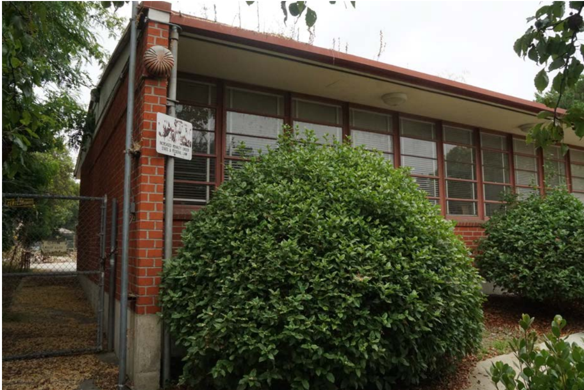
Figure 23. Corner of façade (east elevation) and south elevation, with continuous bands of multi-light windows looking out on landscaping, enhancing indoor-outdoor integration
