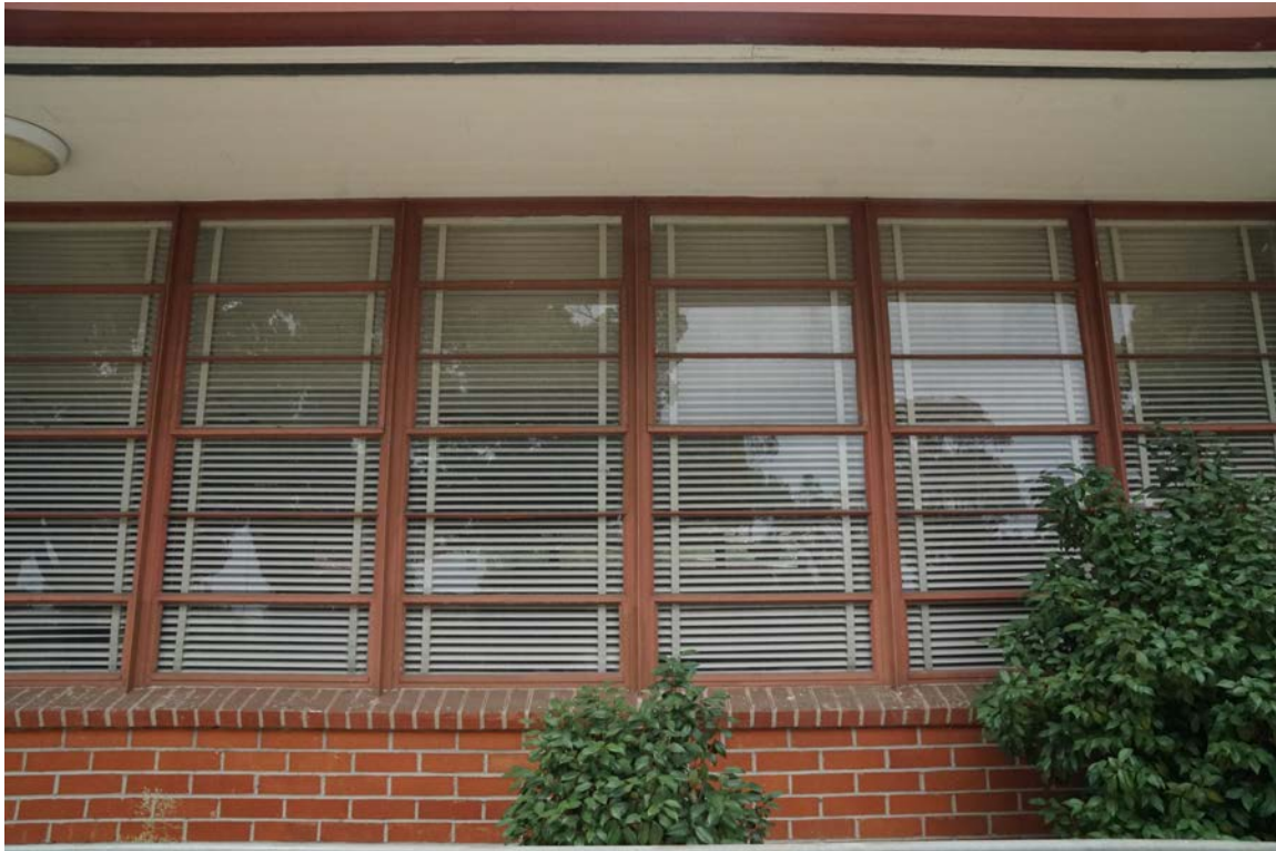
Figure 19. Roosevelt School, detail of brick walls and window sills and original windows; the school retains original multi-light sashes throughout campus
