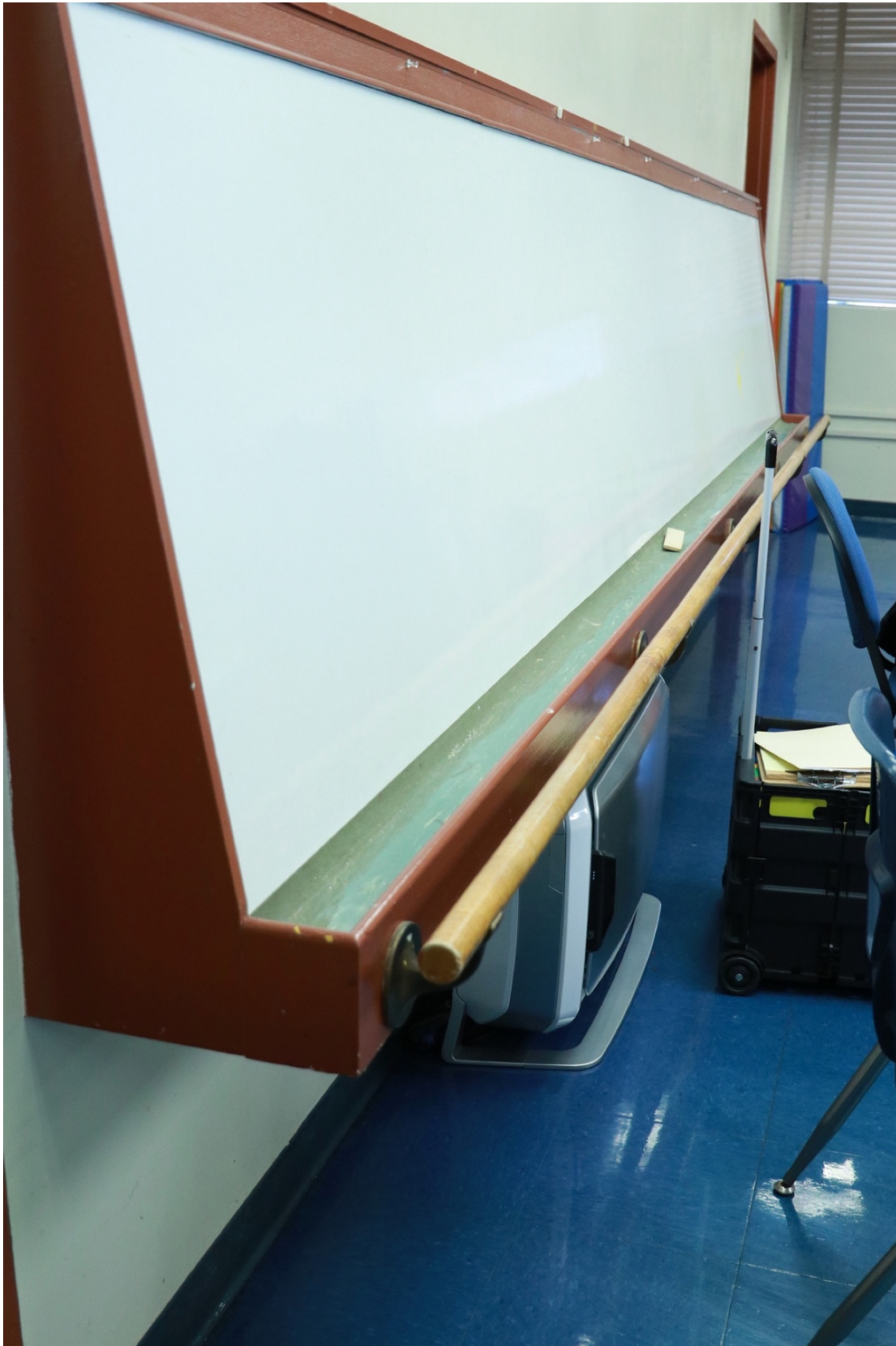
Figure 54. Sloped easels with handrailings
