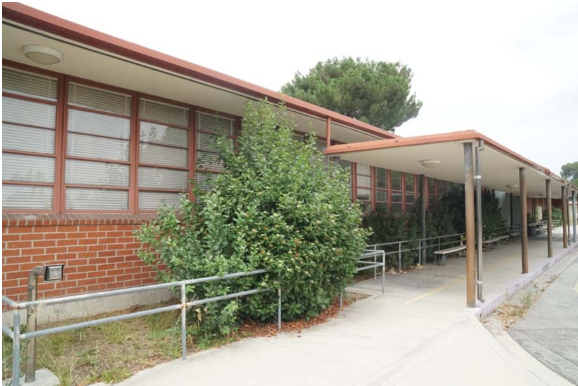
Figure 22. Sheltered entrance patio with landscaping and wide roof eaves with continuous bands of multi-light windows; double-height hand-railings optimize accessibility
