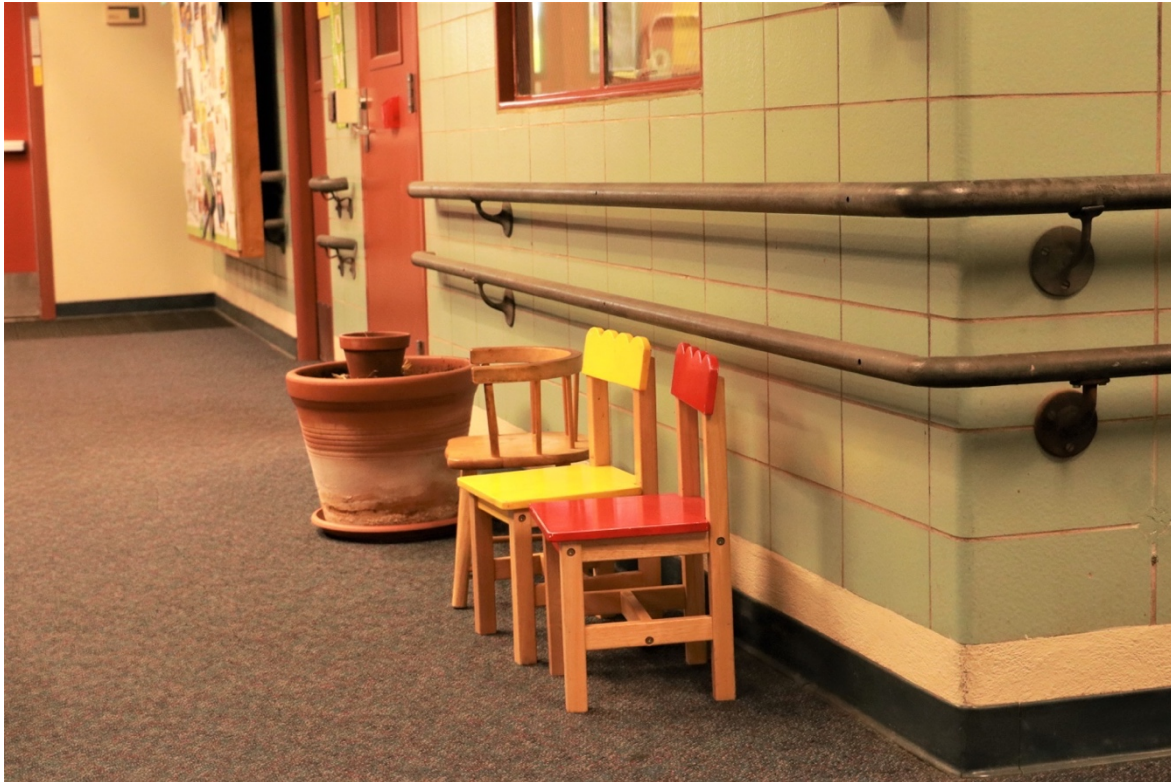
Figure 53. Double-height hand railings, and the absence of stairs or threshold changes, optimize accessibility throughout the interior
