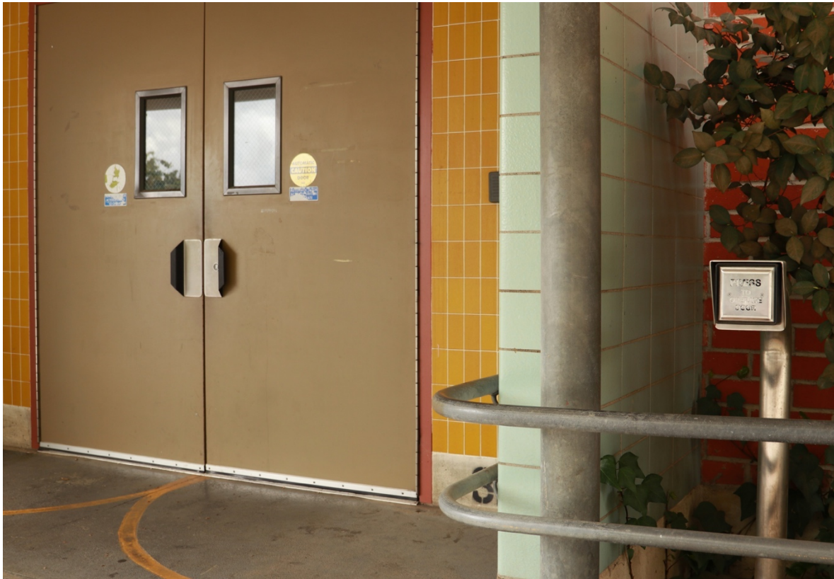
Figure 28. Detail of main entrance, with automated doors, each of which measures 4.5 feet (the minimum width for ADA access defined later was 32 inches)
