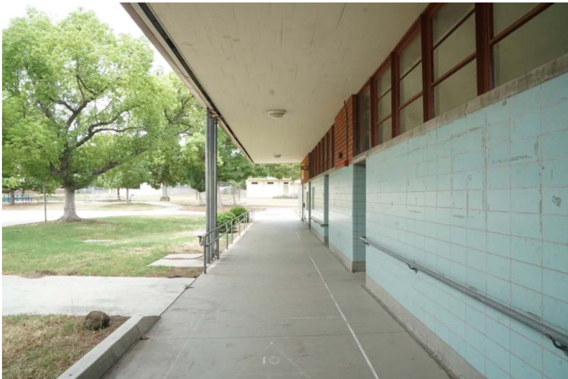
Figure 32. Main Wing, facing interior courtyard, shelters over exterior walkways (a key feature of postwar functionalist schools) provide transitional area from interior to courtyard area
