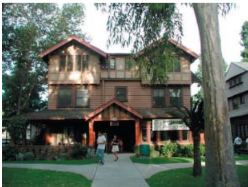
#3 at 130 Oakland Avenue Kreysler Hall
