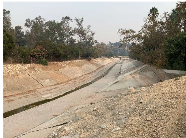
Figure 1-1. San Pascual Site, South Pasadena/Los Angeles
