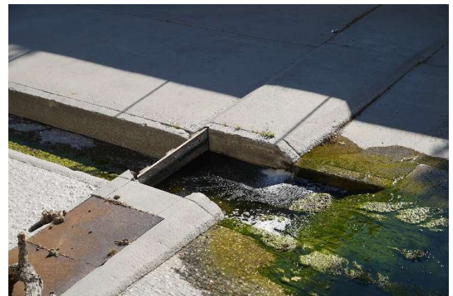
Figure 1-2. Existing Diversion within Arroyo Seco
