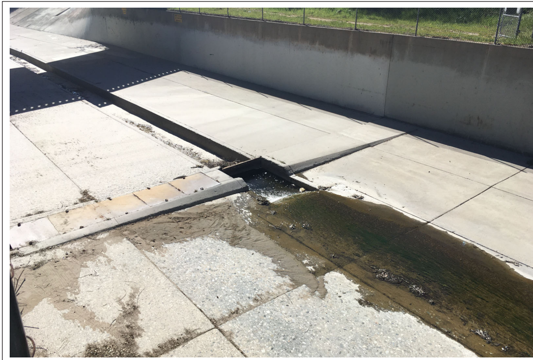
Photo Location 3. February 10, 2022. View of diversion structure in the mainstem Arroyo Seco channel.
