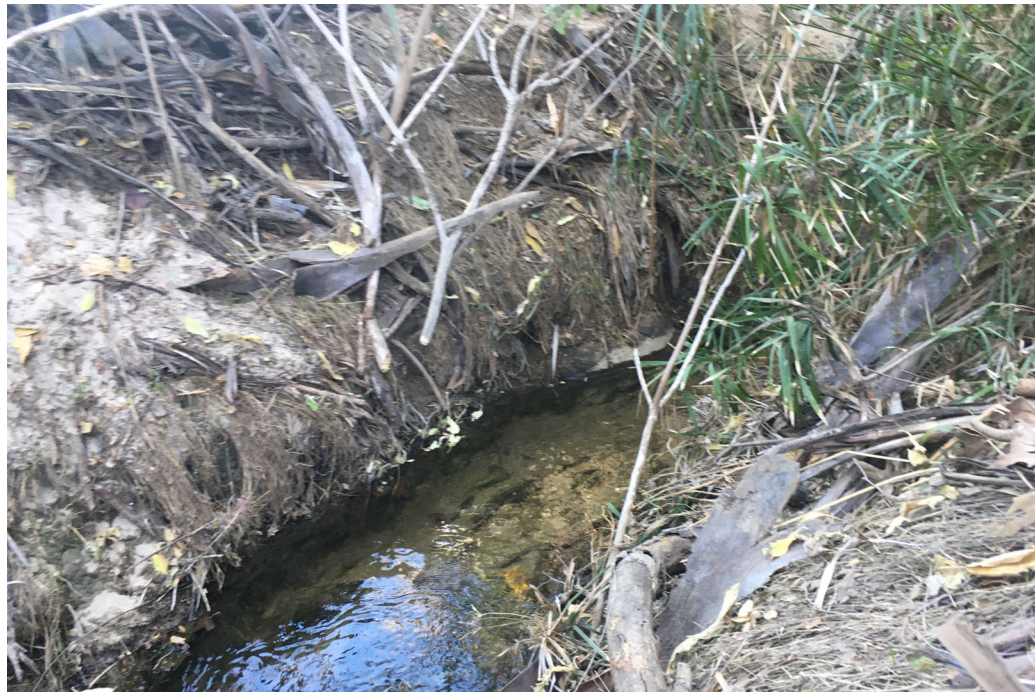
Photo Location 4, facing upstream. February 10, 2022. View of channel conditions in San Pascual Basin area.
