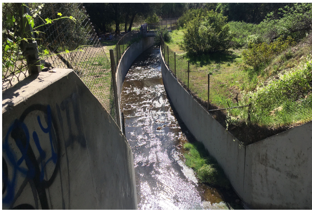
Photo Location 1, facing downstream. February 10, 2022. View of San Rafael Creek.
