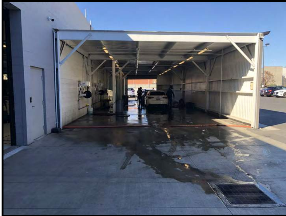
View of the car wash area north of the service area.
