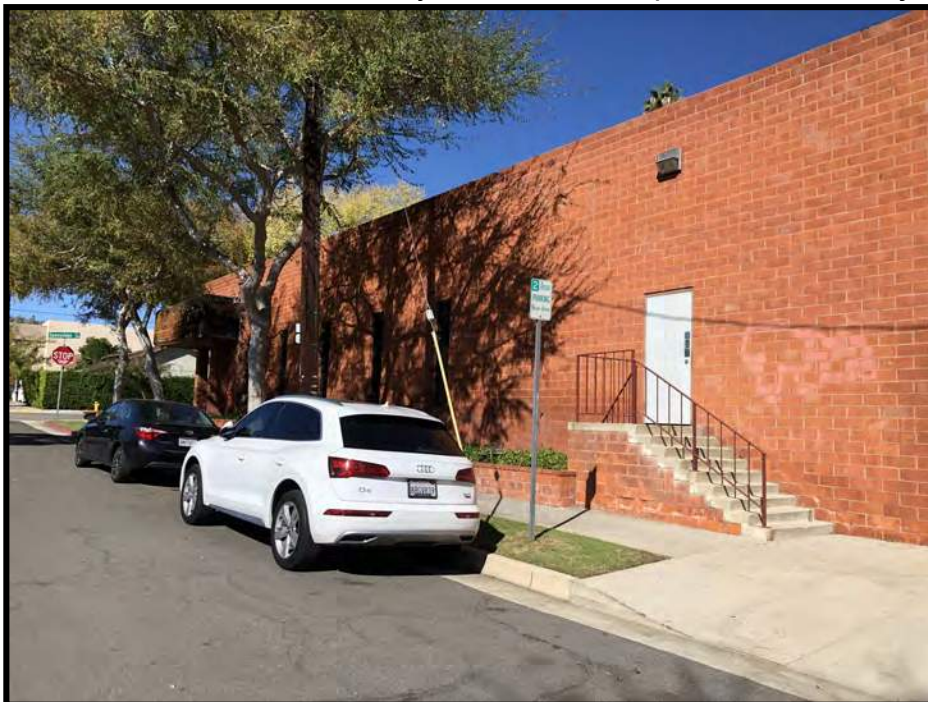
View of some of the industrial buildings in the northwestern corner of the subject property.
