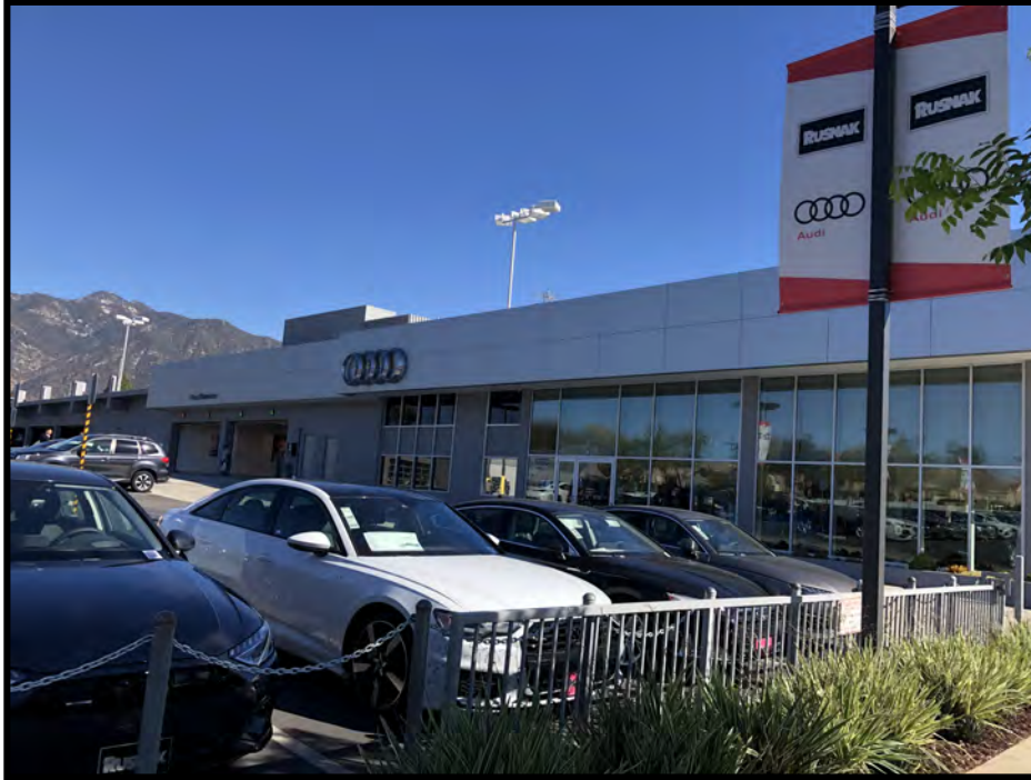
View of the showroom and service facility on the eastern portion of the subject property.
