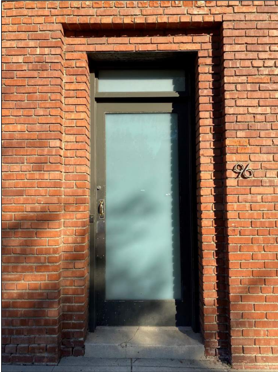
Photograph 5: Original secondary metal-frame entrance in recessed stepped entry along North Sunnyslope Avenue. Camera facing east, October 28, 2021.
