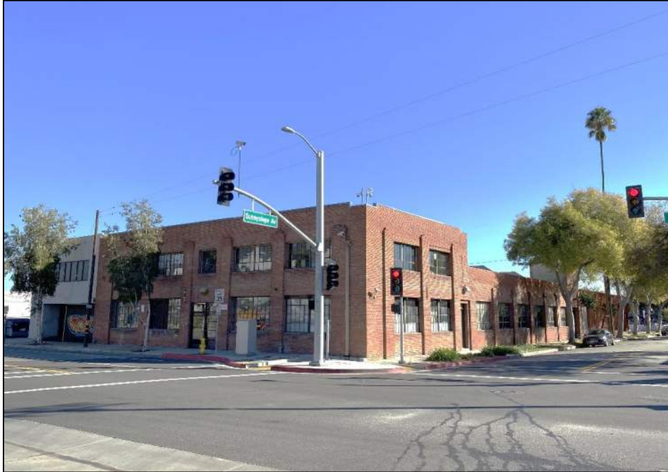
Photograph 2: North and east sides of the factory building, showing portions of the east and south additions. Camera facing southeast, October 28, 2021.
