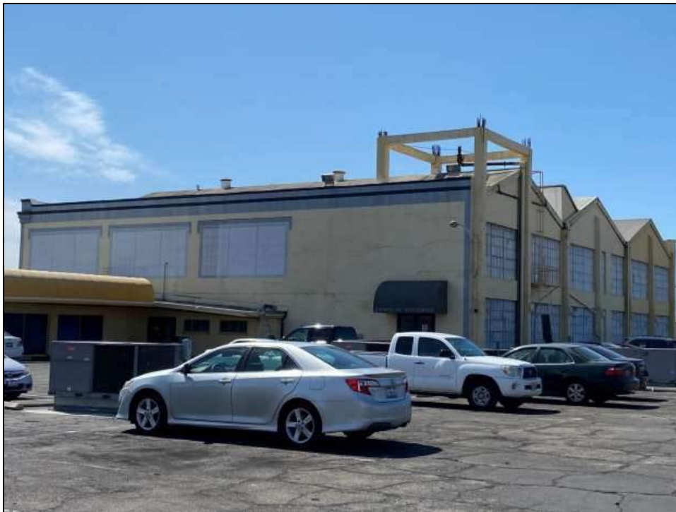
Figure 10: West and south elevations of the daylight factory on South Raymond Avenue, showing roof profile and fenestration (Reyes 2021).
