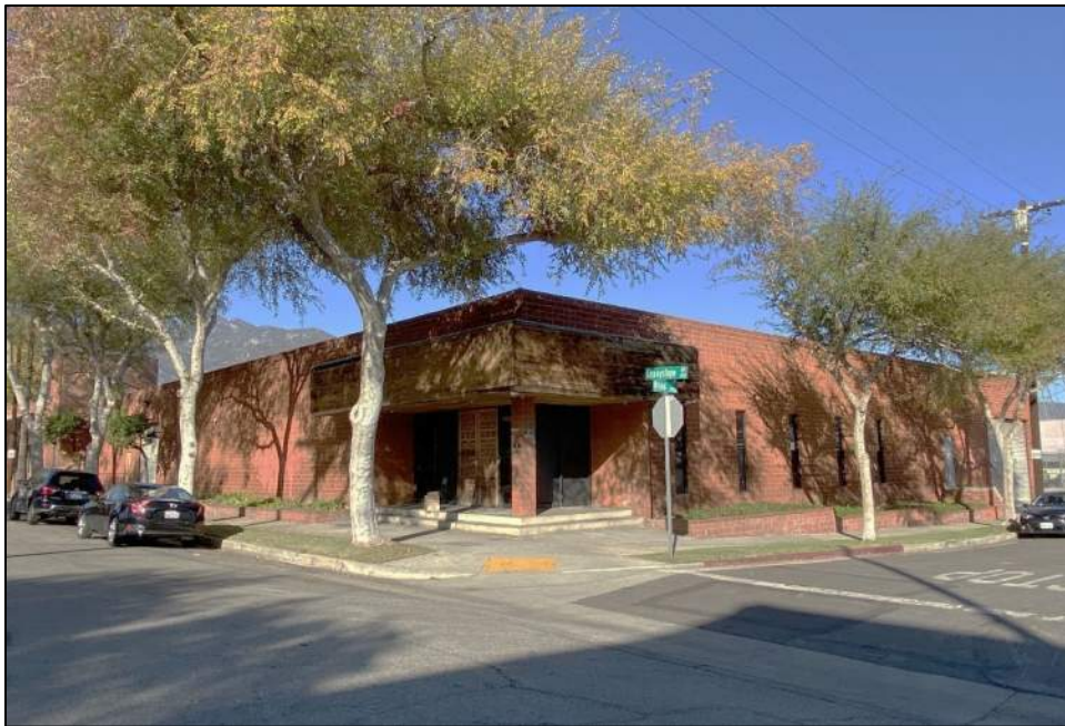
Photograph 7: Addition constructed in 1979 at 60 North Sunnyslope Avenue. Camera facing northeast, October 28, 2021.
