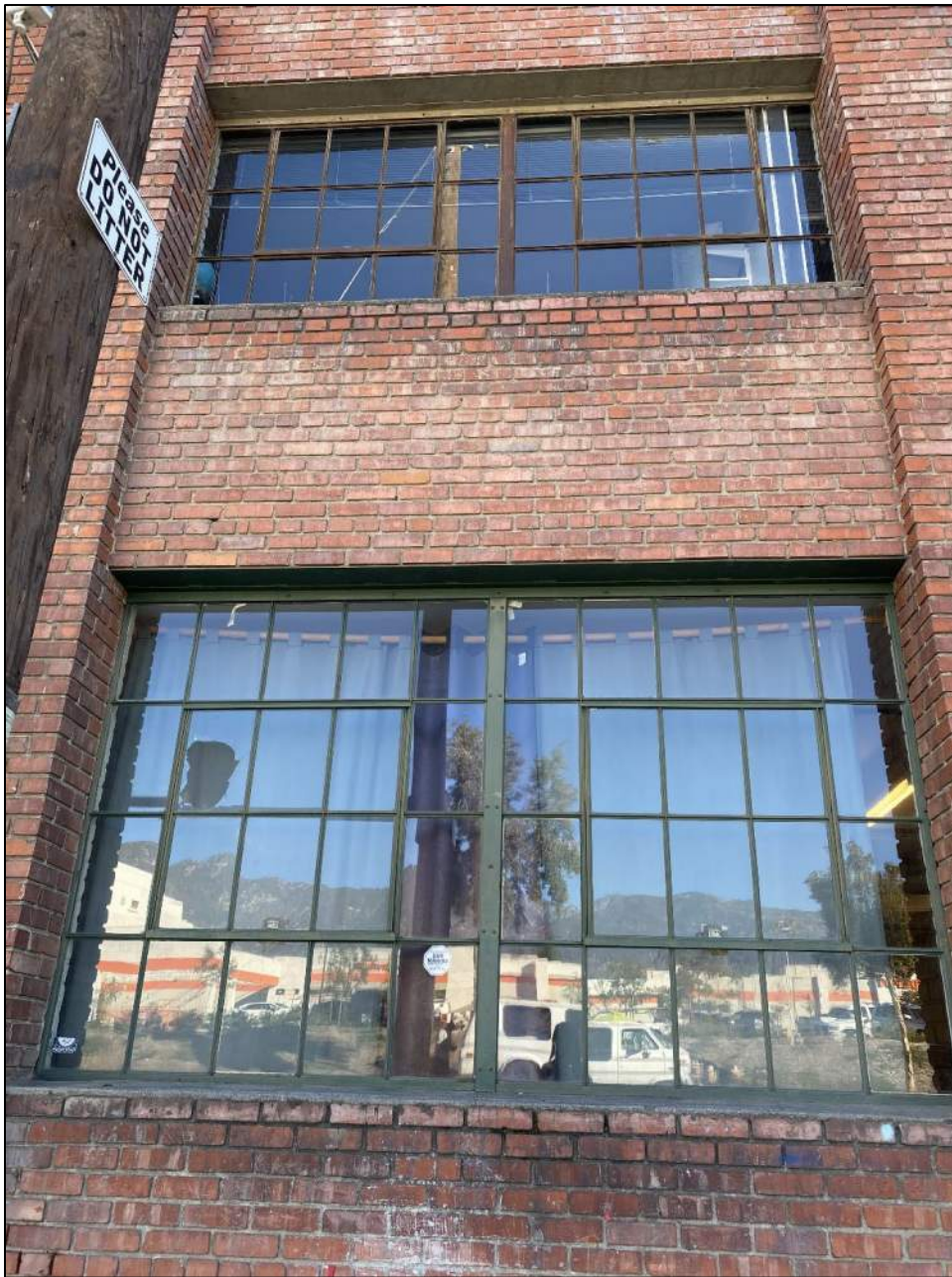
Photograph 4: Detail view of steel-sash windows and brickwork. Camera facing south, October 28, 2021.
