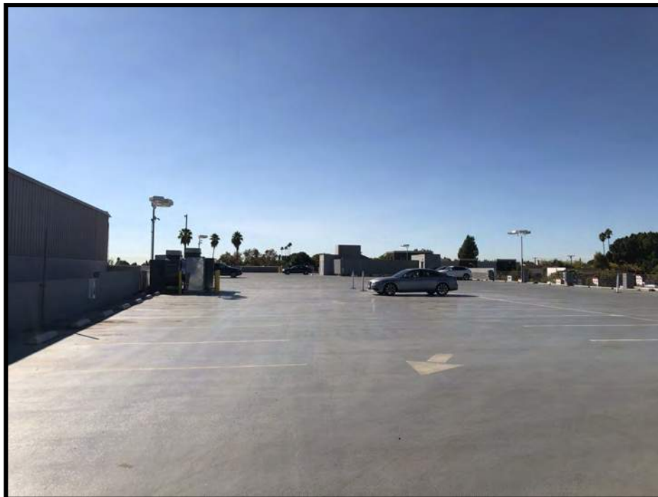
View of the parking area on the 2 nd floor, above the service area, of the Rusnak building.
