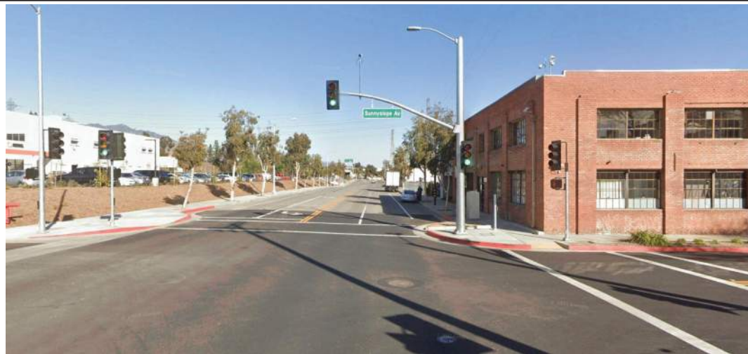
Photograph 01: View at the intersection of Walnut Street and North Sunnyslope Avenue facing east along Walnut Street, at the northwest corner of the Project site (on the right).
