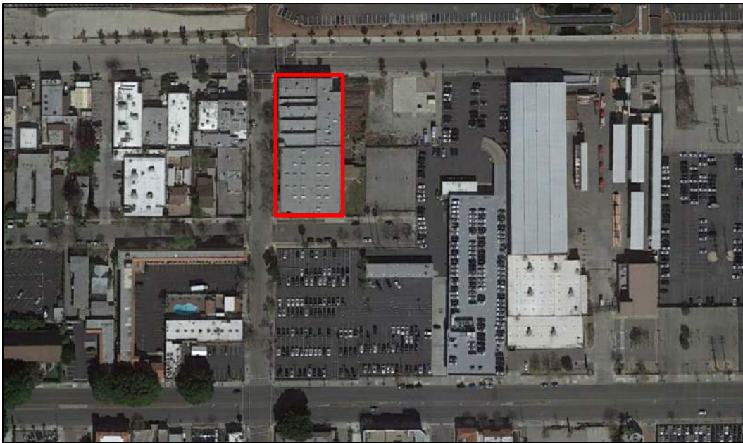
Figure 7: Google Earth aerial photograph, dated February 20, 2021, showing the present footprint of 2914 East Walnut Street, 2926 East Walnut Street, and 60 North Sunnyslope Avenue (Google Earth 2021).
