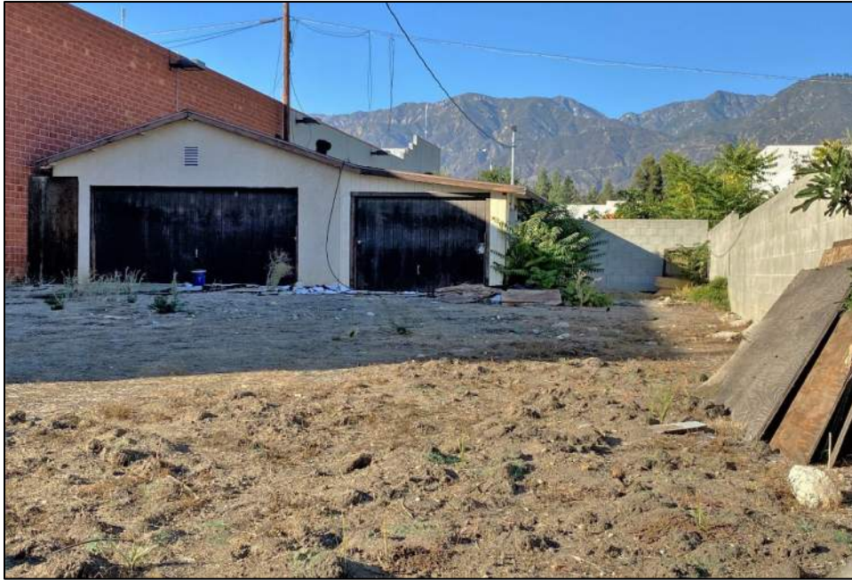
Photograph 8: Detached garage building located east of the addition constructed in 1979. Camera facing north, October 28, 2021.
