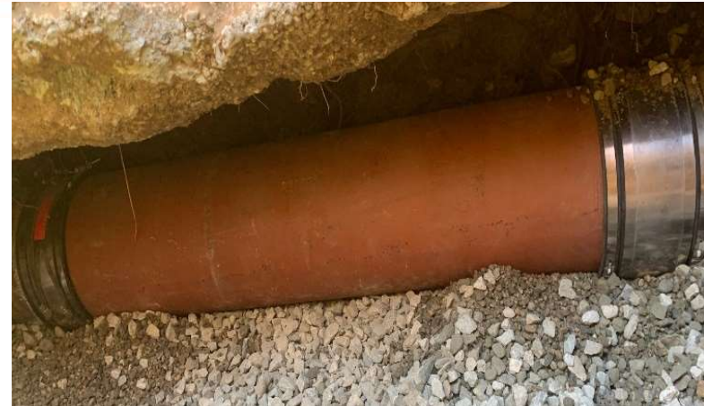
Completed Sewer Line Replacement
