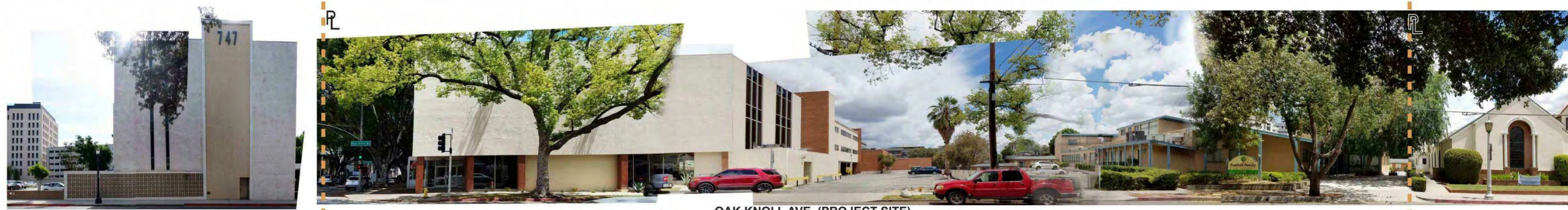
A OAK KNOLL AVE - PROJECT SITE
