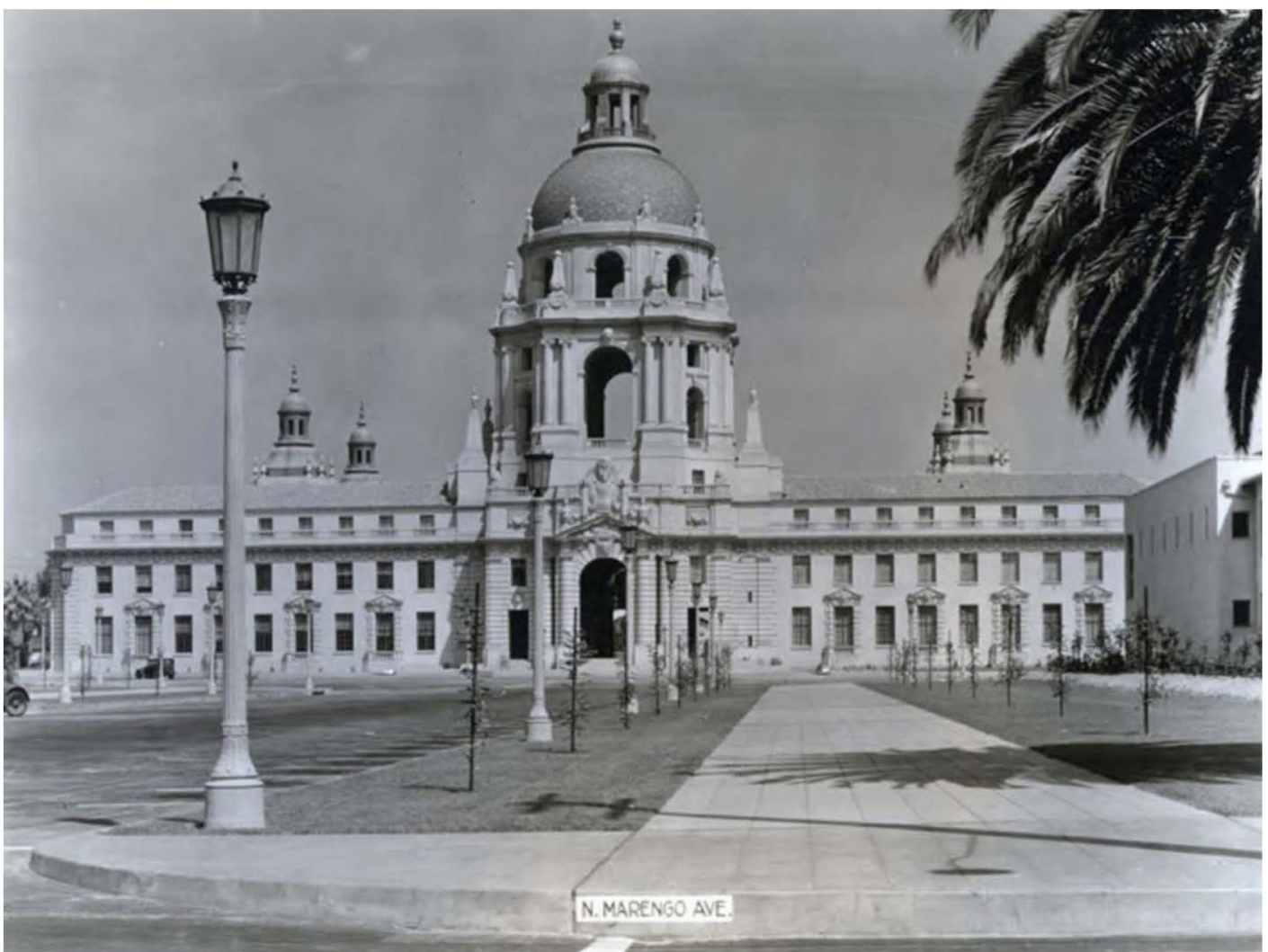
PASADENA CITY HALL, BAKEWELL & BROWN ARCHITECTS, 1927
