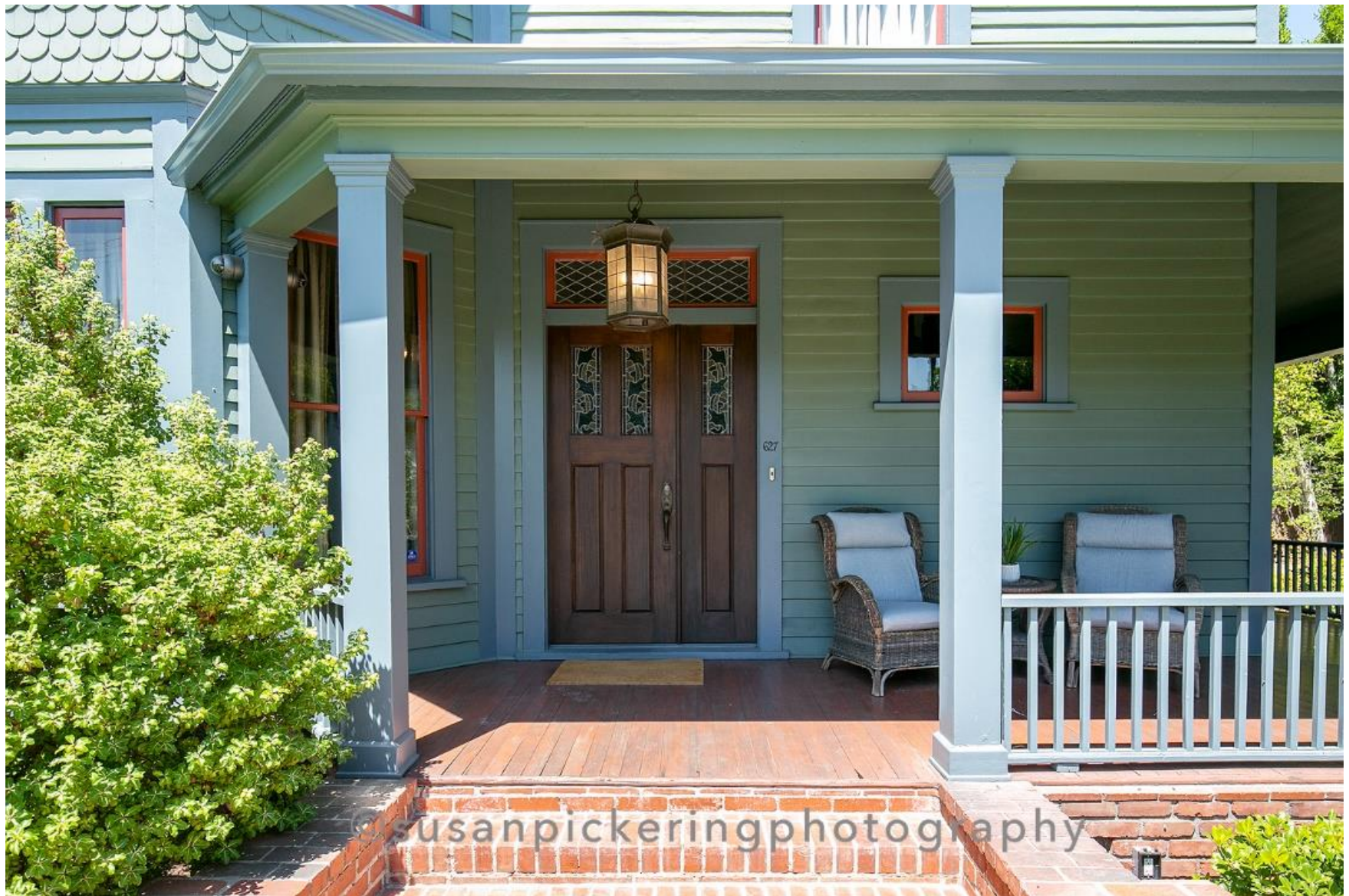
Primary Entry (East Elevation)
