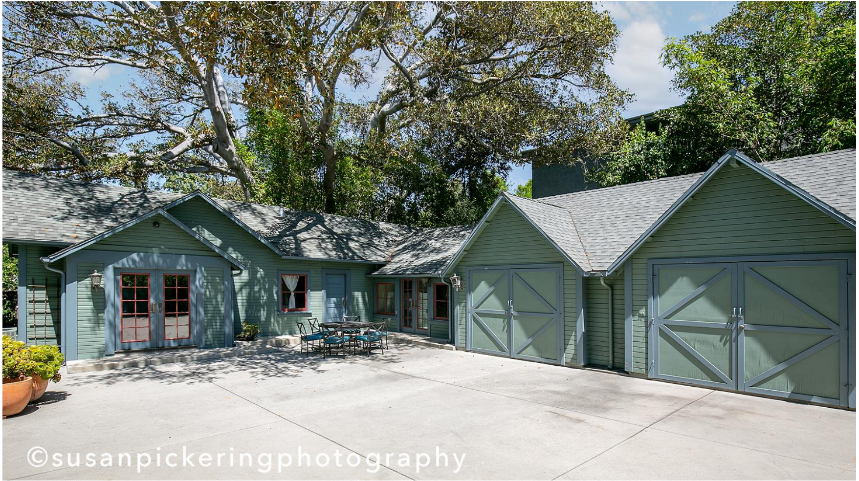
Carriage House (Left) and Garage (Right)
