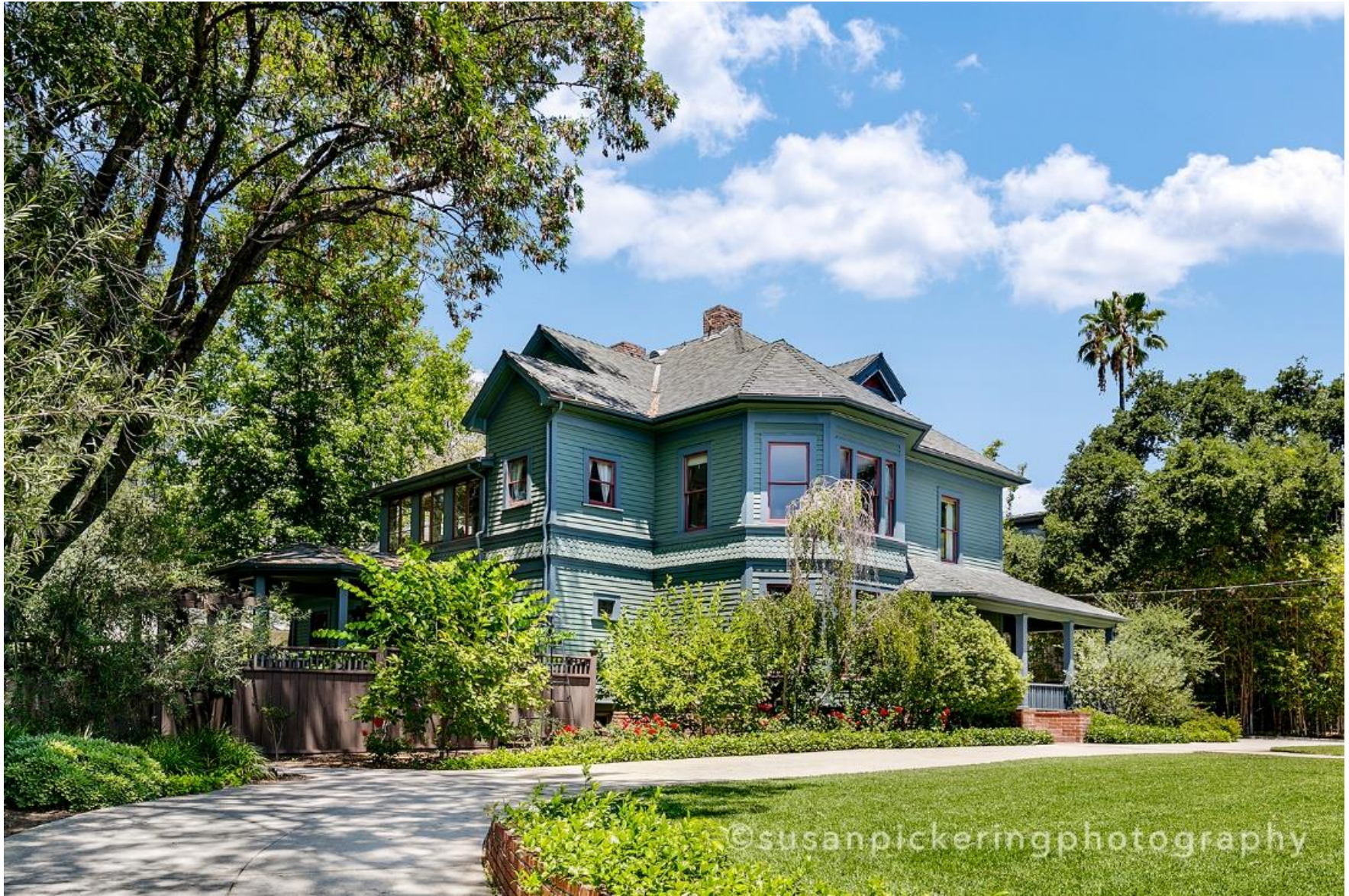
Front (East) and South Elevations
