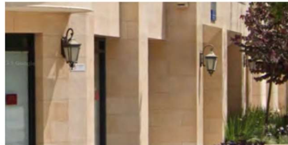
Light fixtures in which lightbulbs are fully enclosed support improved safety and cleanliness.
