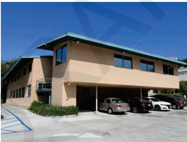
Figure 19. Building 5: South and East Elevations, View looking northwest (IMG_8497)
