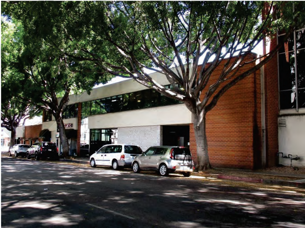
Figure 2. Building 2: Right section of North Elevation, View looking southeast (IMG_0496)
