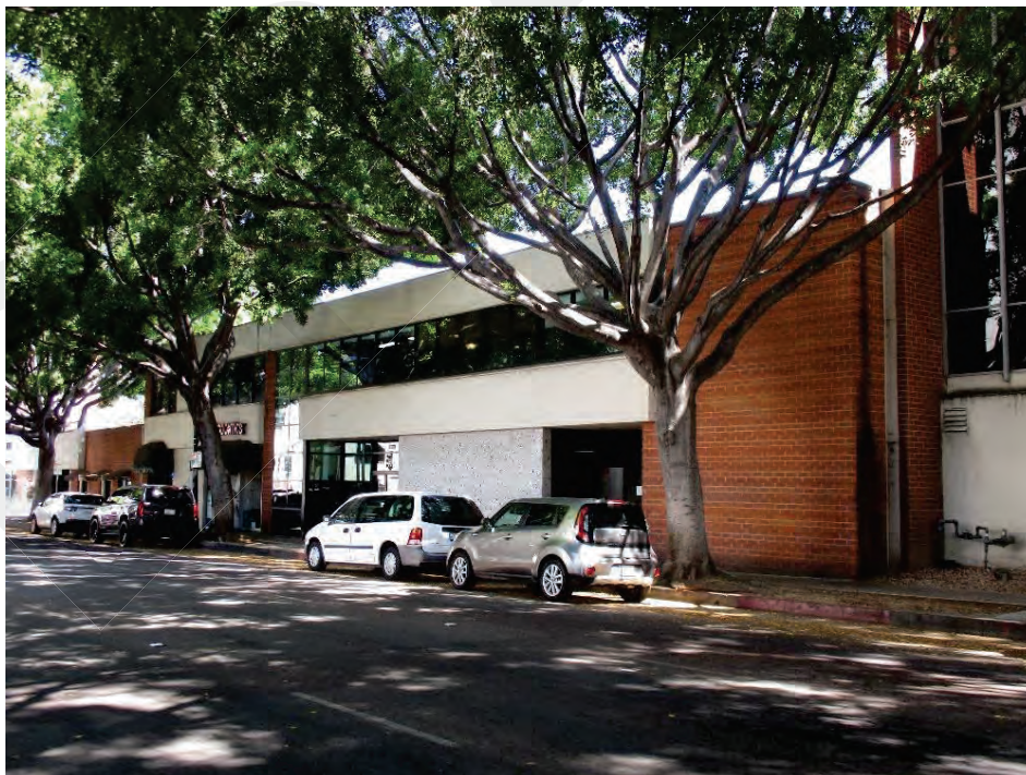
Figure 9. Building 2: Right section of North Elevation, View looking southeast (IMG_0496)
