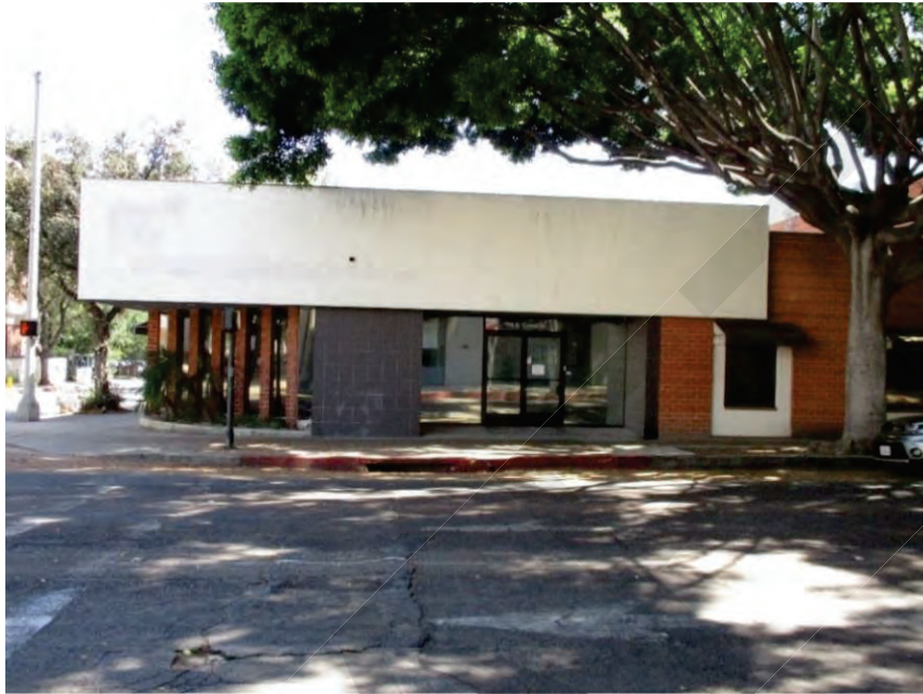
Figure 1. Building 3: North elevation, View looking south (IMG_0484)
