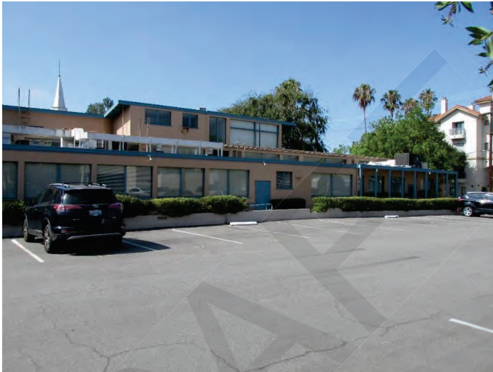
Figure 3. Building 5: North Elevation, View looking southwest (IMG_8506)
