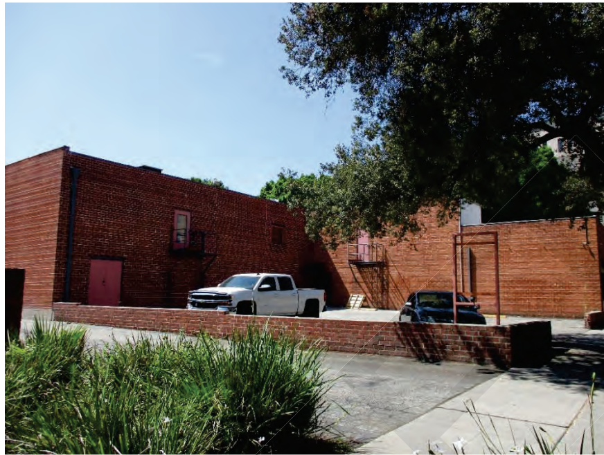
Figure 12. Building 3: South elevation, View looking northwest (IMG_0463)
