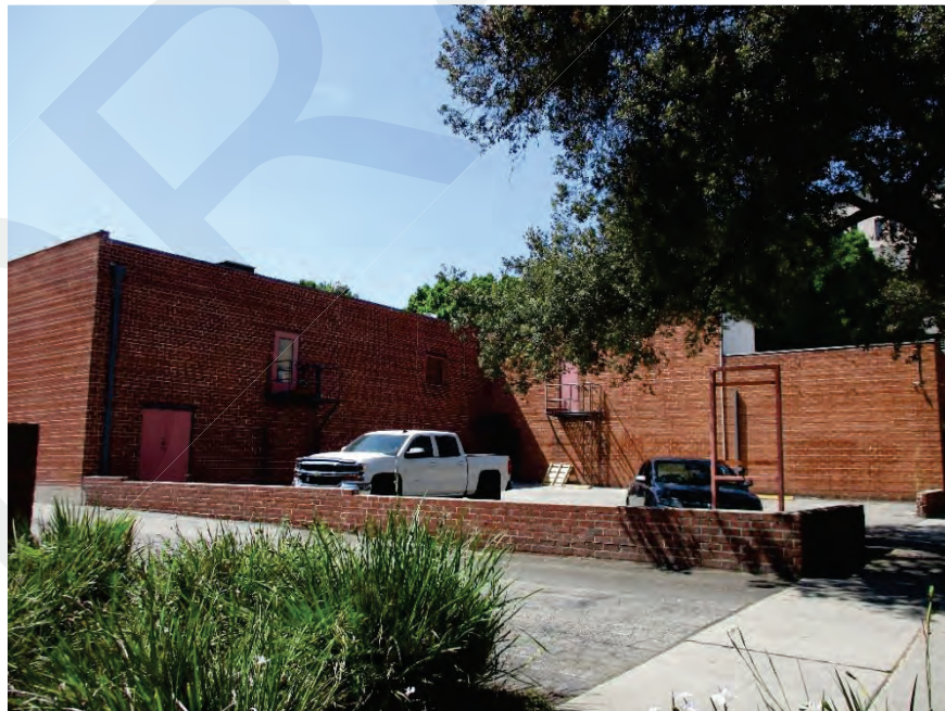
Figure 2. Building 3: South elevation, View looking northwest (IMG_0463)
