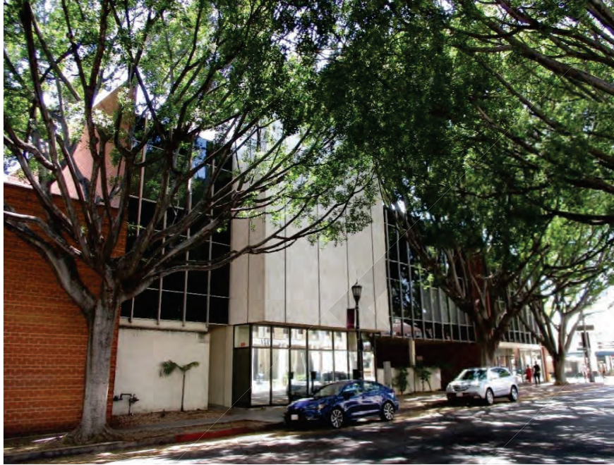
Figure 1. Building 1: North Elevation, View looking southwest (IMG_0362)
