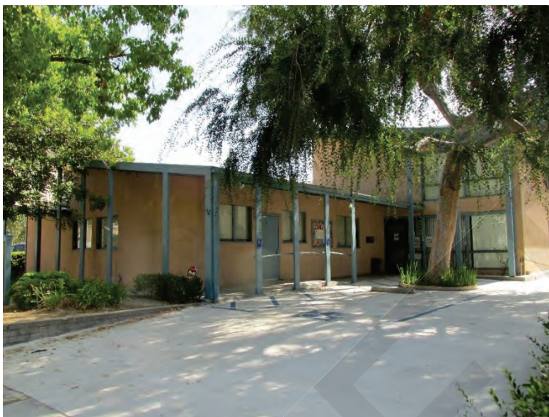
Figure 18. Building 5: West Elevation, View looking northeast (IMG_8491)
