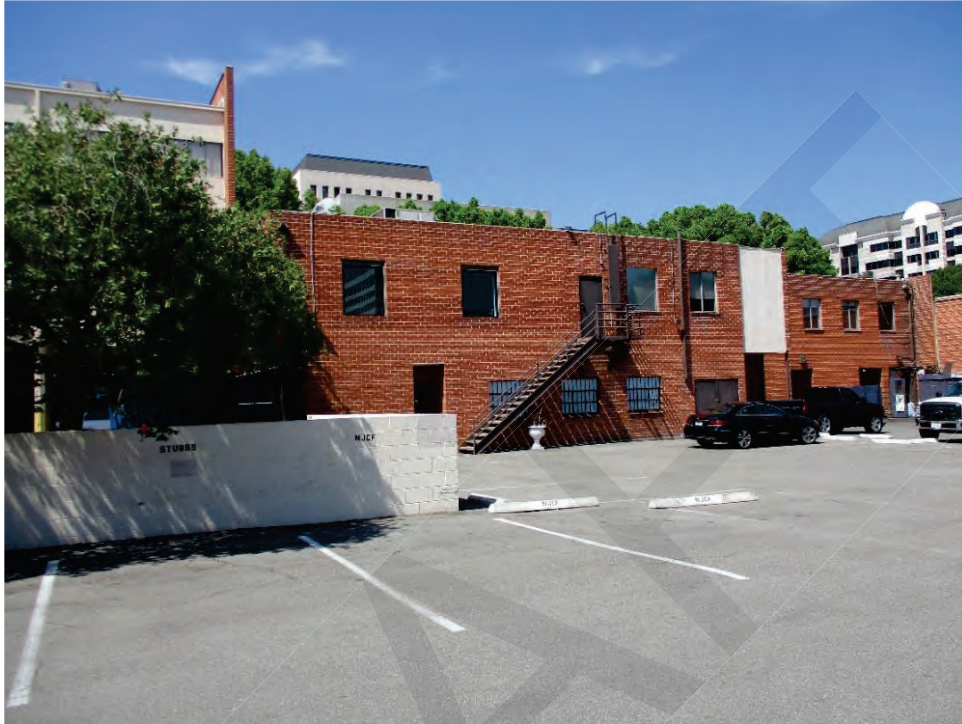
Figure 3. Building 2: South Elevation, View looking northeast (IMG_0455)
