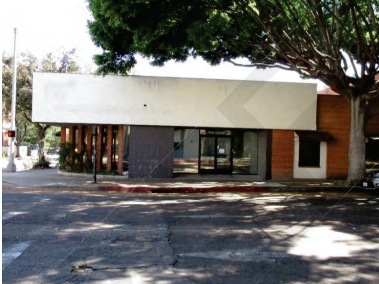
Figure 11. Building 3: North elevation, View looking south (IMG_0484)
