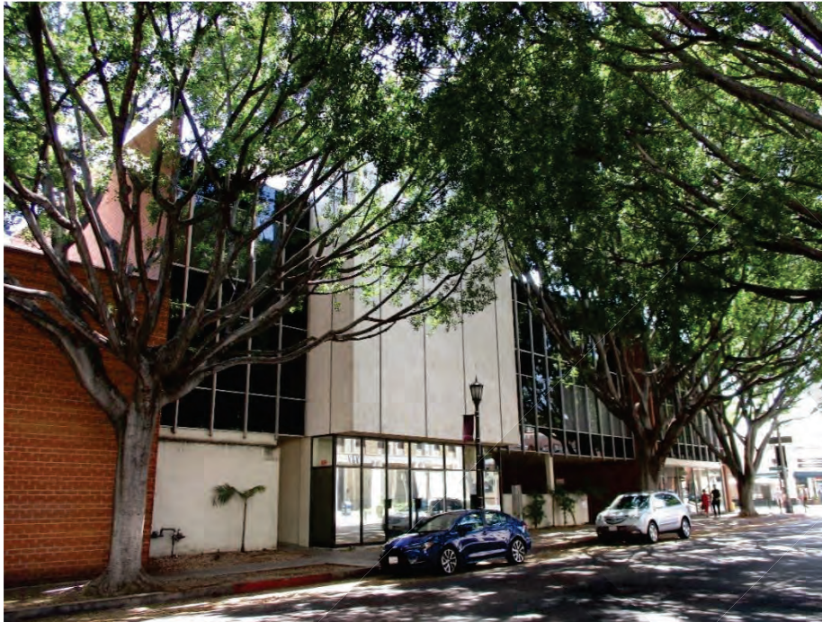
Figure 5. Building 1: North Elevation, View looking southwest (IMG_0362)
