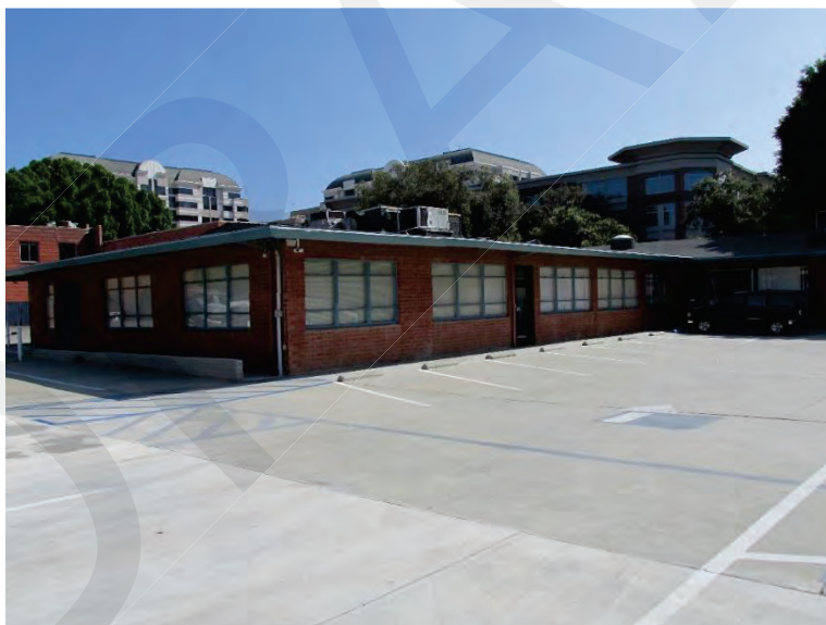
Figure 16. Building 4: West and South Elevations, View looking northeast (IMG_8541)
