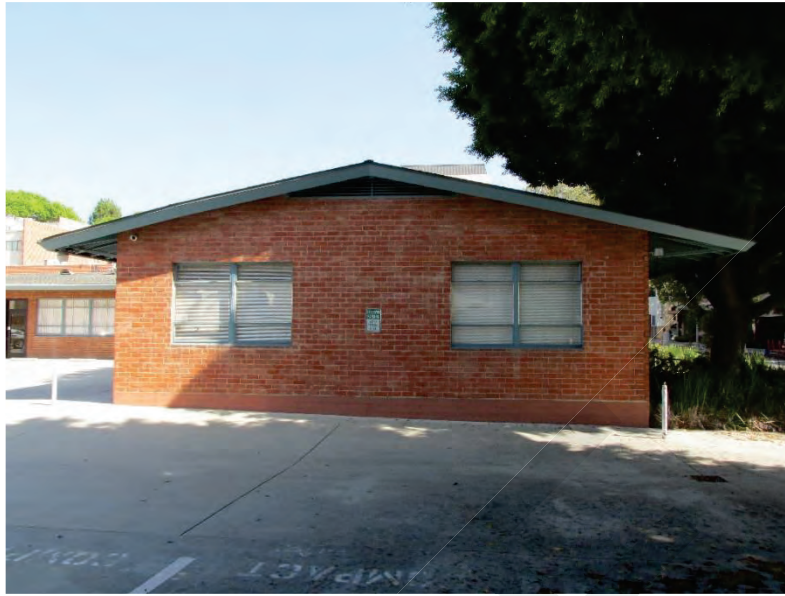
Figure 17. Building 4: South Elevation, View looking north (IMG_8534)
