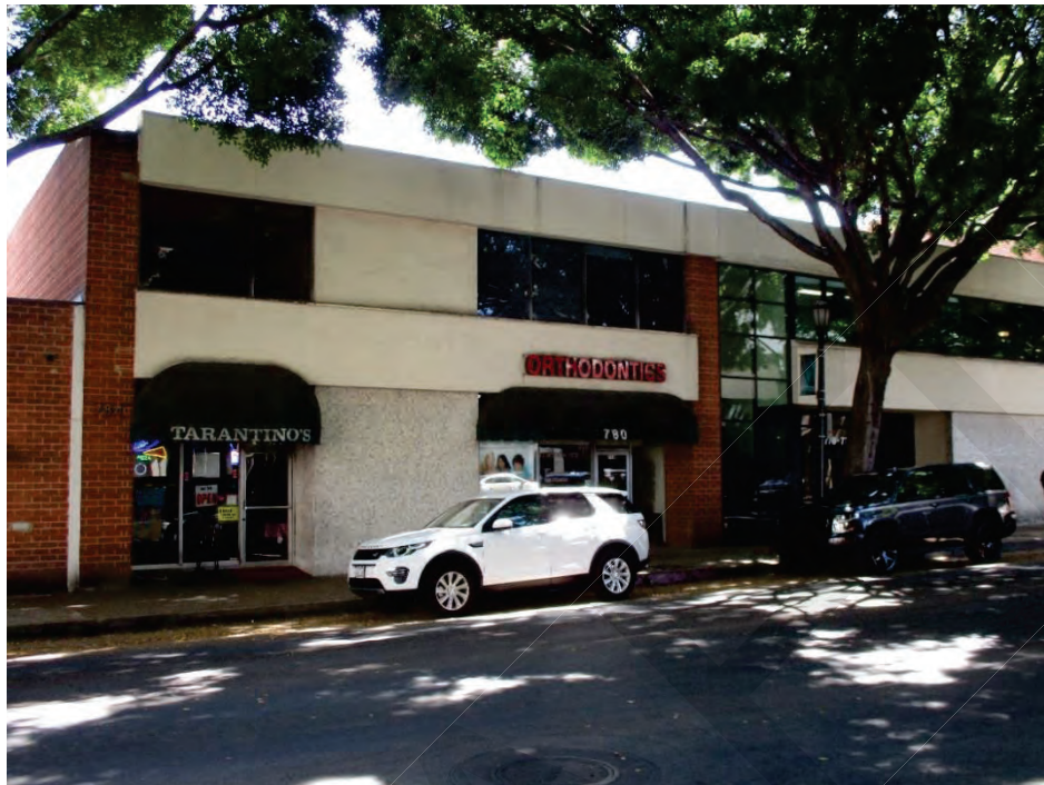
Figure 8. Building 2: Left section of North Elevation, View looking southwest (IMG_0489)
