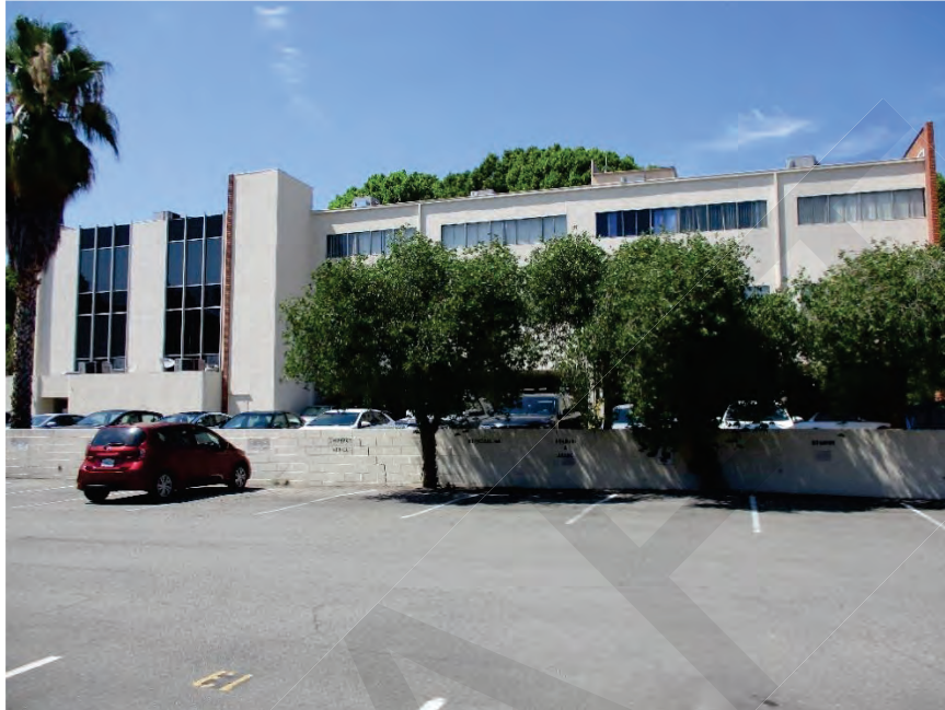
Figure 3. Building 1: South Elevation, View looking north (IMG_0414)
