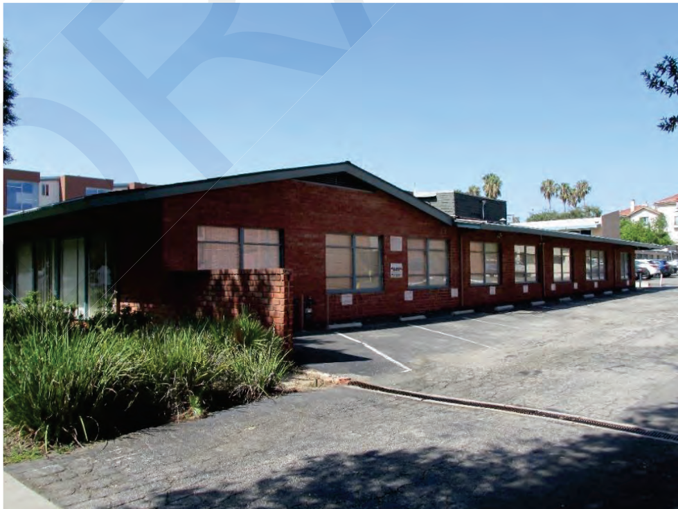
Figure 2. Building 4: North Elevation, View looking southwest (IMG_8521)
