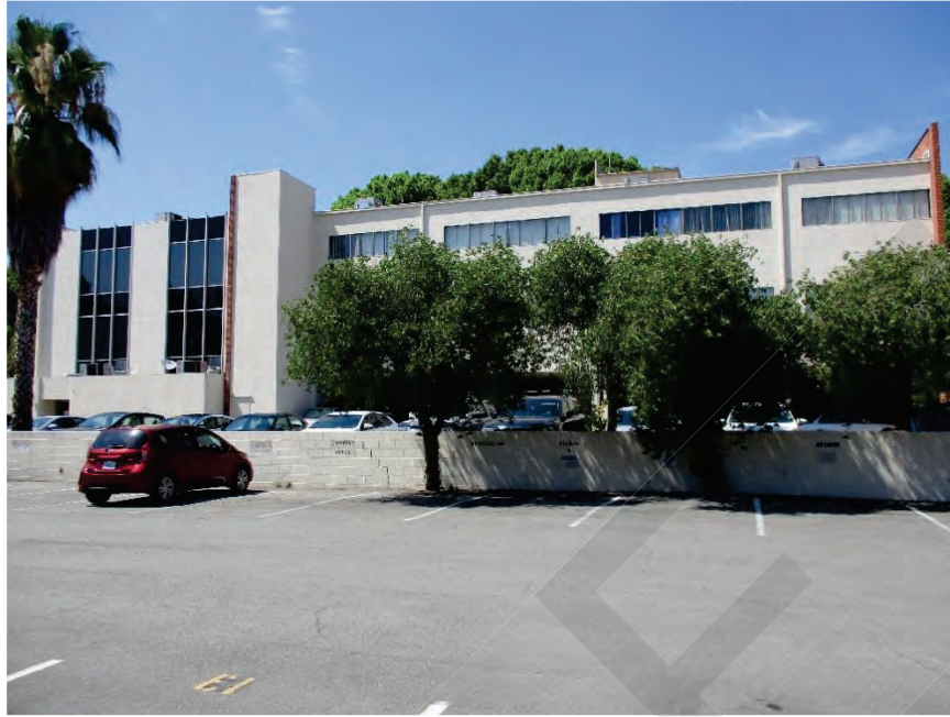
Figure 7. Building 1: South Elevation, View looking north (IMG_0414)
