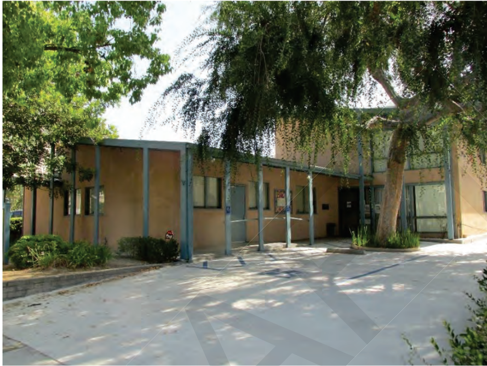
Figure 1. Building 5: West Elevation, View looking northeast (IMG_8491)
