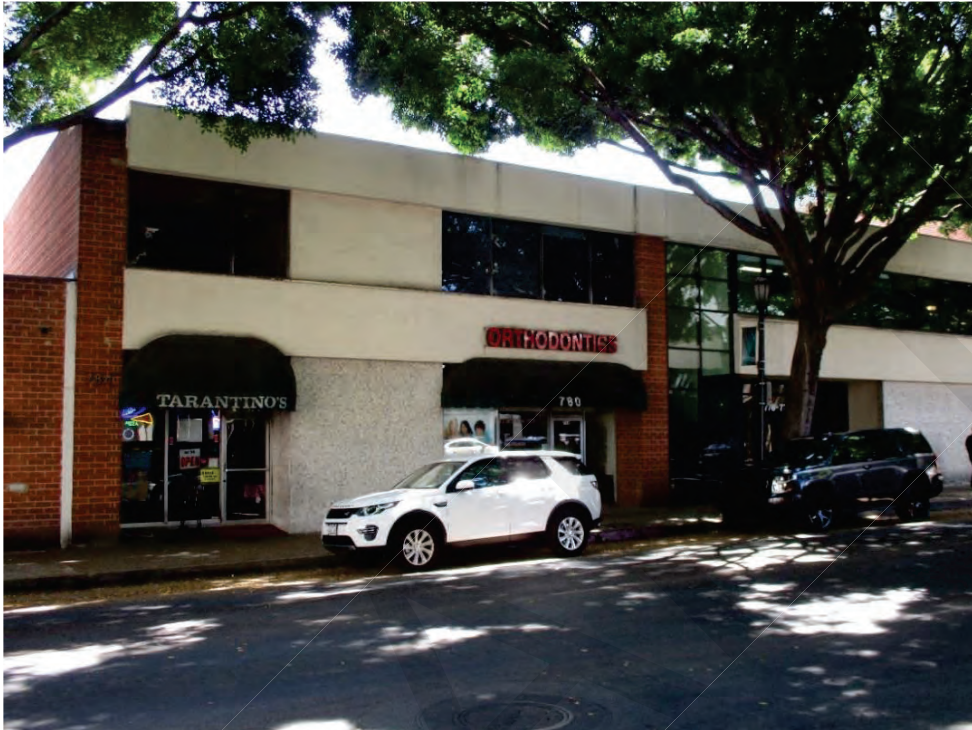
Figure 1. Building 2: Left section of North Elevation, View looking southwest (IMG_0489)
