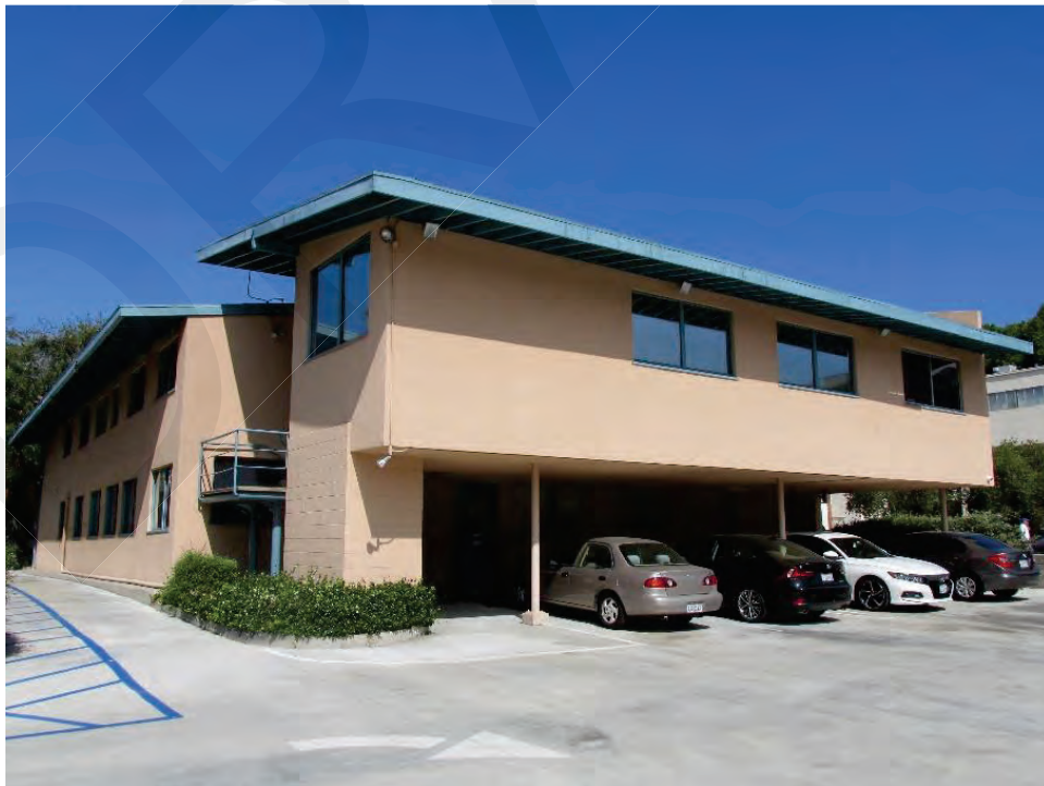
Figure 2. Building 5: South and East Elevations, View looking northwest (IMG_8497)
