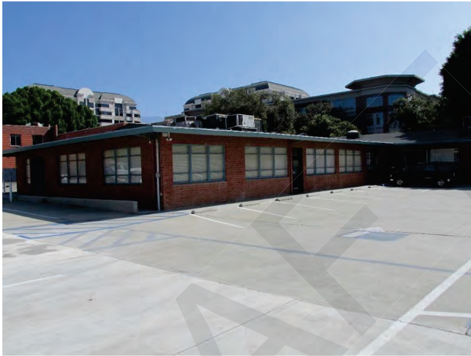
Figure 3. Building 4: West and South Elevations, View looking northeast (IMG_8541)
