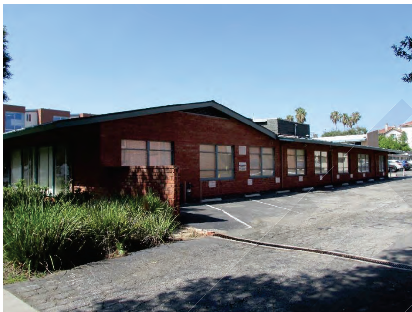
Figure 15. Building 4: North Elevation, View looking southwest (IMG_8521)
