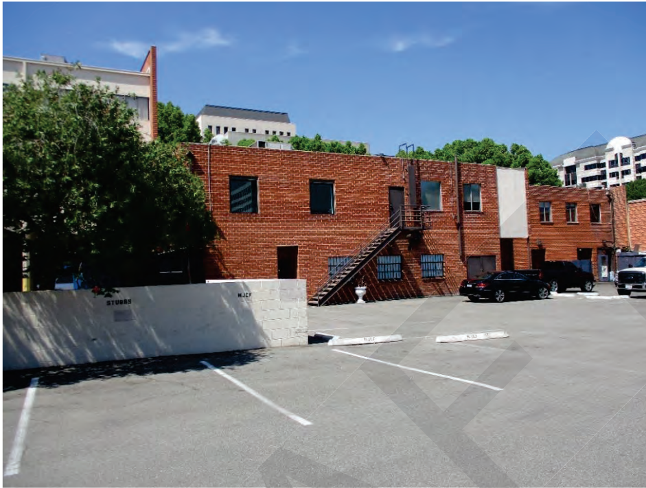
Figure 10. Building 2: South Elevation, View looking northeast (IMG_0455)
