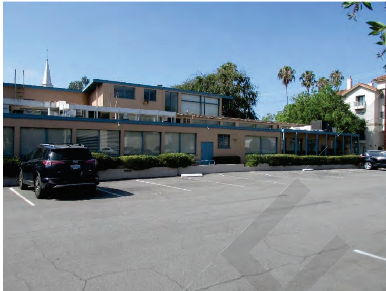
Figure 20. Building 5: North Elevation, View looking southwest (IMG_8506)
