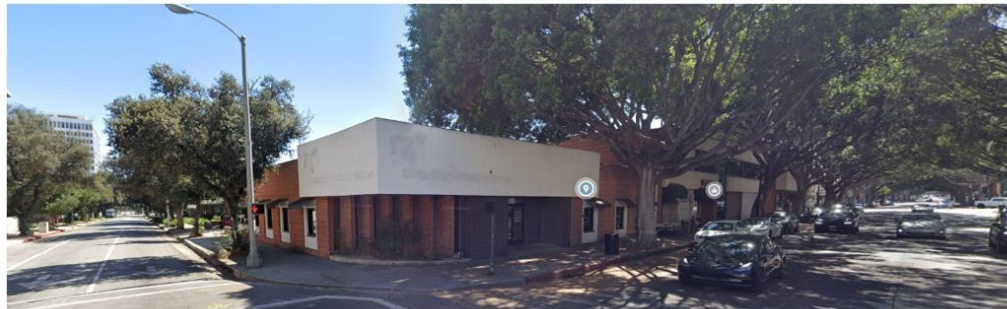
SW view from E. Green St. & S. Hudson Ave.
