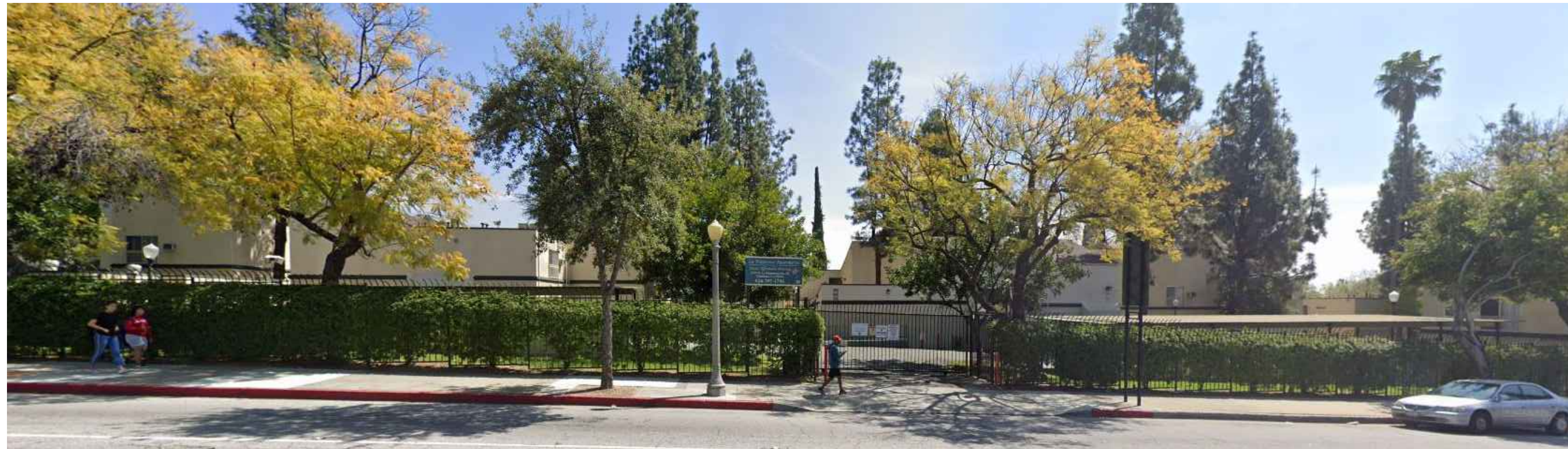
NORTH PARKING ENTRANCE TO PINTORESCA APARTMENTS OFF OF NORTH FAIR OAKS AVE.
