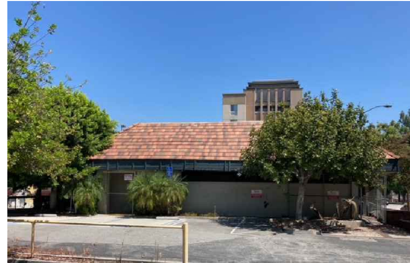
west elevation of existing building (to be removed)
