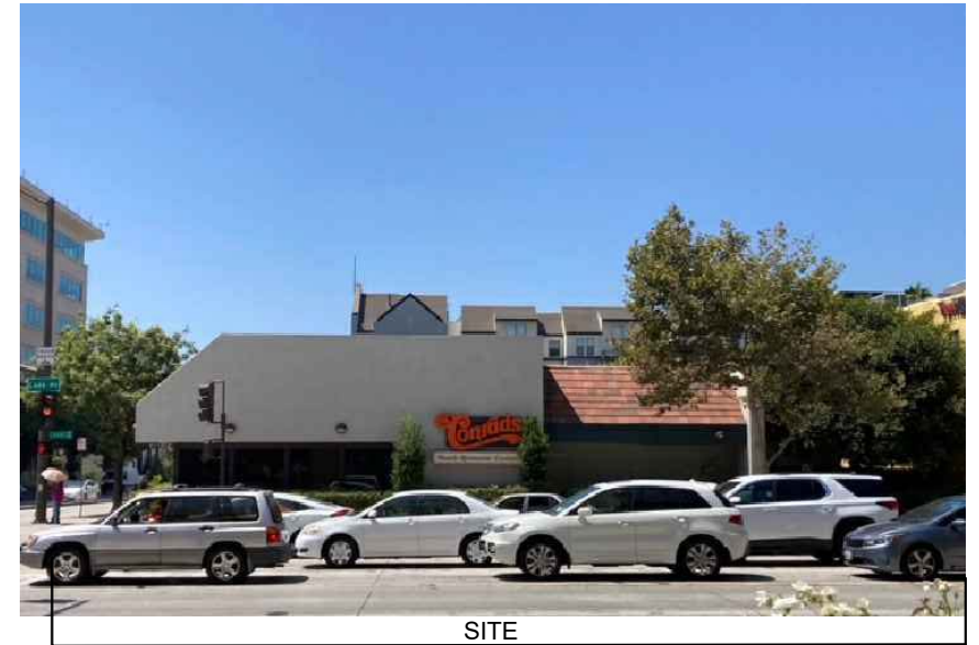
N LAKE AVE. east elevation of existing building (to be removed)
