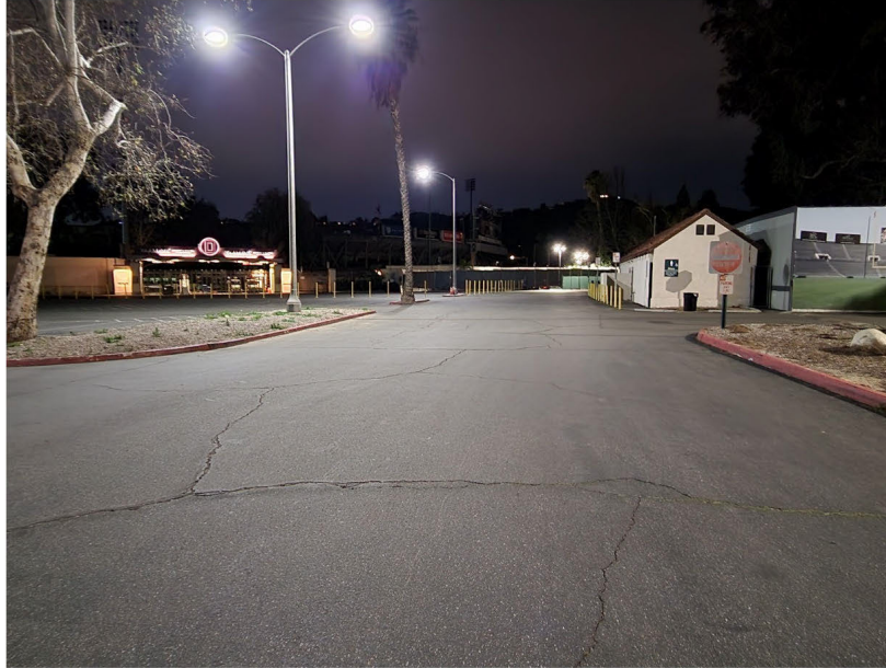
Parking lot access road
