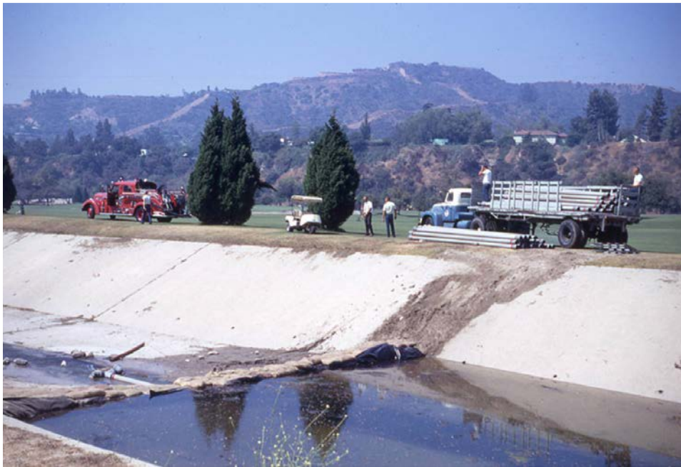
Renovation of Arroyo Seco Channel block, 1967.
