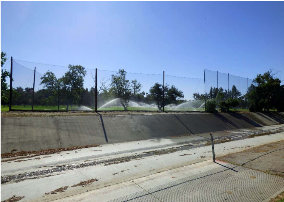
View of rear of driving range from across Arroyo Seco Channel looking southeast. Historic Resources Group, 2021.
