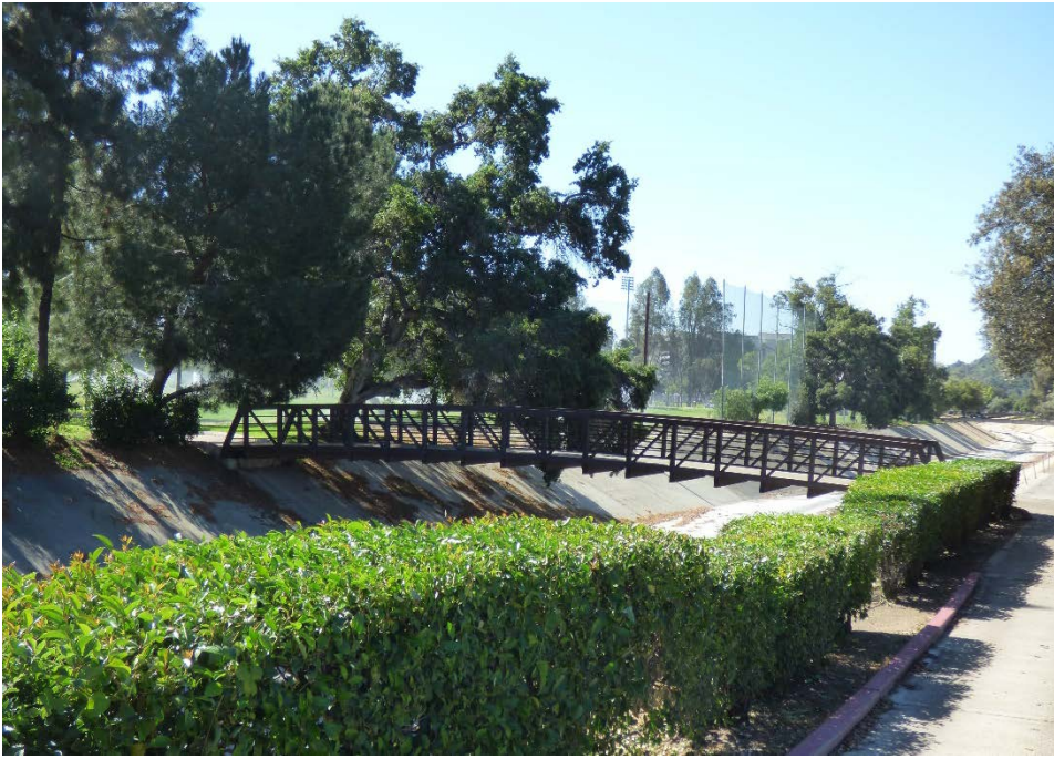
View of Arroyo Seco Channel and wood cross bridge with driving range in background looking northeast. Historic Resources Group, 2021.
