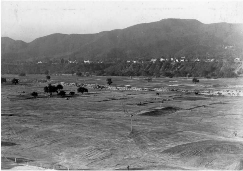
Overview of the new course being built looking southwest, c. 1940
