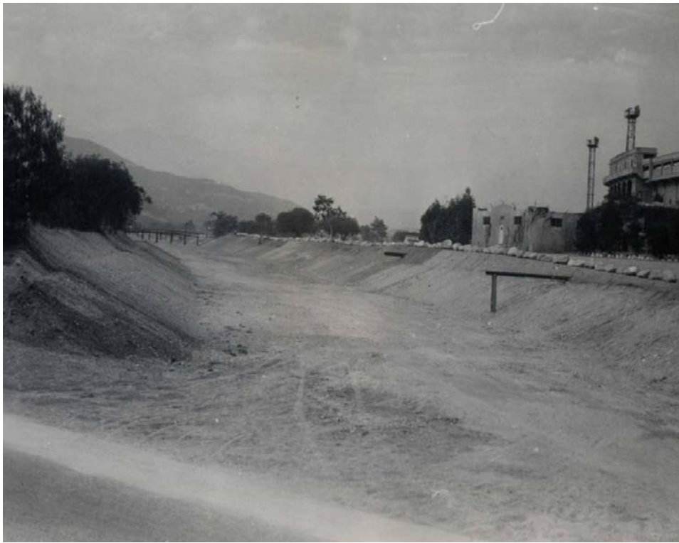
Construction of Arroyo Seco Channel near Rose Bowl, 1934.
