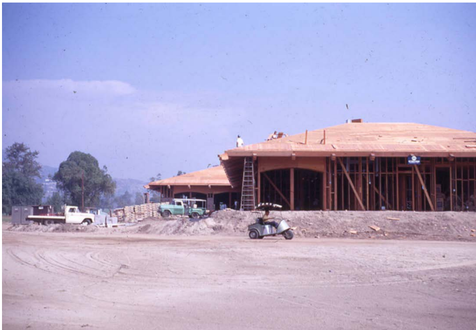
Construction of new clubhouse looking north, 1967.
