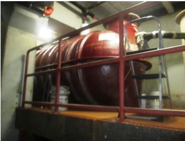
Grease trap in parking garage of 441-483 Building (Whole Foods)
