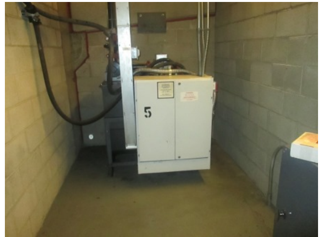
Hydraulic elevator equipment in parking garage
