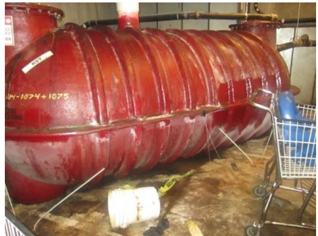
Grease trap in parking garage of 441-483 Building (Whole Foods) Grease trap in parking garage of 441-483 Building (Whole Foods)
