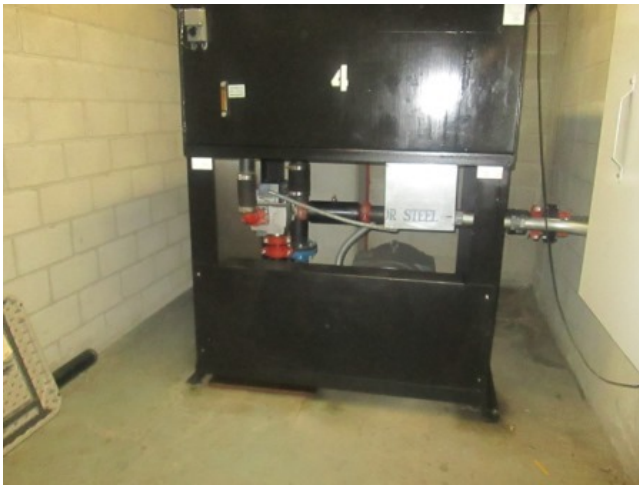
Hydraulic elevator equipment in parking garage
