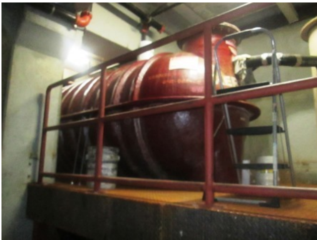
Grease trap in parking garage of 441-483 Building (Whole Foods) Grease trap in parking garage of 441-483 Building (Whole Foods)
