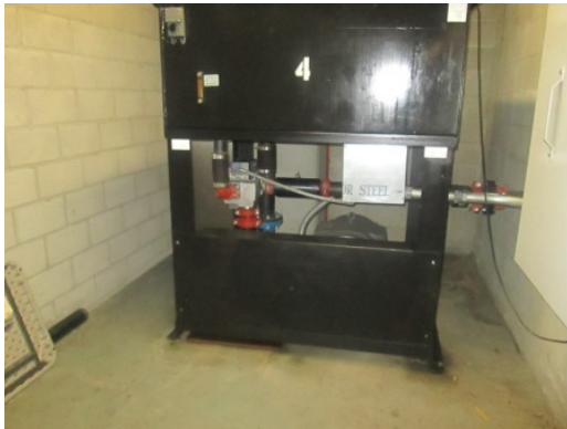
#55 HYDRAULIC ELEVATOR EQUIPMENT IN PARKING GARAGE
