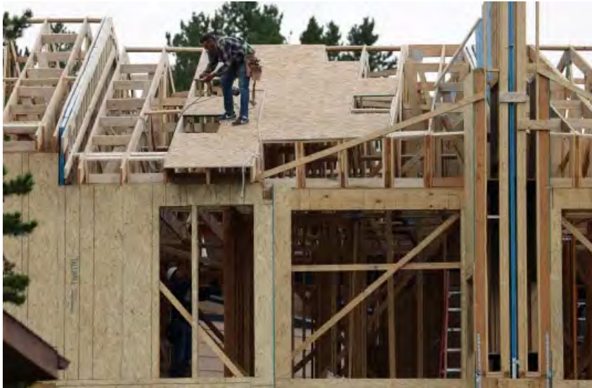
Pasadena continues to experience significant new housing construction.
