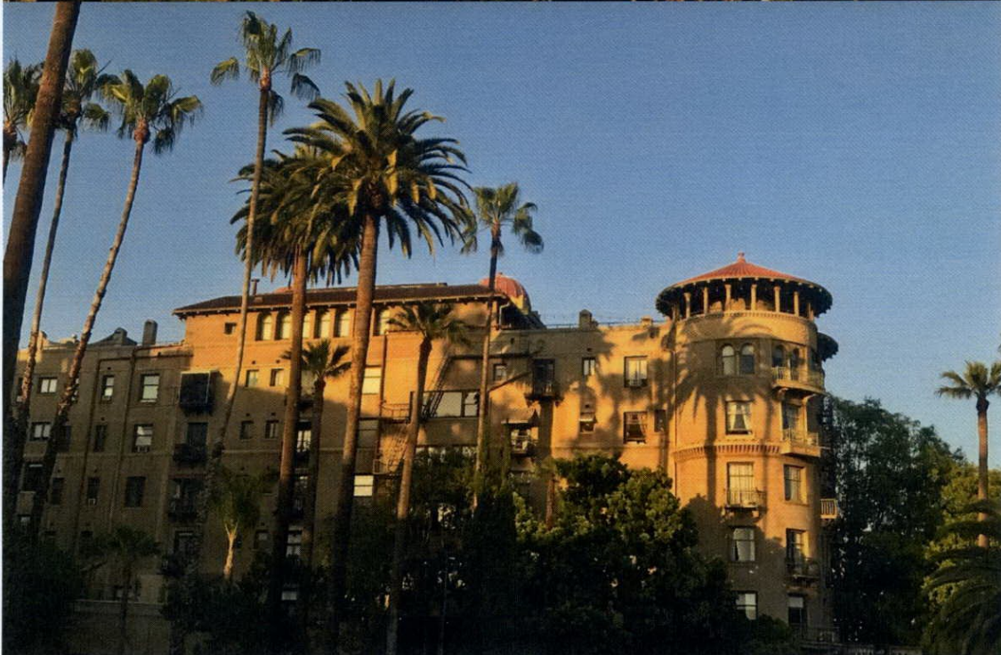
This current 124-year-old-view from Fair Oaks of The Castle Green with its iconic turrets will be blocked out
