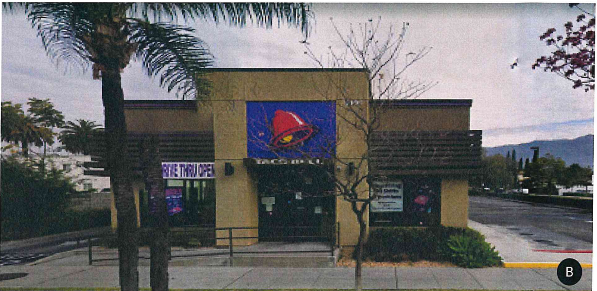
1953 E Colorado Blvd South Facade
