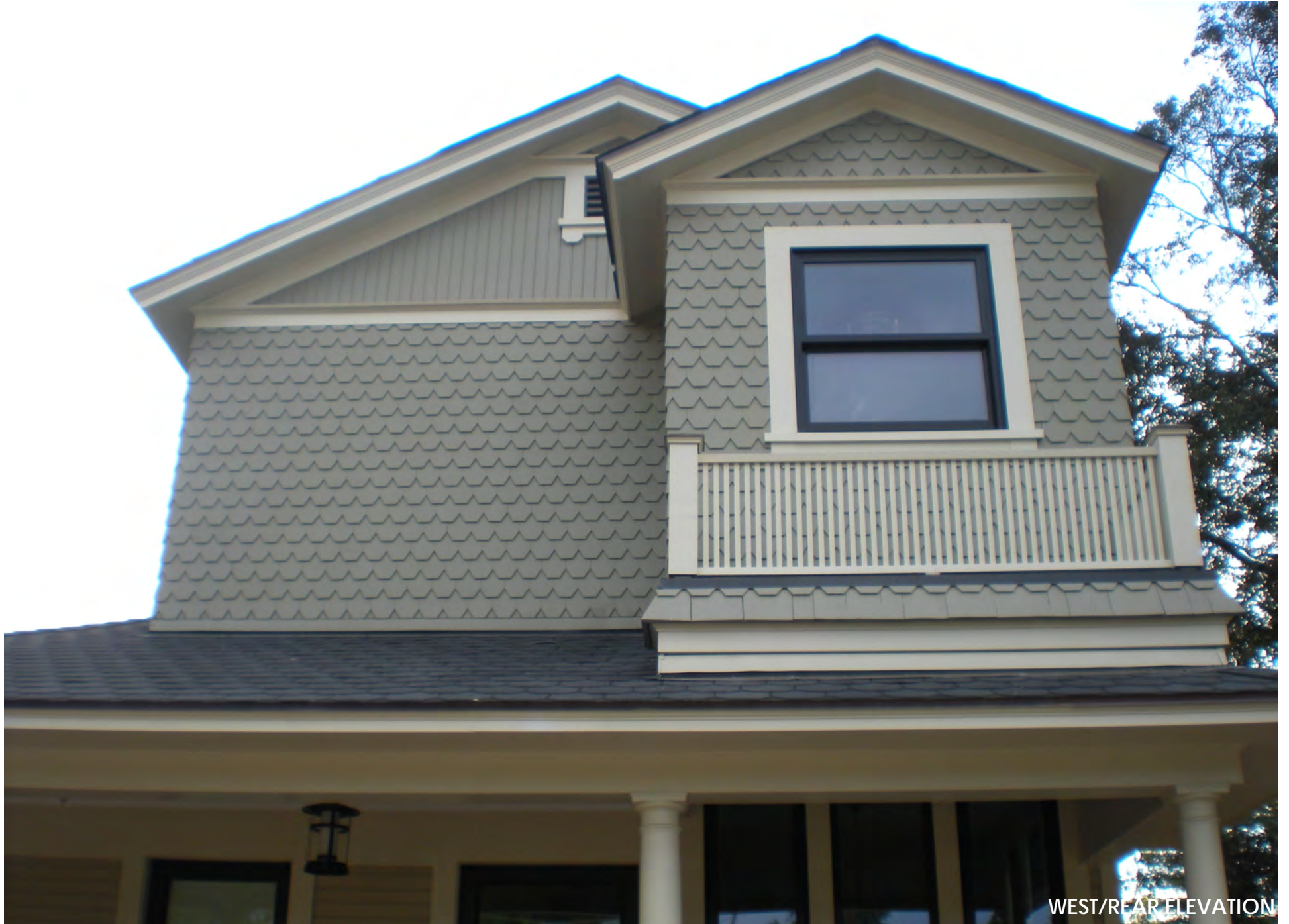
673 South Los Robles Avenue | James L. Lee Residence
