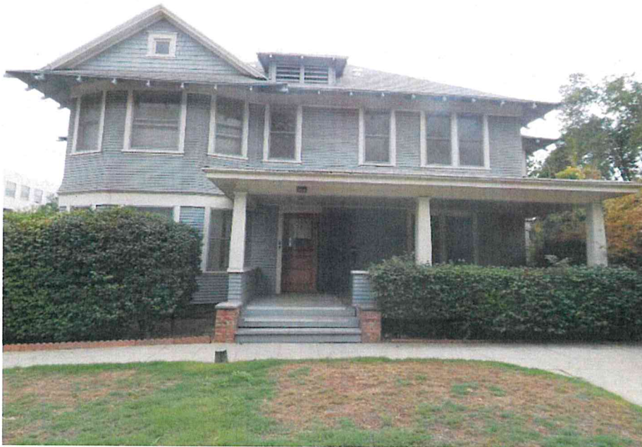
Figure 5. Front (north) façade of 164 Chestnut Street with hipped roof, two-story bay topped with gabled roof, and partial-width porch. View looking south.
