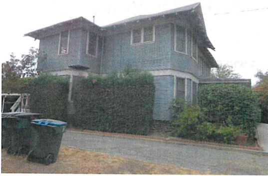
Figure 10: East façade of 164 Chestnut Street along driveway. View facing southwest.
