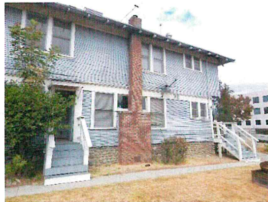
Figure 14: Living room entrance, kitchen entrance, and rebuilt chimney. Looking northeast.
