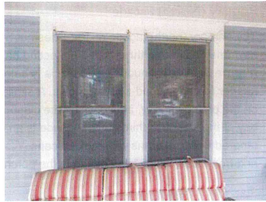
Figure 7: Typical double-hung wood windows with wood screens at the porch.
