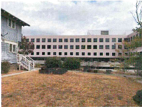
Figure 23: Rear yard, looking east to Gold Line tracks and back of building on Marengo Avenue.
