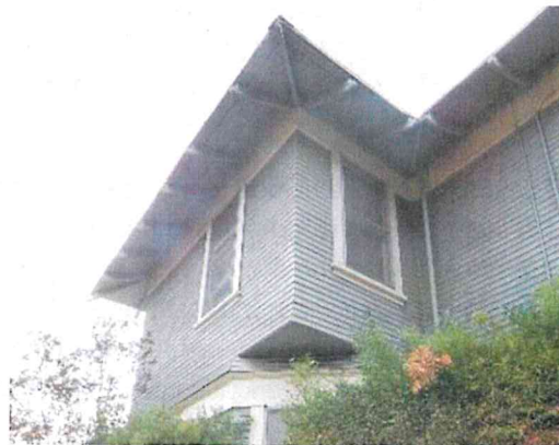
Figure 11: Projecting bay at east facade with clipped corners, looking southwest
