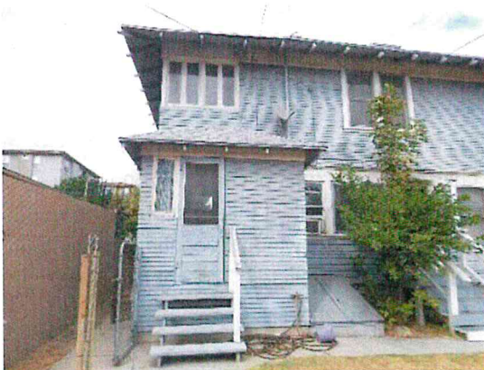
Figure 13: Sunroom addition and enclosed porch at the second-story. Looking north.
