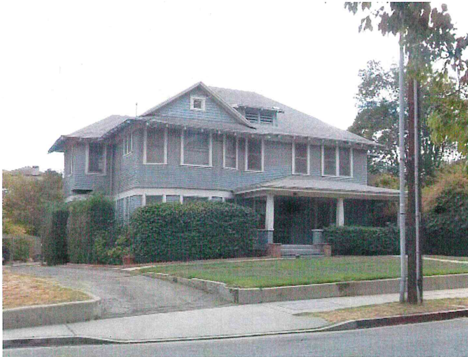
Figure 4. The front (north) façade of 164 Chestnut Street, looking southwest.
