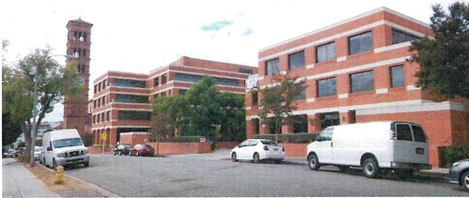
Figure 29. The International Union of Operating Engineers building, with St. Andrew's Church bell tower in the background, at the corner of Raymond Avenue and Chestnut Street, looking northwest.
