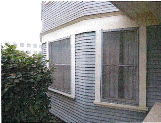
Figure 6: Typical double-hung wood windows with wood board or fascia as header.
