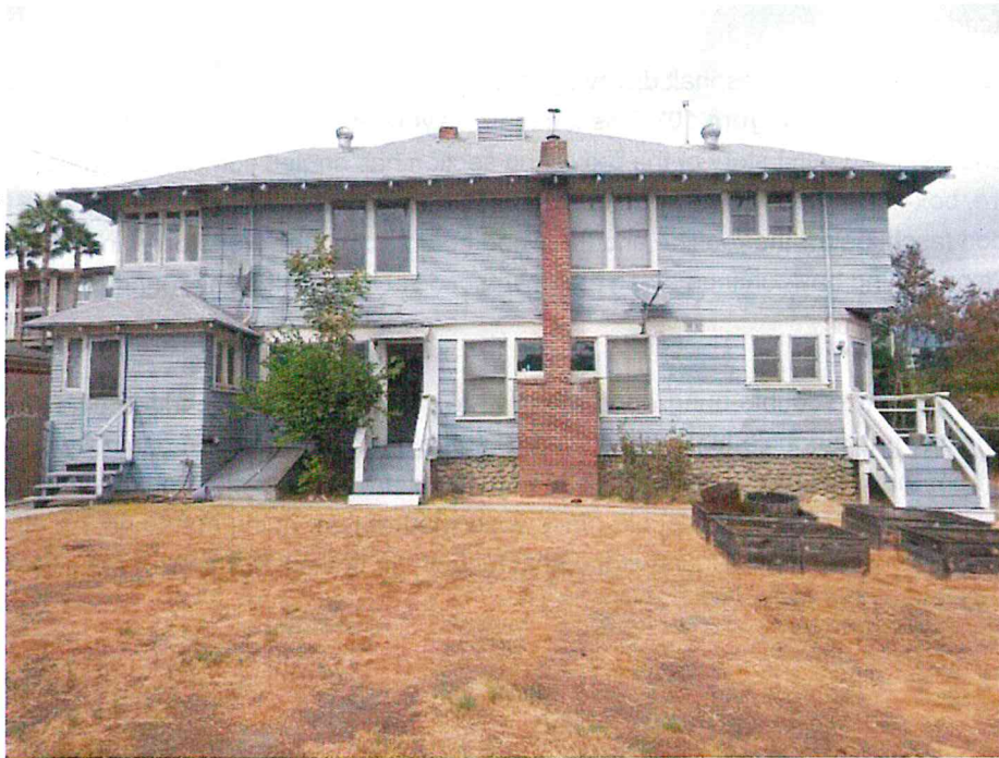
Figure 12: South (rear) facade of 164 Chestnut Street. View facing north.
