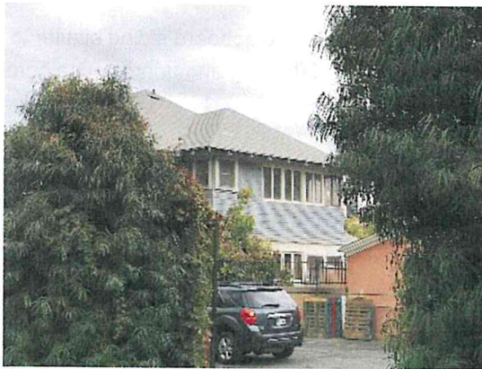
Figure 15: Partial west façade with the projecting, enclosed porch. View looking southeast.
