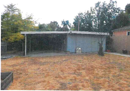
Figure 19: Wood-framed garage that now serves as storage and attached carport. Looking south.
