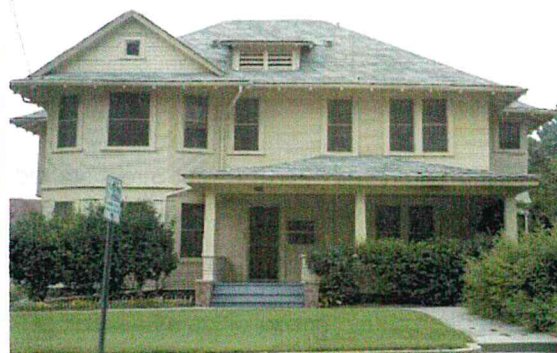
Figure 46: Detailed view of front facade of 164 Chestnut, 1978. Source: City of Pasadena.
