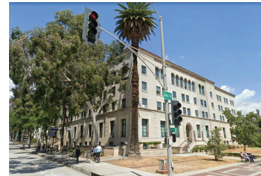
YMCA CENTENNIAL PLACE CORNER OF HOLLY + MARENGO
