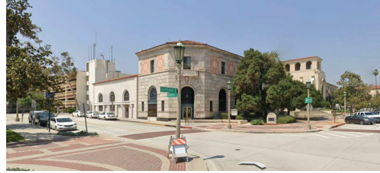
GEORGE ELLERY HALE BUILDING VIEW FROM CORNER OF GARFIELD + HOLLY
