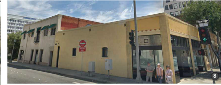
238 UNION & 48 MARENGO AVE
