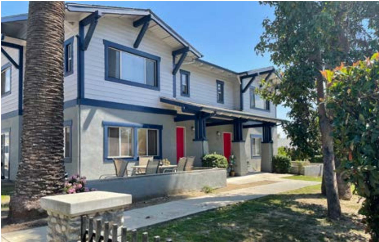
New multi-family housing at the corner of Lincoln Ave. and Idaho St.
