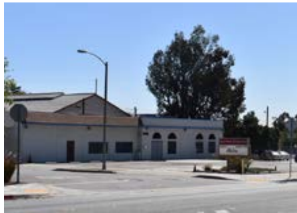
Church with large surface parking lot along Lincoln Ave. at Claremont St.
