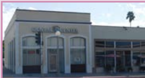
Dental Center building at 2030 Lincoln Ave.
