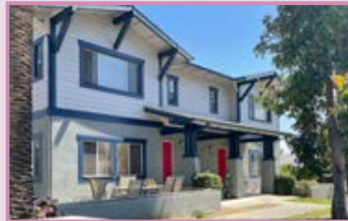
Multifamily residential on Lincoln Ave. between Idaho St. and the I-210 Freeway
