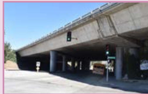
I-210 Freeway over Lincoln Ave. at Howard St.
