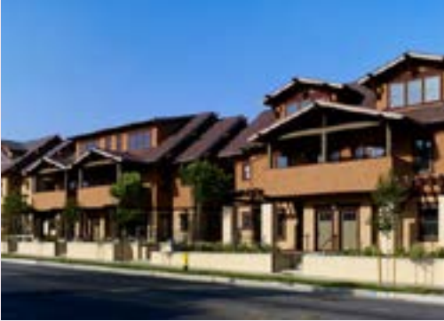
Example of approximately 36' building
