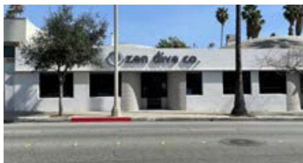
Office use in traditional storefront with inactive frontage
