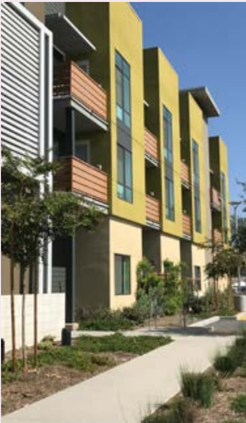
Example of approximately 39' building
