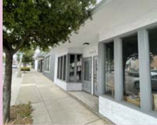
Commercial building on Lincoln Avenue with recessed entrance and transparency
