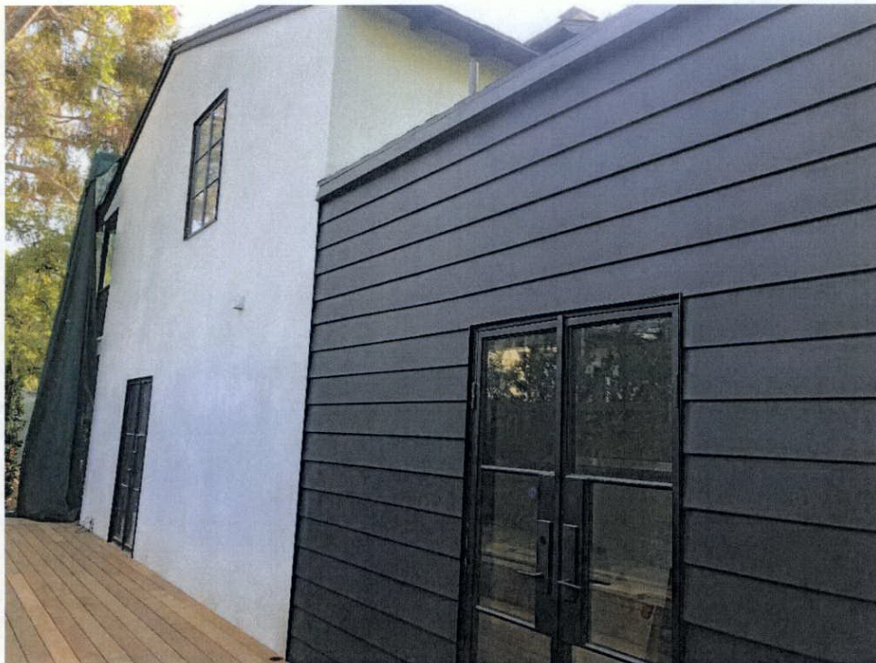
Figure 7. Northwest Façade, 801 S. San Rafael Avenue (view northeast) SOURCE: Sapphos Environmental, Inc., 2021
