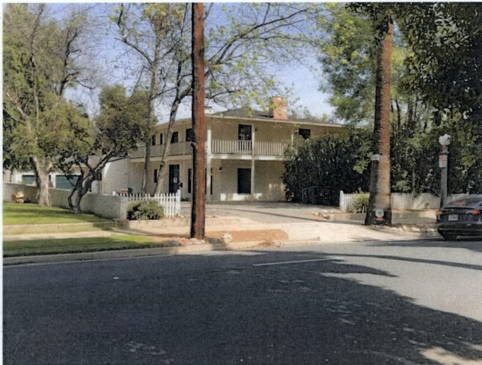
Figure 12. The McCarthy House, 762 St. John Street SOURCE: Sapphos Environmental, Inc., 2021
