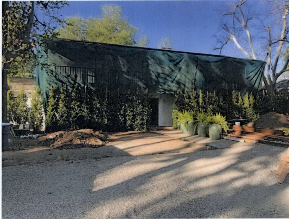
Figure 2. 801 S. San Rafael Avenue (view southwest) SOURCE: Sapphos Environmental, Inc., 2021
