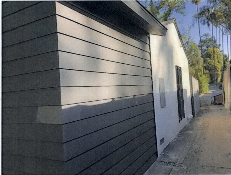
Figure 6. Southeast Façade, 801 S. San Rafael Avenue (view north) SOURCE: Sapphos Environmental, Inc., 2021
