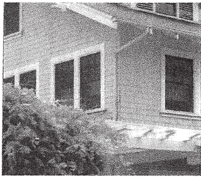
F. Gutter and downspout
