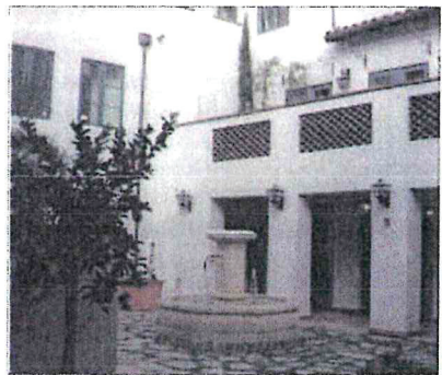
C. Plaster walls with clay tile grilles.
