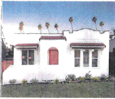
D. Flat roof with parapet and tile cap
