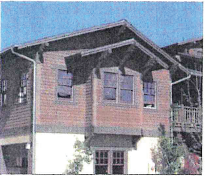
A. Cantilevered bay window
