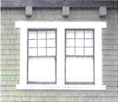
G. Painted openings framed by wide boards
