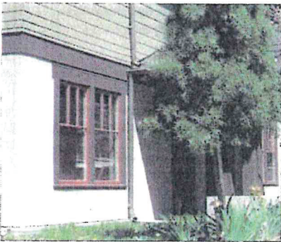
B. Plaster ground floor as base
