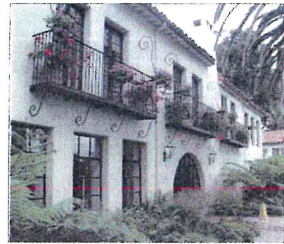
C. Plaster Walls with formal window composition
