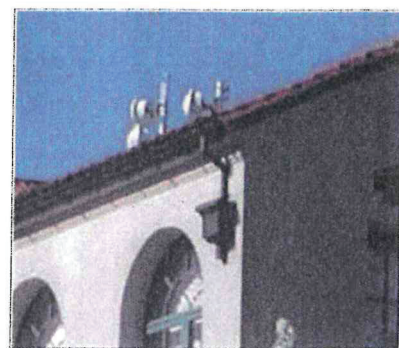
F. Gutter transitions to internal drain pipe
