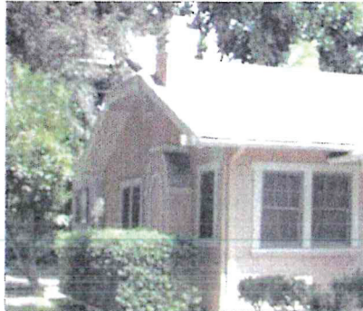
H. Attached chimney
