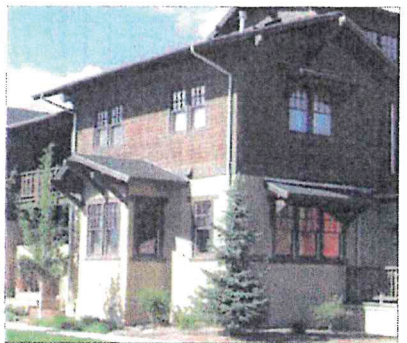
C. Plaster and wood siding
