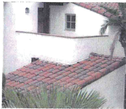
E. Sloped tile roof
