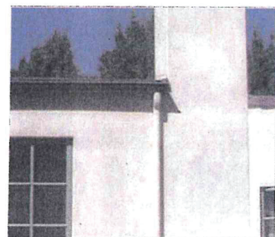
F. Gutter and downspout
