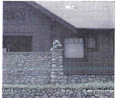
C. Stone base with clapboard siding
