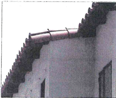
D. Shallow eave with large rafter tails
