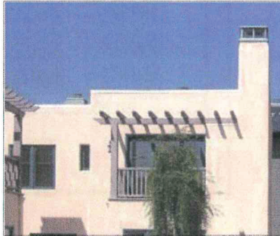
H. Integrated chimney and trellis
