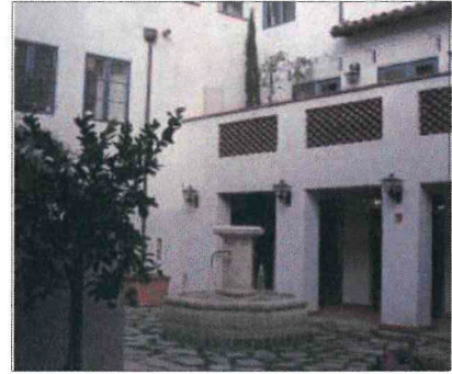
C. Plaster walls with clay tile grilles.
