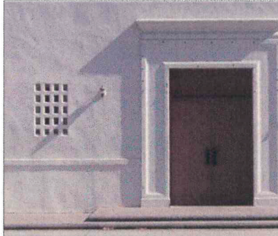
B. Plaster molding articulates base
