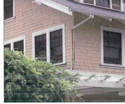
F. Gutter and downspout
