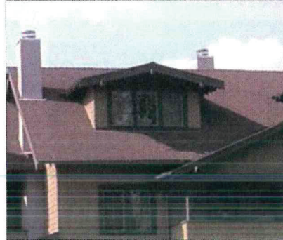
E. Dormer window with pitched roof
