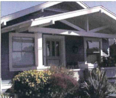
G. Single opening and wide door with lights
