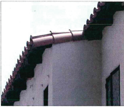
D. Shallow eave with large rafter tails
