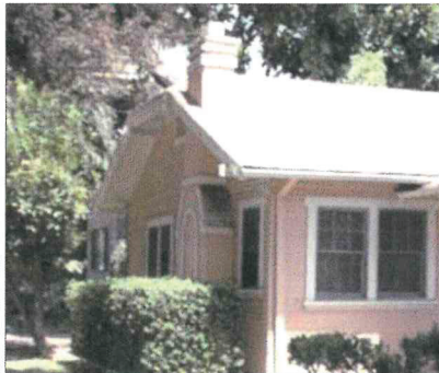
H. Attached chimney
