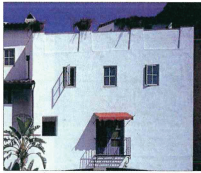
E. Roof as balcony behind articulated parapet
