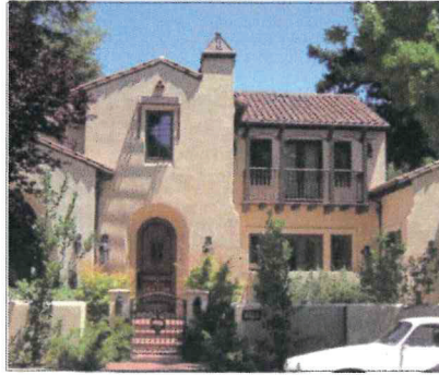
H. Attached balcony and integrated chimney
