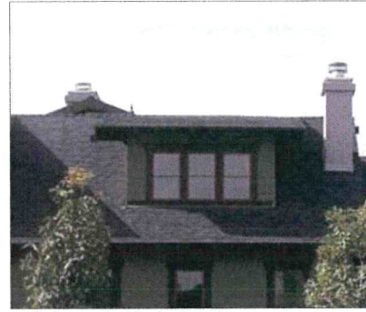
E. Dormer with shed roof
