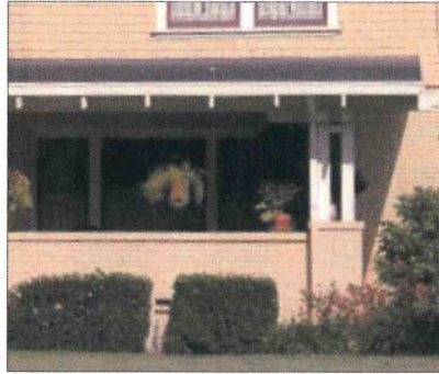
B. Painted brick base
