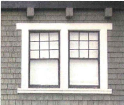
G. Painted openings framed by wide boards
