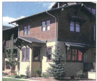
C. Plaster and wood siding
