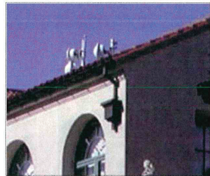
F. Gutter transitions to internal drain pipe
