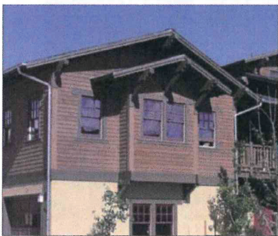
A. Cantilevered bay window
