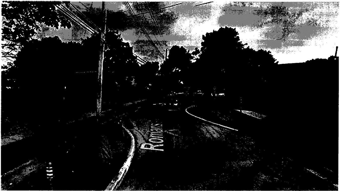
Figure 3.5.4. Chicane Designed to Retain Drainage Features (Source: Google Street View)
