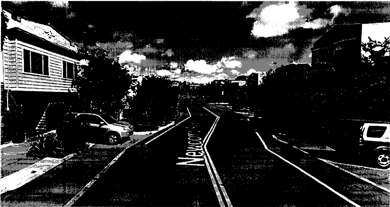
Figure 3.4.3. Midblock Lateral Shift (Source: Google Street View)
