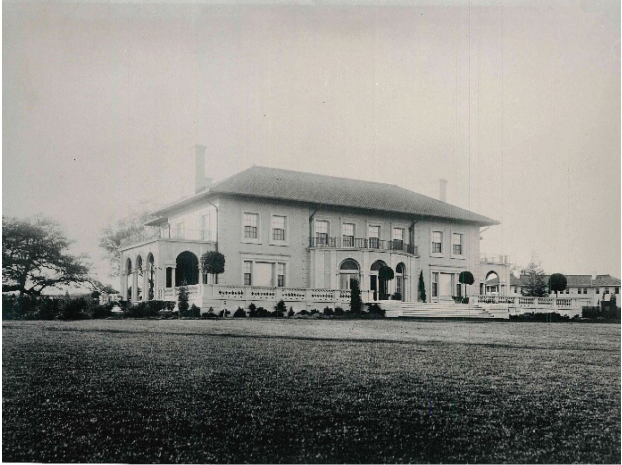
Figure 7: View looking northwest across the lawn toward the rear (east) elevation, circa 1915. Source: Pasadena Museum of History.
