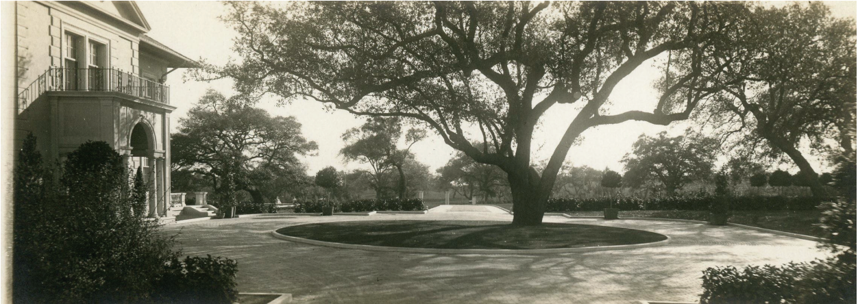
Figure 13: View looking south across the motor court toward the driveway, circa 1920. Once again, the existing pond near the oak tree is not present. The driveway was defined by the same stone curb. There appears to have been two paving materials, a dark material in the center with a lighter material to each side. The existing wrought iron gates are not present. Source: Pasadena Public Library.
