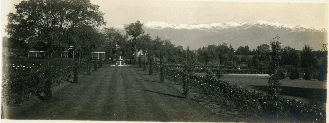
Figure 17: View looking north from the north loggia toward the greenhouse, circa 1920. The fountain at the end of the view is in the portion of the original estate that was subdivided from the property after 1948. The fountain and greenhouse were demolished at an unknown date. Source: Pasadena Public Library.
