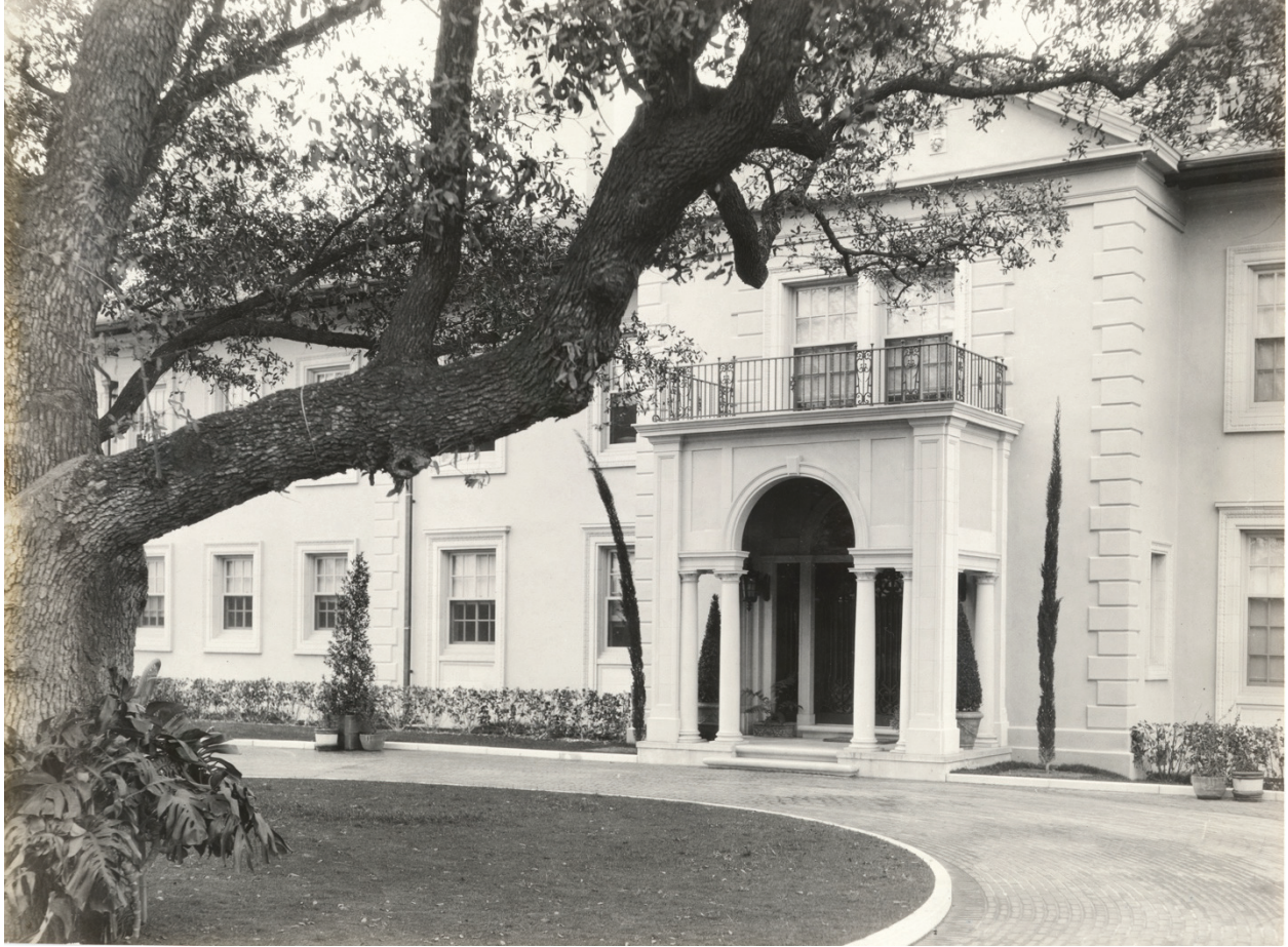
Figure 8: View looking northeast across the motor court toward the facade, 1920. Note the presence of the raised concrete curb and red brick paving. Source: California State Library.
