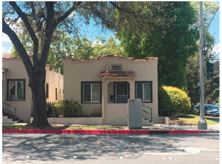
1094 Del Mar North Elevation Looking South
