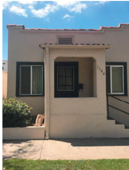
1104 Del Mar North Elevation Looking South
