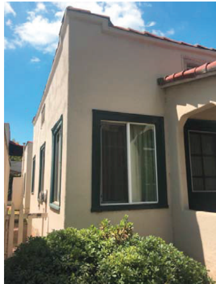
1104 Del Mar East Elevation Looking South
