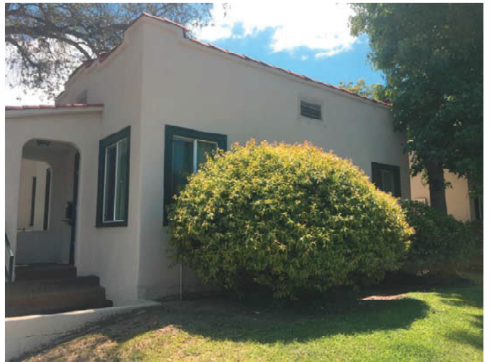
1094 Del Mar West Elevation Looking Southeast
