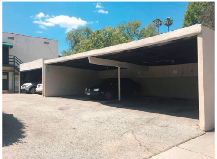
Carport and North Garage South Elevation Looking South
