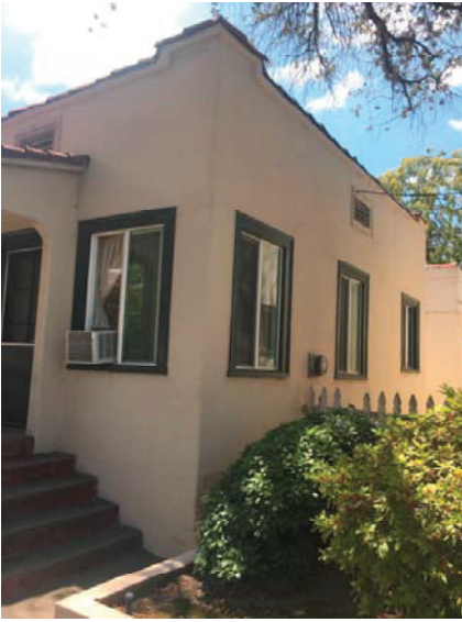
1100 Del Mar West Elevation Looking Southeast 2
