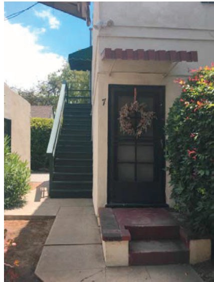
Residence 7 West Elevation Looking East
