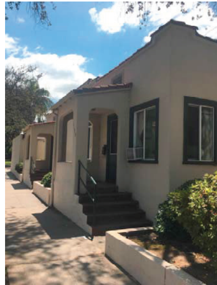
1104 and 1100 Del Mar North Elevation Looking Southeast
