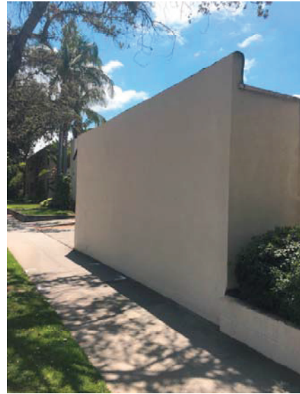
Carport North Elevation Looking East
