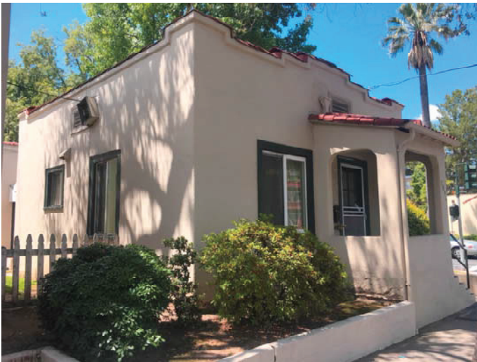
1094 Del Mar North and East Elevation Looking Southwest
