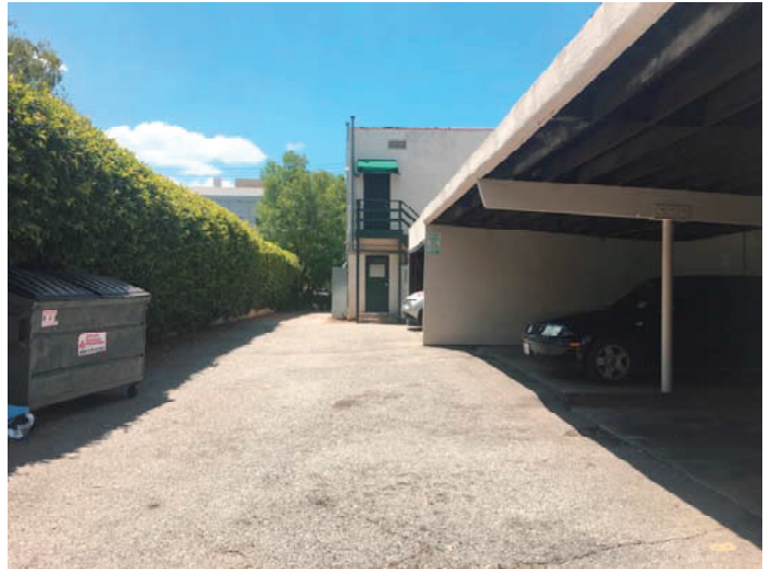
Carport, Residence 7,8 and North Garage Looking South
