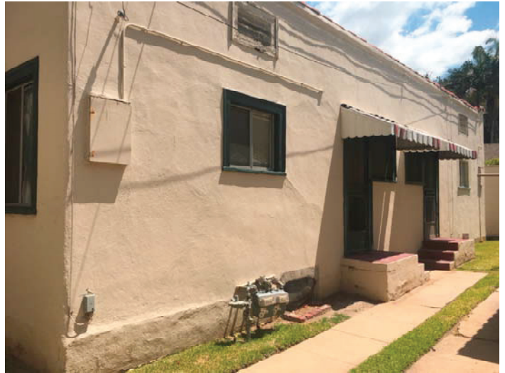
Del Mar Residences South Elevation Looking Northeast
