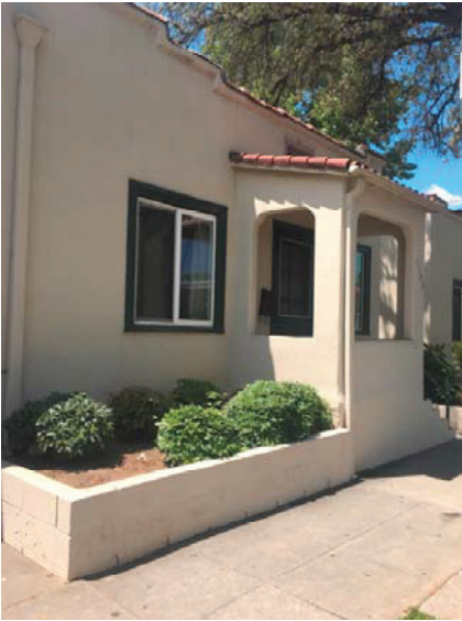
1100 Del Mar North Elevation Looking Southwest
