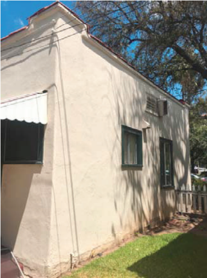
1104 Del Mar East Elevation Looking Northwest
