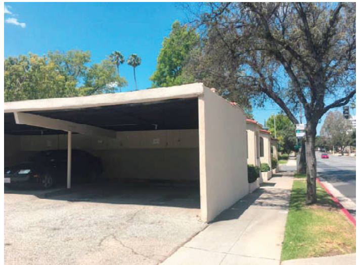
Carport Looking West
