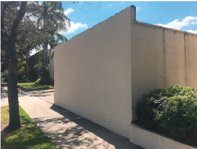
Carport North Elevation Looking East 2
