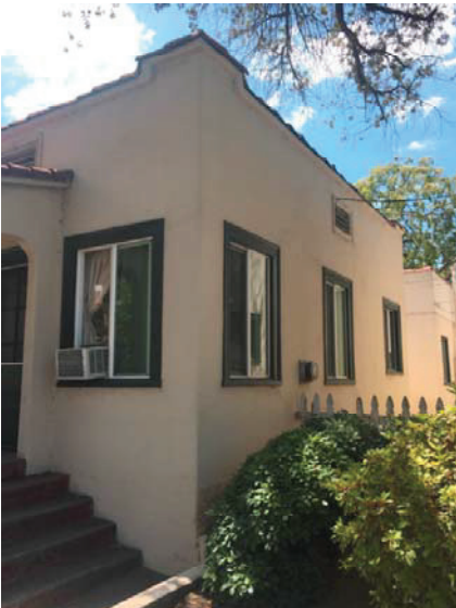
1100 Del Mar West Elevation Looking Southeast 1
