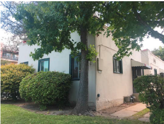
1094 Del Mar West and South Elevations Looking Northeast
