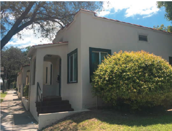
1094 Del Mar West Elevation Looking East 2
