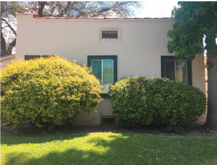
1094 Del Mar West Elevation Looking East 1
