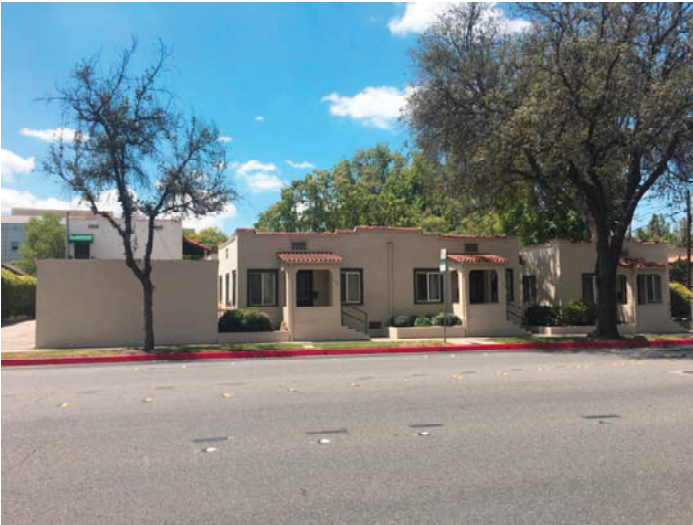
Carport, 1104 and 1100 Del Mar North Elevation Looking
