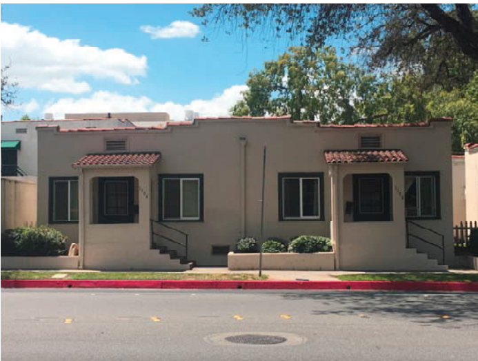
1104 and 1100 Del Mar North Elevation Looking South 1
