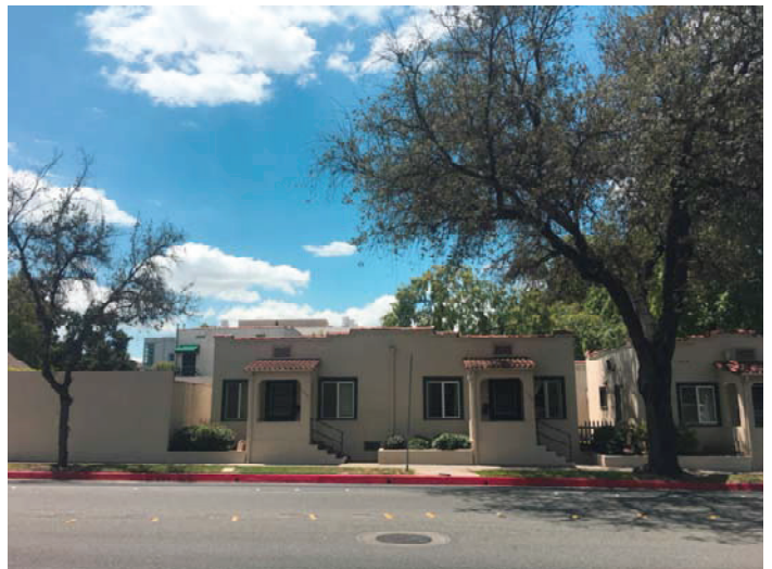
1104 and 1100 Del Mar North Elevation Looking South 2
