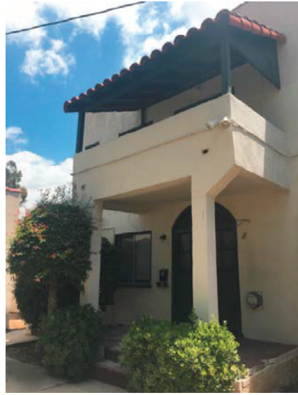
Residence 7,8 West Elevation Looking Northeast
