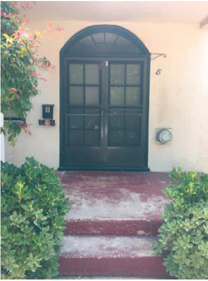
Residence 8 West Elevation Looking East
