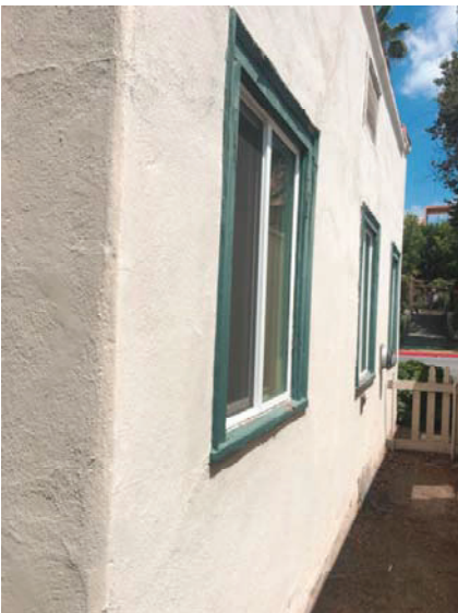
1104 Del Mar East Elevation Looking North
