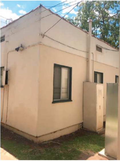
Residence 3 West Elevation Looking Southeast
