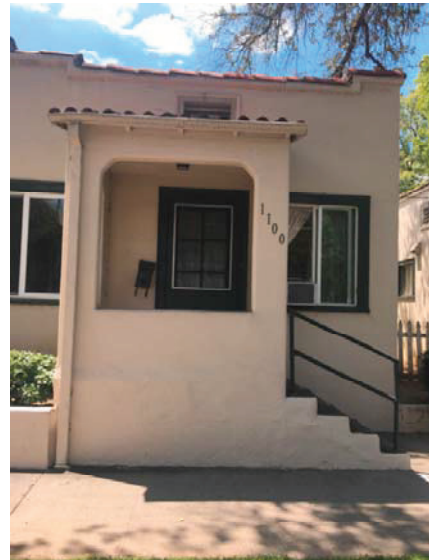
1100 Del Mar North Elevation Looking South
