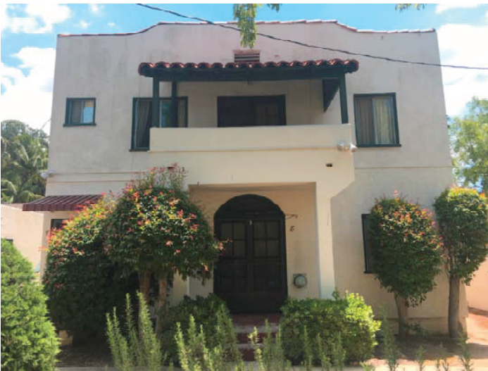
Residence 7,8 West Elevation Looking East
