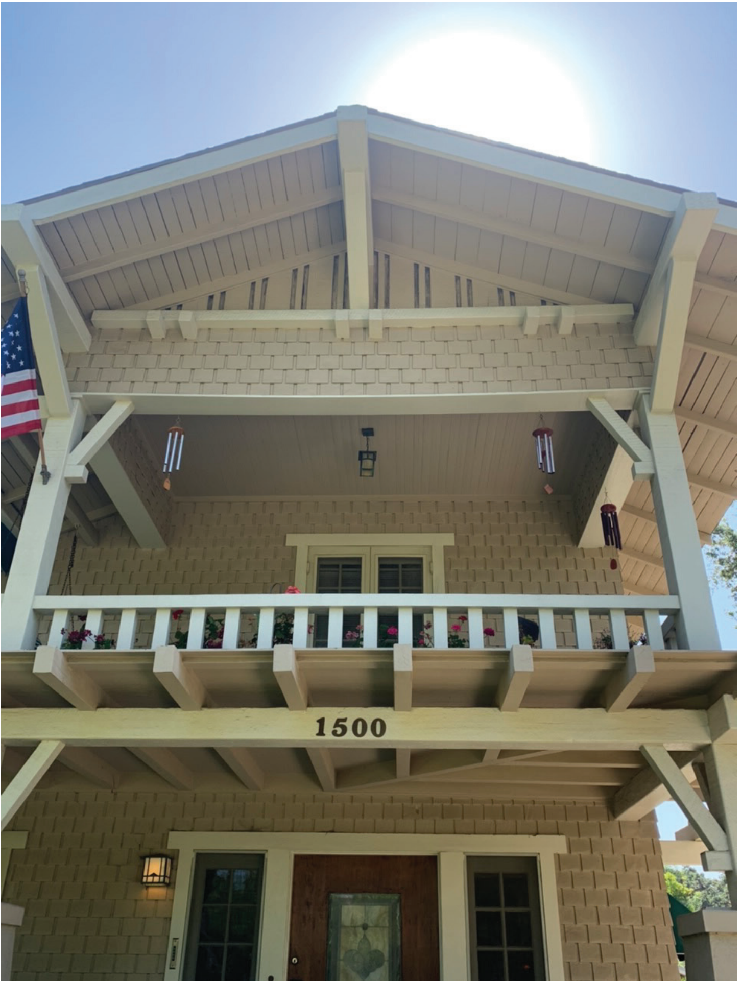
1500 N. LOS ROBLES AVE: UPPER BALCONY, FRONT ELEVATION
