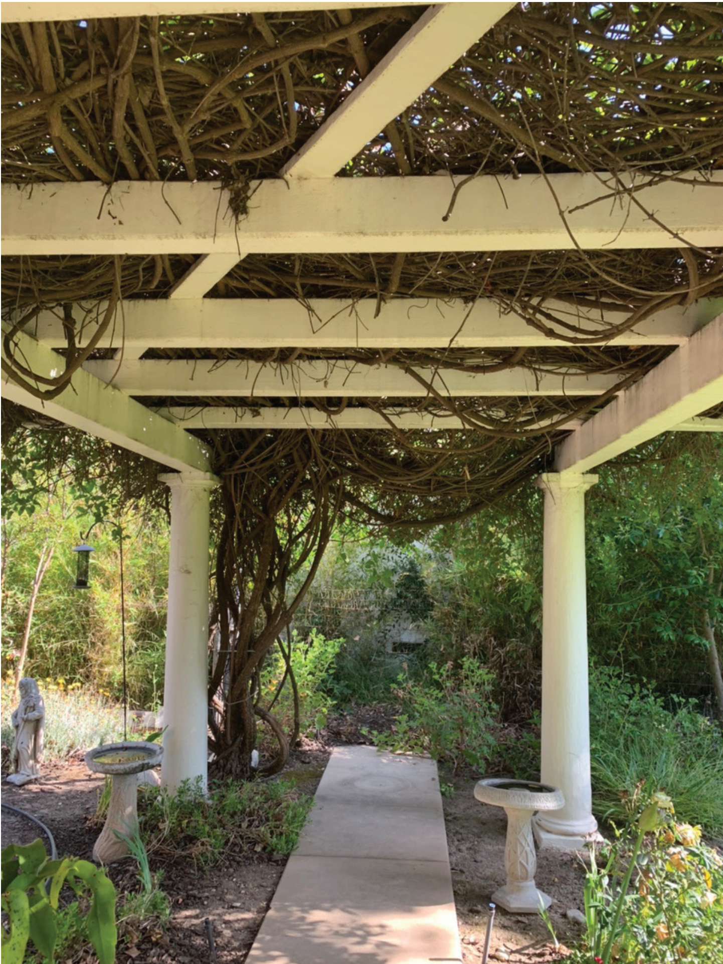
1500 N. LOS ROBLES AVE: REAR YARD PERGOLA AT NORTH END
