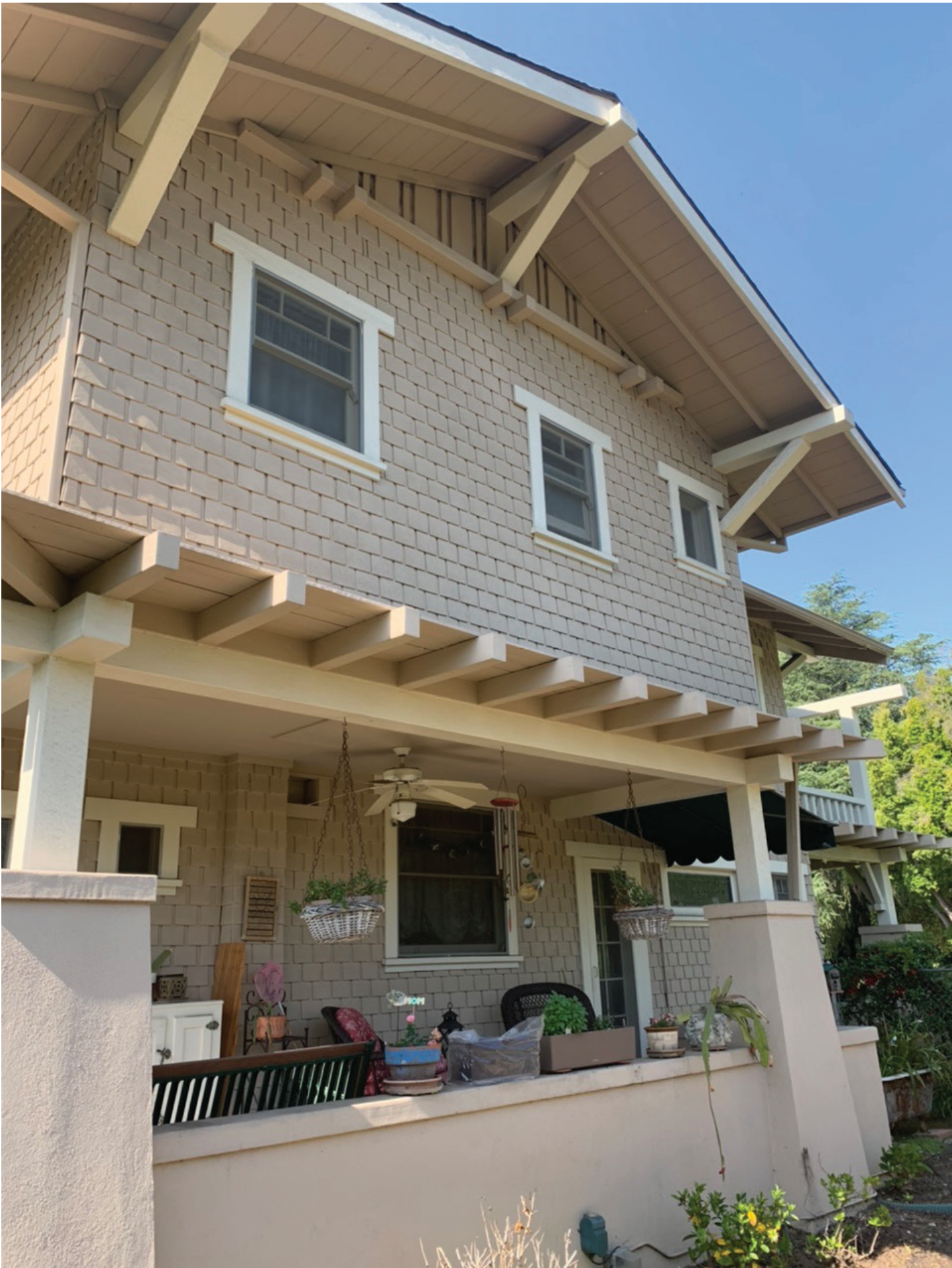
1500 N. LOS ROBLES AVE: NORTH SIDE ELEVATION WITH SIDE PORCH AND UPPER FLOOR ADDITION
