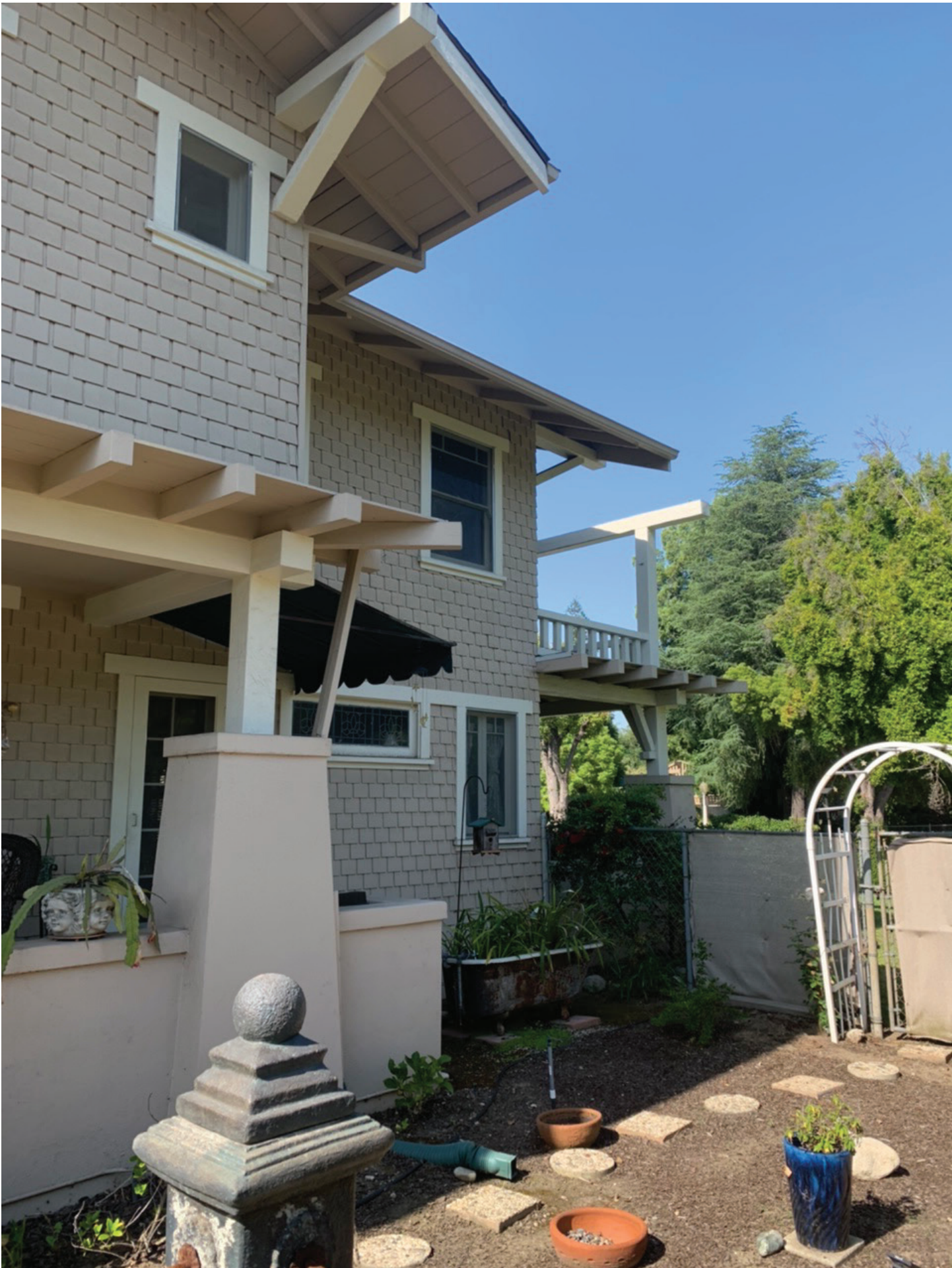
1500 N. LOS ROBLES AVE: NORTH SIDE ELEVATION LOOKING AT FRONT NORTHWEST CORNER OF HOUSE
