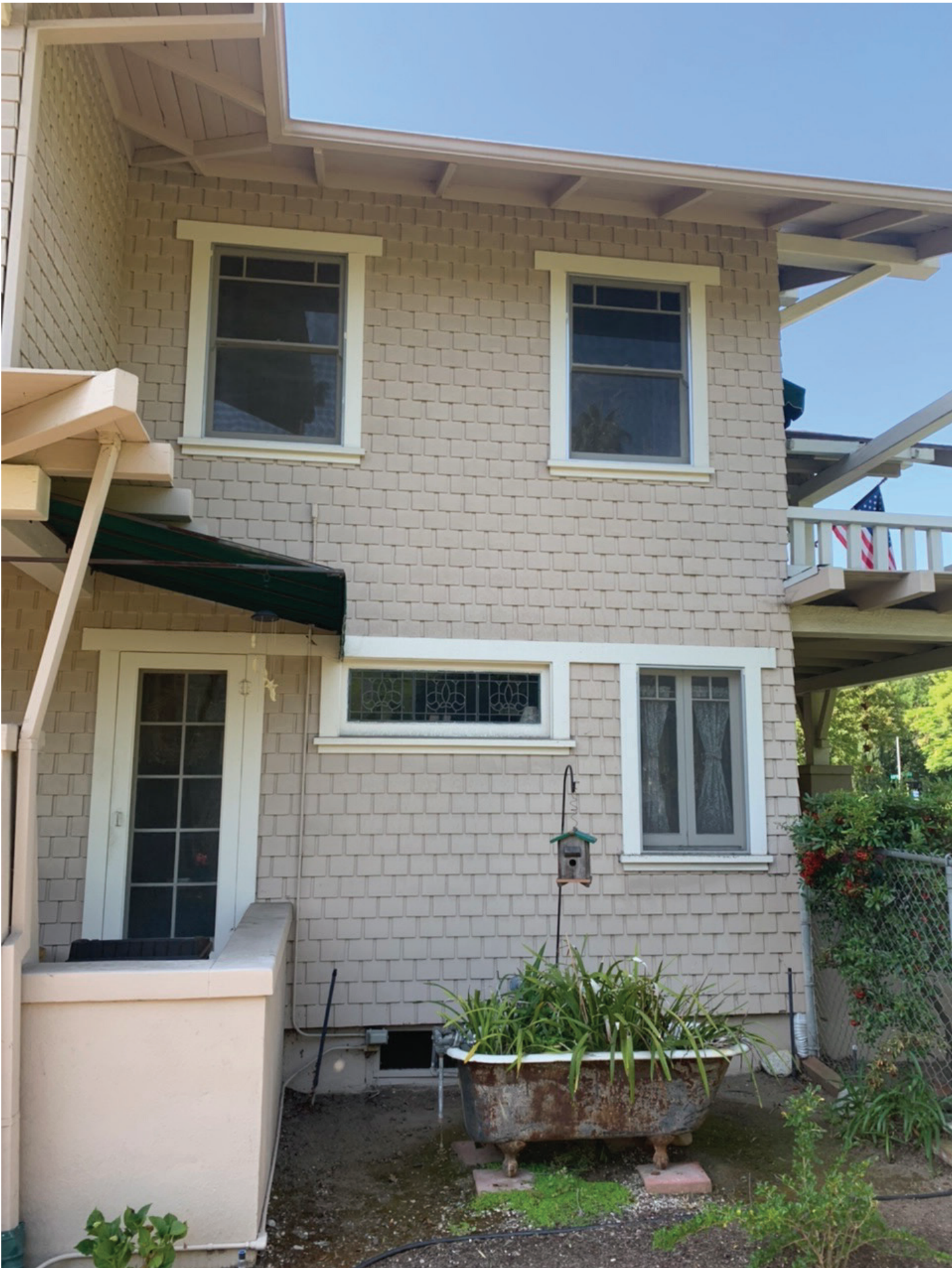
1500 N. LOS ROBLES AVE: REAR ELEVATION LOOKING AT NORTHEAST REAR CORNER OF HOUSE
