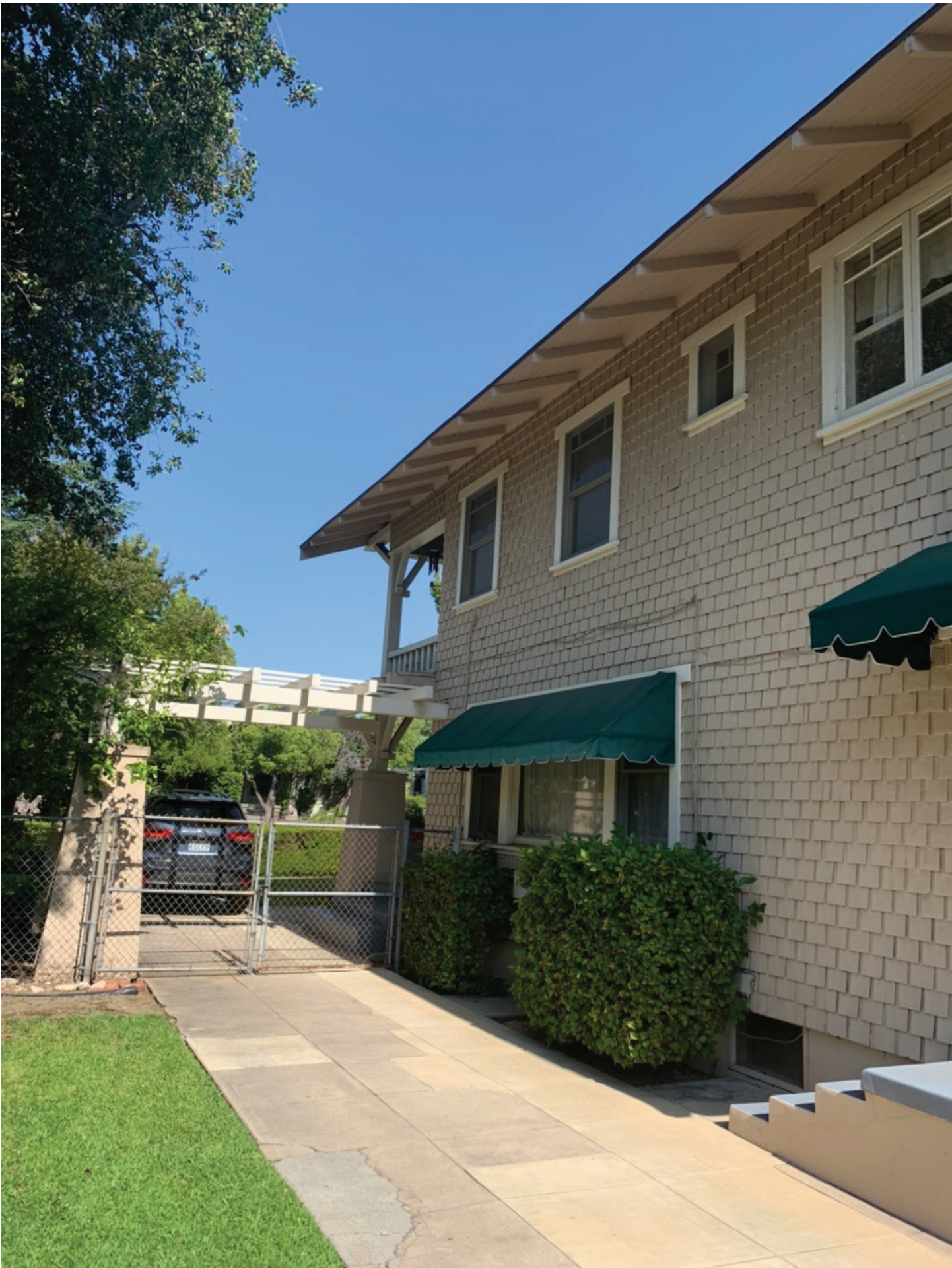
1500 N. LOS ROBLES AVE: SOUTH SIDE ELEVATION ALONG DRIVEWAY, LOOKING WEST
