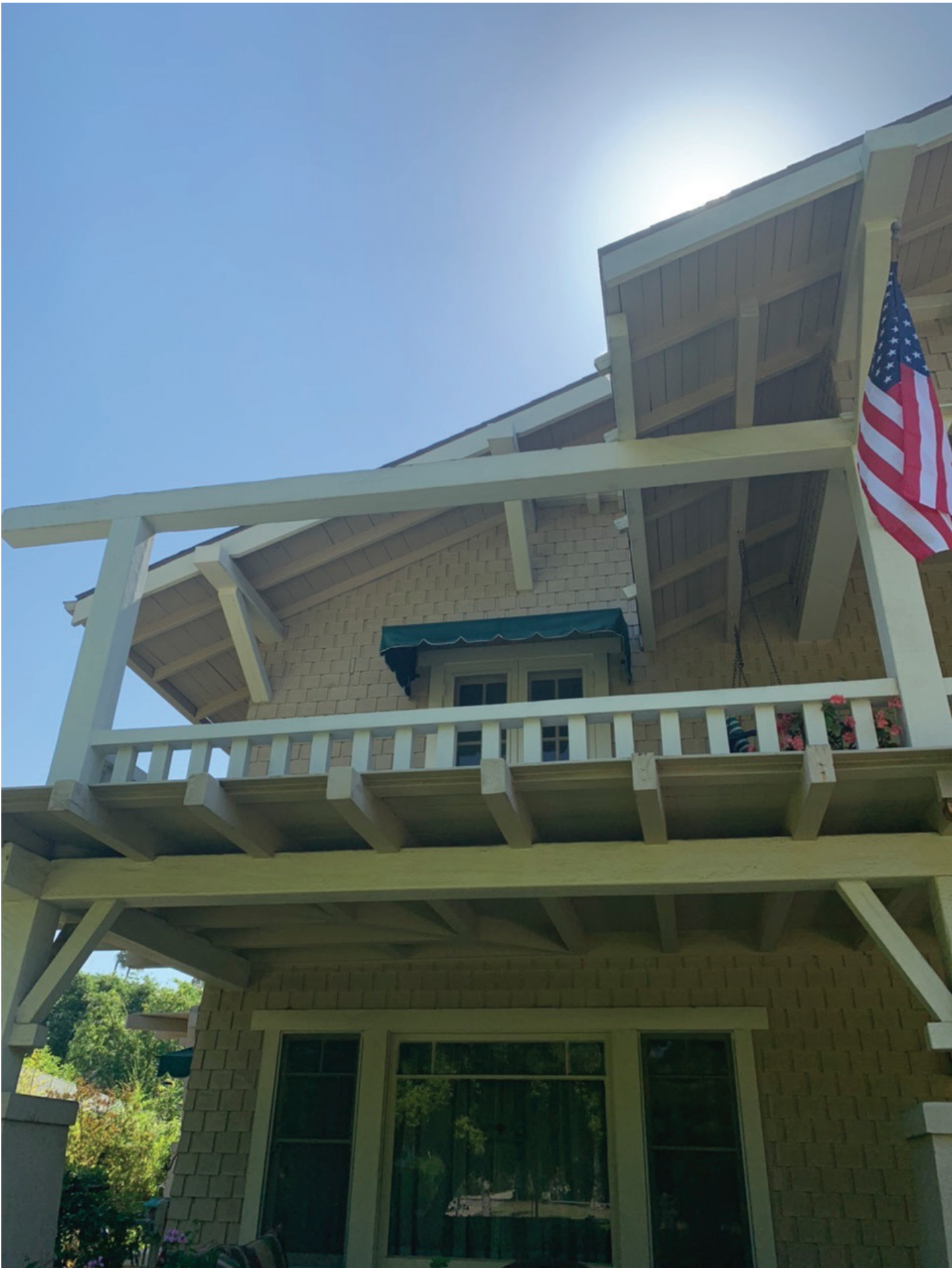
1500 N. LOS ROBLES AVE: UPPER BALCONY, NORTHWEST CORNER
