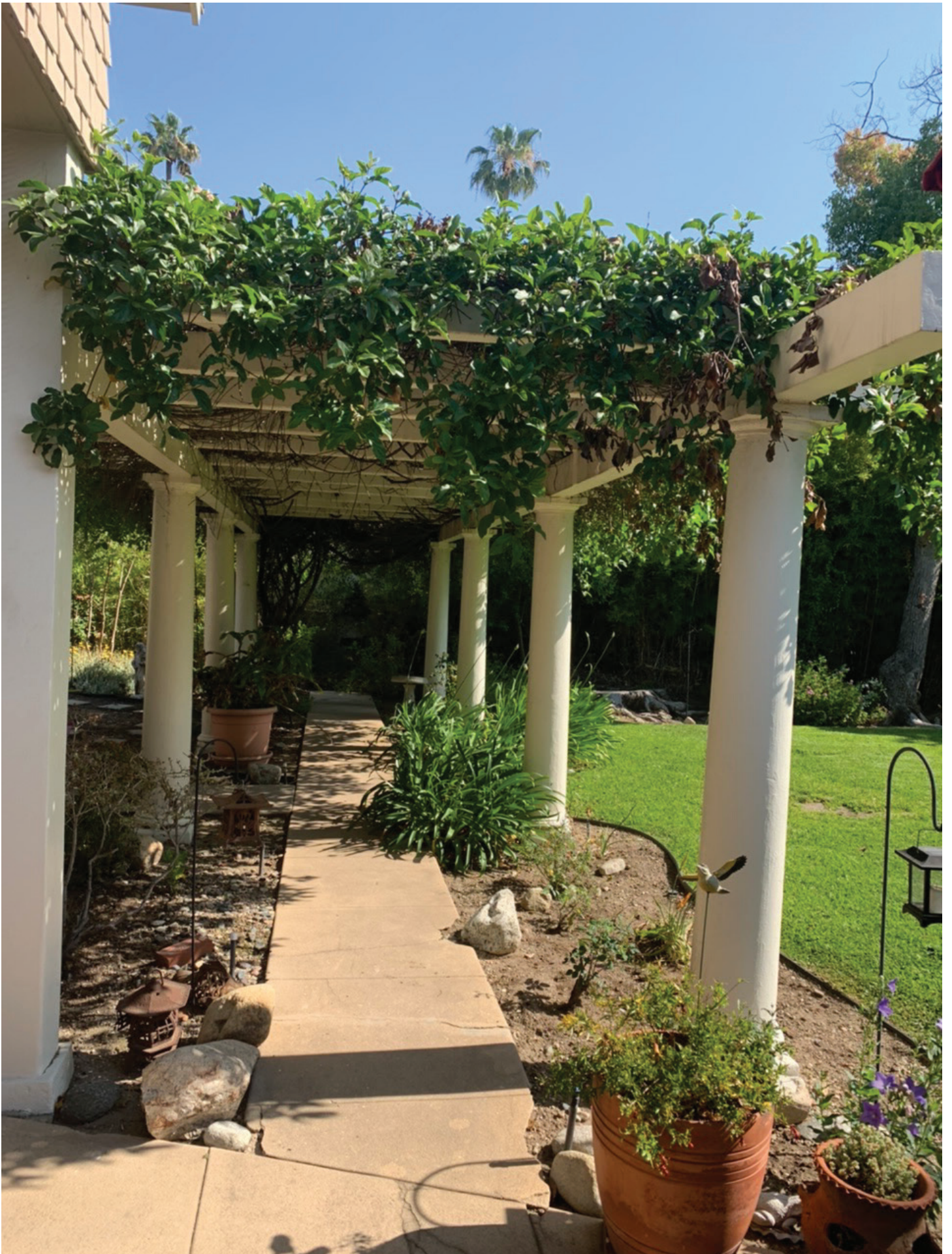
1500 N. LOS ROBLES AVE: REAR YARD PERGOLA LOOKING NORTH
