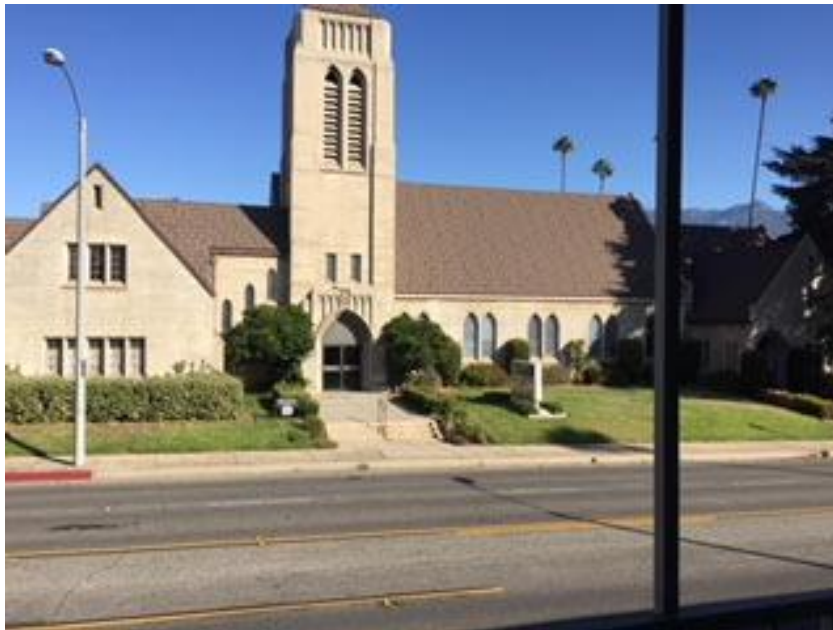
View of the north adjoining property.
