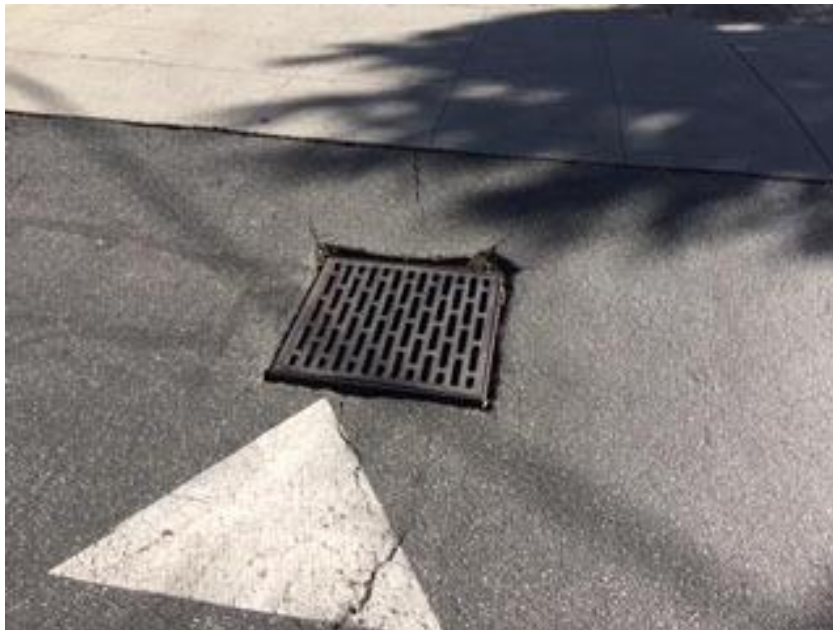
View of a storm drain in the parking area.
