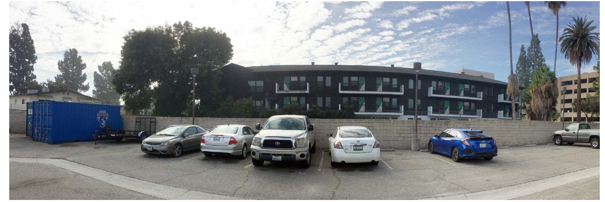
3 EXISTING SITE CONDITIONS
