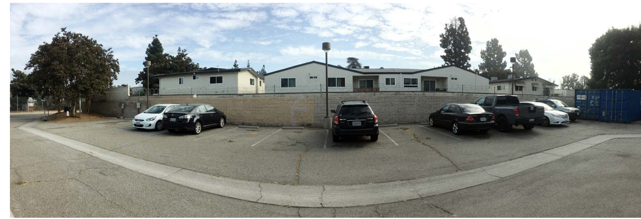
5 EXISTING SITE CONDITIONS
