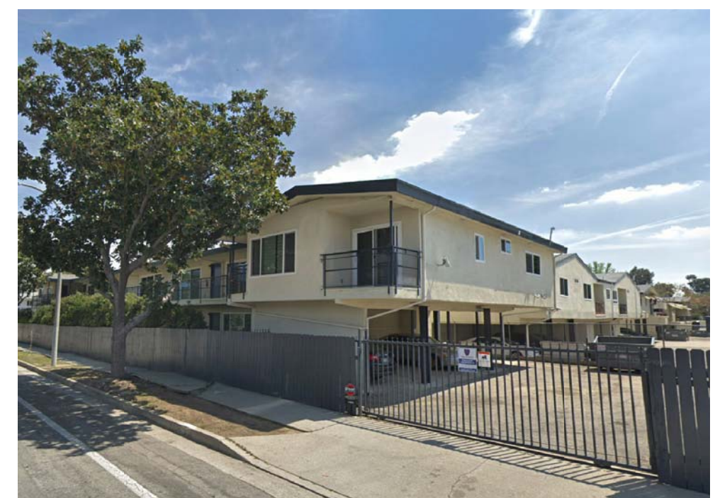
11 303 N OAKLAND AVE - STONECREST
