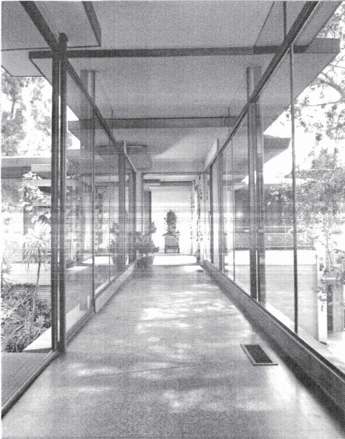
Figure 10. Lyon House, interior view of gallery on glass bridge, view facing south. Photograph by Julius Shulman, 1951. © J. Paul Getty Trust. Getty Research Institute, Los Angeles [2004.R.10(Job 958)].
