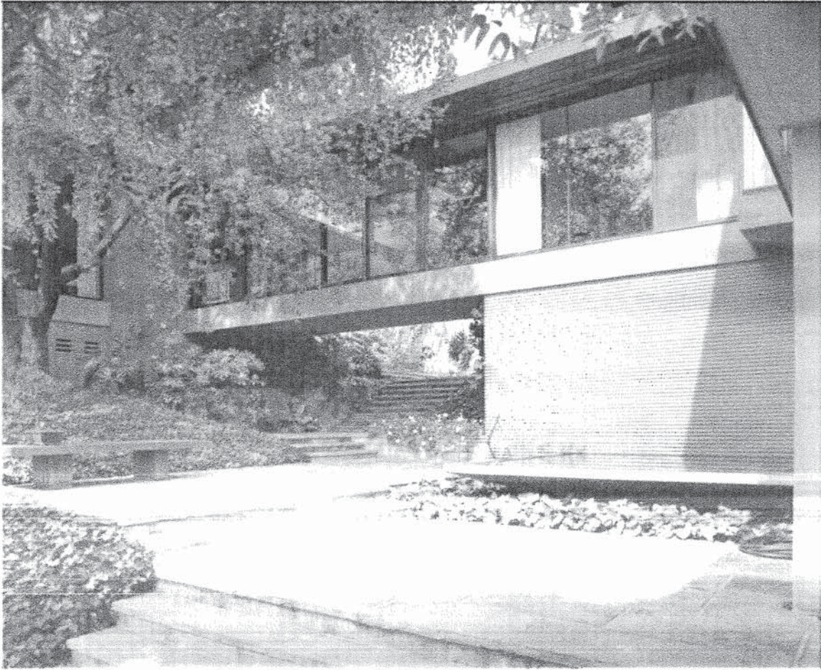
Figure 8. Lyon House, west (primary) façade and glass bridge, view facing northeast. Photograph by Julius Shulman, 1951. © J. Paul Getty Trust. Getty Research Institute, Los Angeles [2004.R.10(Job 958)].
