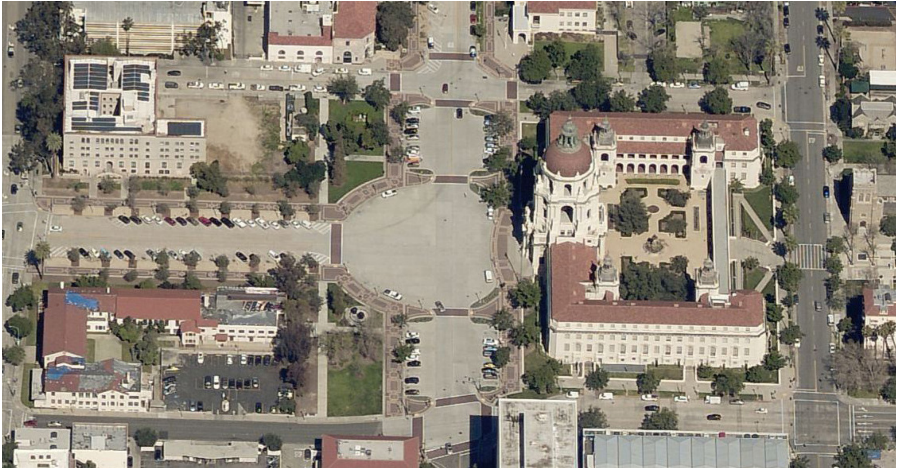
AERIAL VIEW OF EXISTING SITE CONDITIONS
