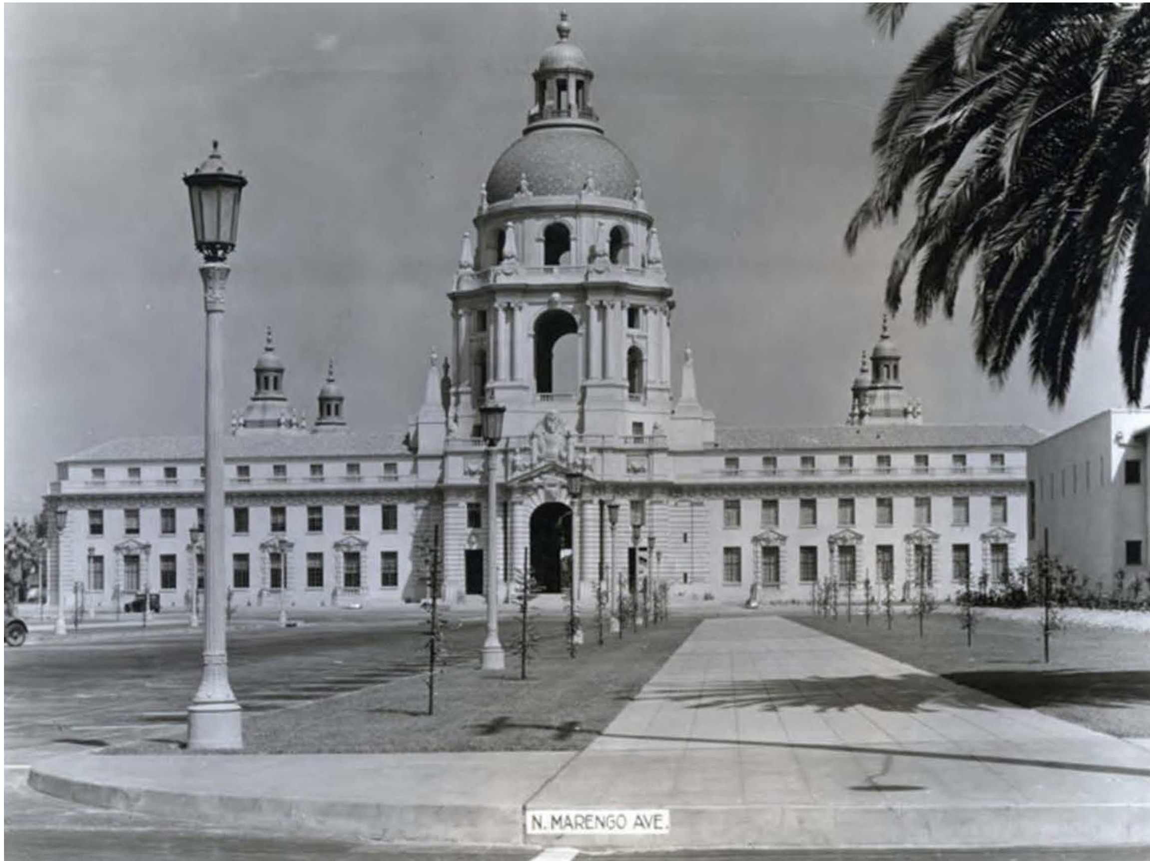
PASADENA CITY HALL, BAKEWELL & BROWN ARCHITECTS, 1927
