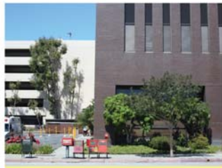
Fair Oaks Avenue - West
