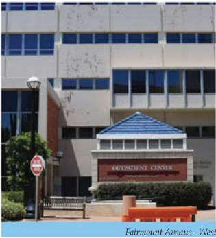
Fairmount Avenue - West
