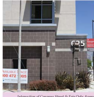
Intersection of Congress Street & Fair Oaks Avenue
