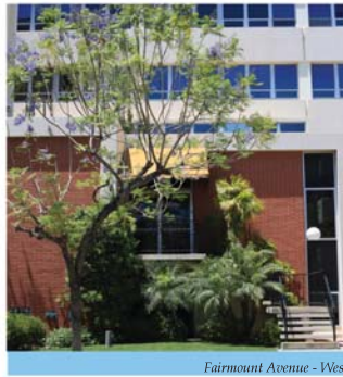
Fairmount Avenue - West
