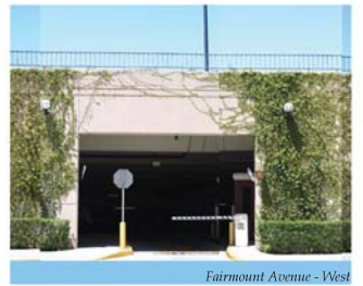
Fairmount Avenue - West
