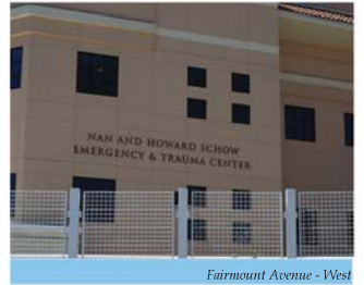
Fairmount Avenue - West
