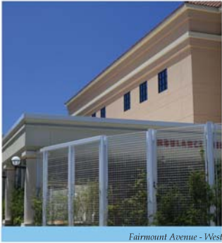
Fairmount Avenue - West
