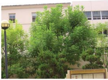
Valentine Building - North Elevation
