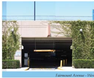
Fairmount Avenue - West
