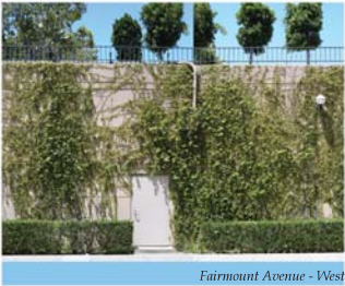
Fairmount Avenue - West
