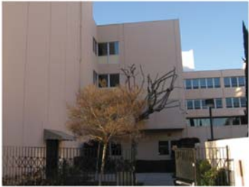
Valentine Building - South Elevation
