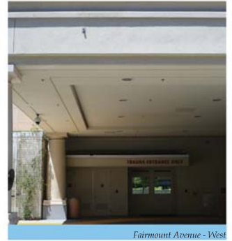
Fairmount Avenue - West
