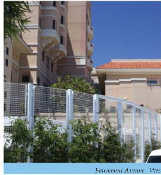
Fairmount Avenue - West
