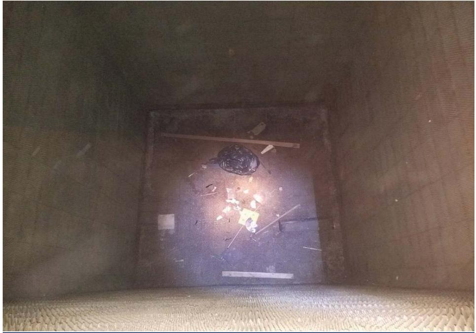
**Photograph 3:** View of the inside of the anechoic tank. Water or other indications of liquid were not observed.
