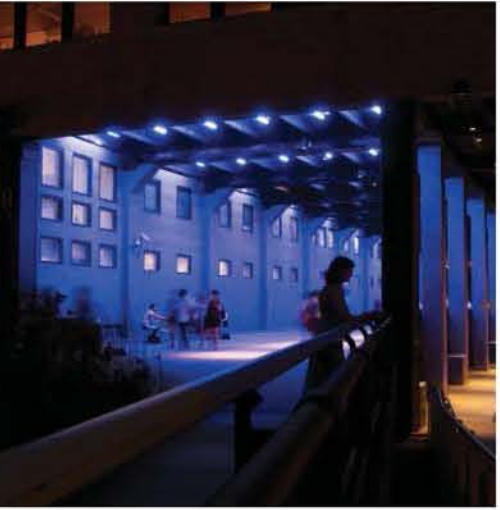
Tunnels, vehicular entry ramps and areas under Buildings (image: High Line, New York City, NY, USA)
