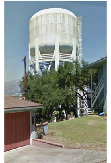
D / WATER TOWER
