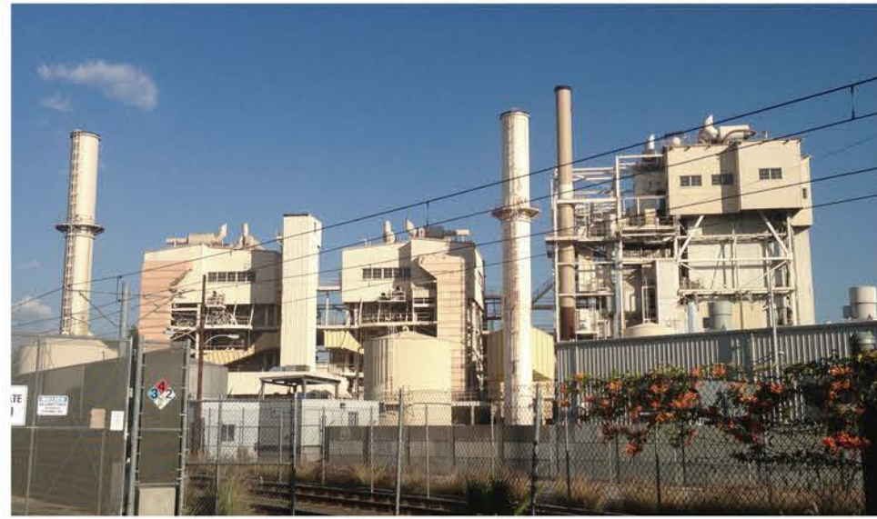
B / BROADWAY POWER PLANT
