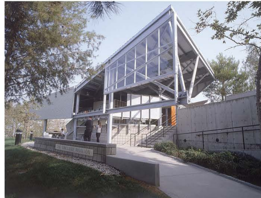
EXTERIOR VIEW / SINCLAIRE PAVILION
