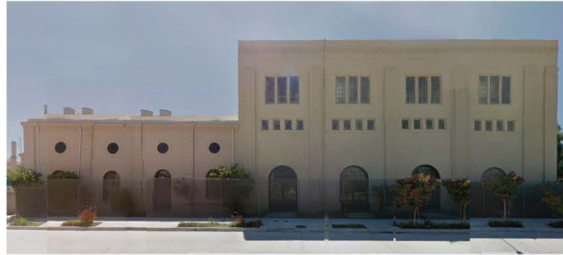
C / GLENARM POWER PLANT
