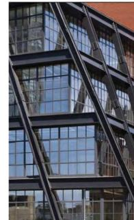
The south façade of the Dayton block apartments will be primarily glass and metal and will filter the light through metal panels with a custom decorative pattern, an interpretation of the play of light and shadow from both plants and structure in 19th century glasshouses. This will allow some shelter on the southern exposure while maintaining views of the park.
